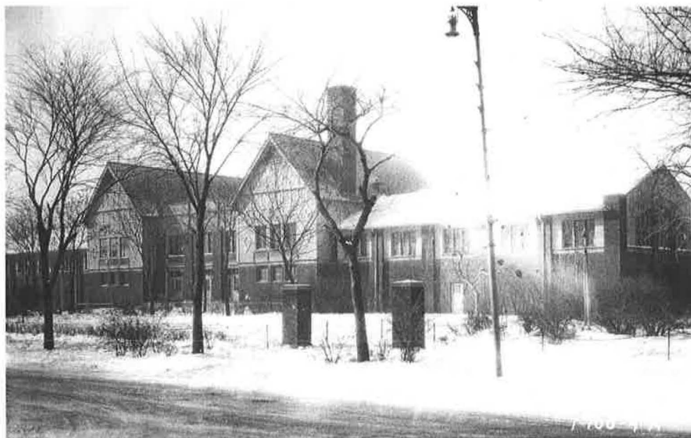
Figure 4: Historic photograph of Kosciuszko Park field house East façade looking Southwest
