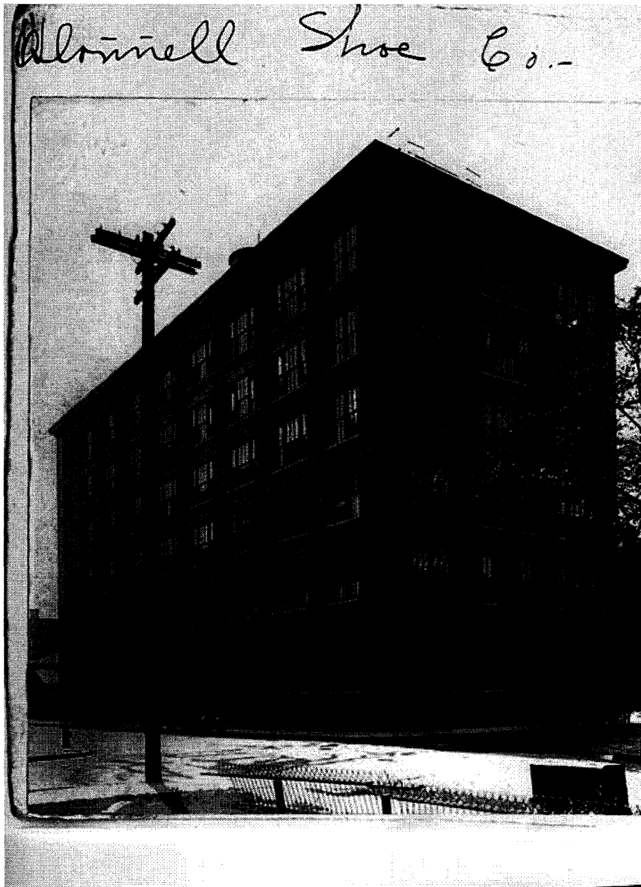
O'Donnell Shoe Company Building, looking southwest ca. 1915-19. (Minnesota Historical Society)
