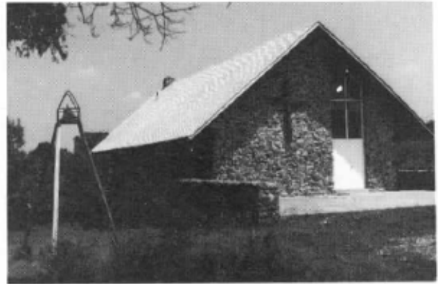
Figure 6: St. Sylvester Church completed in 1954 of local stone and clear span wood truss roof (right); Bristol Primary School completed in 1956 of glass and steel (bottom). Source: Architecture and Urbanism . Special supplemental issue devoted to Gyo Obata/HOK 1954-1990. December 1990, extra edition, page 226.
