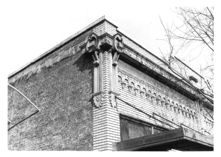
6 of 7 Close-up view of galvanized sheet metal cornice assembly, SW corner.
