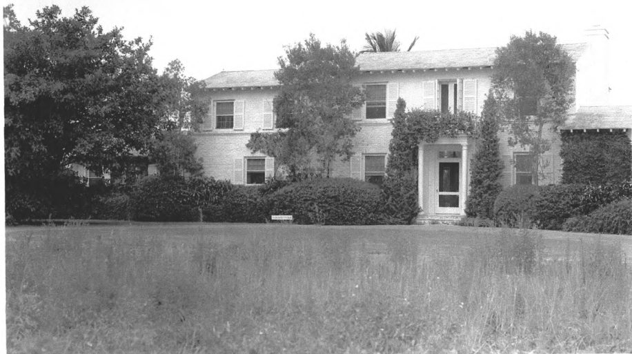
DICKENSON HOUSE (front)
