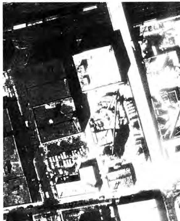
Figure 22: 1963 photo, showing concrete mixing plant to the south of the building (City of Des Moines)
