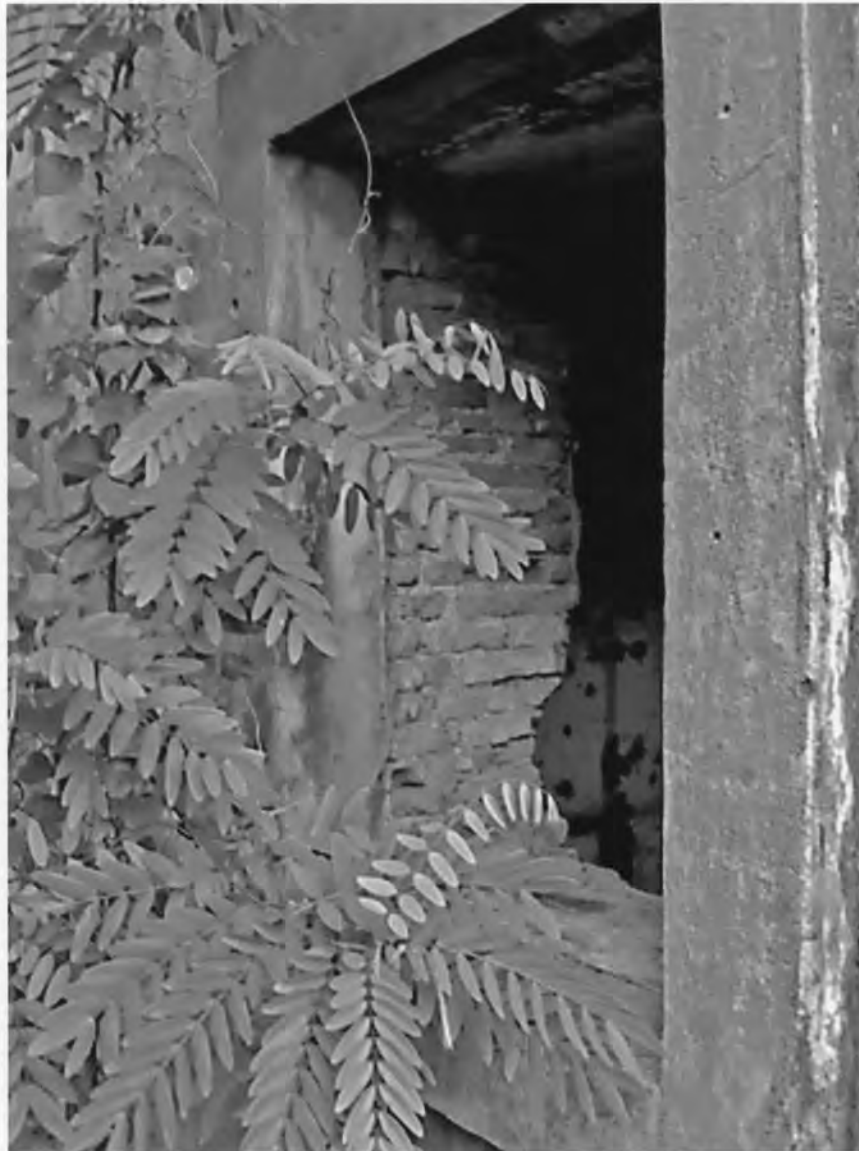
PHOTO #98. Water reservoir, valve house, Acueducto de San Juan Historic District.
