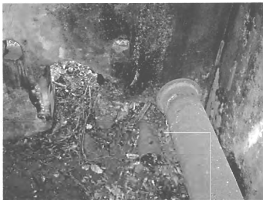
PHOTO #100. Water reservoir, valve house, Acueducto de San Juan Historic District.
