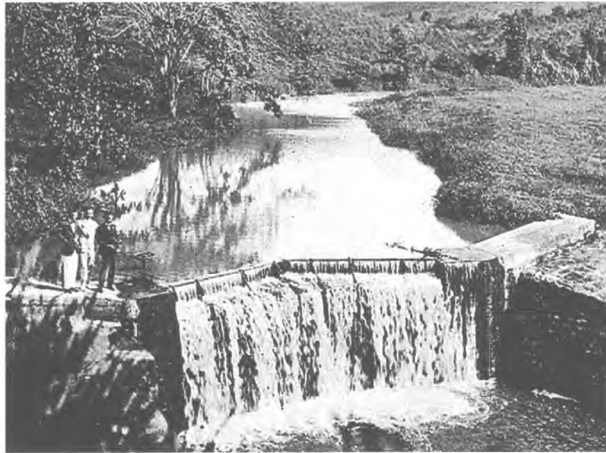
PHOTO #59. Weir, general view, 1916, Acueducto de San Juan Historic District.
