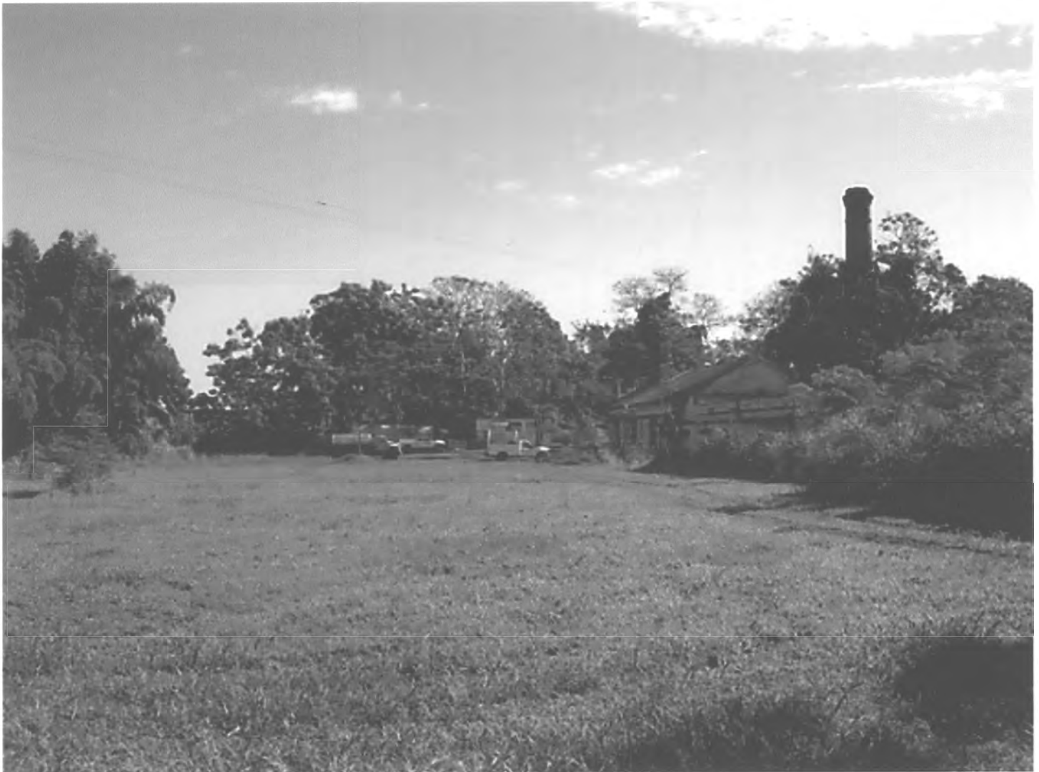
PHOTO #82. Settling basins area, Acueducto de San Juan Historic District.
