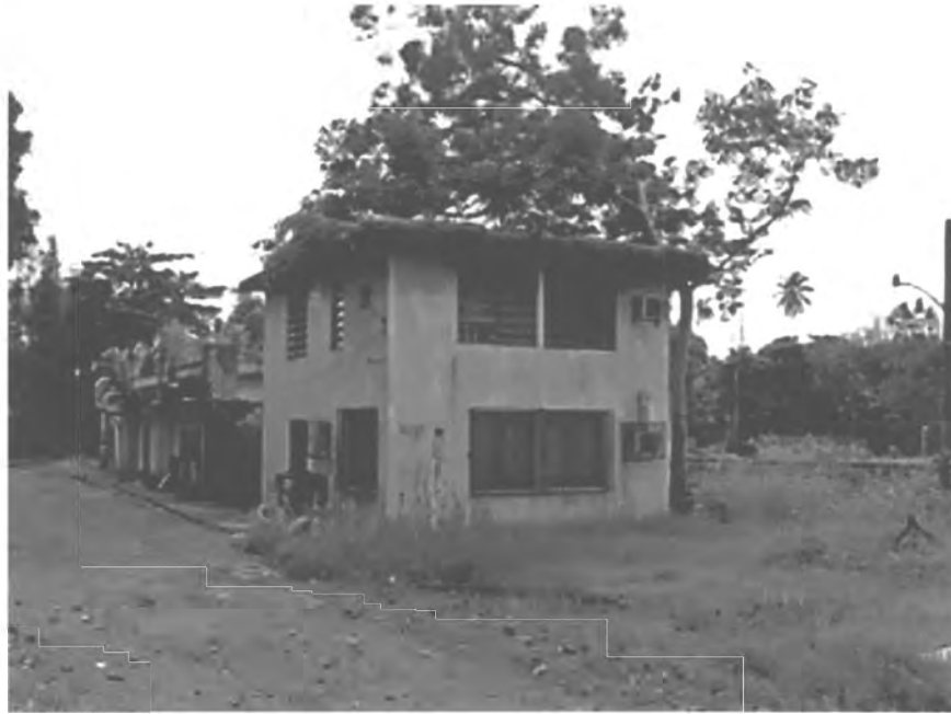
PHOTO #73. Engineer's Offices I, exterior, Acueducto de San Juan Historic District.
