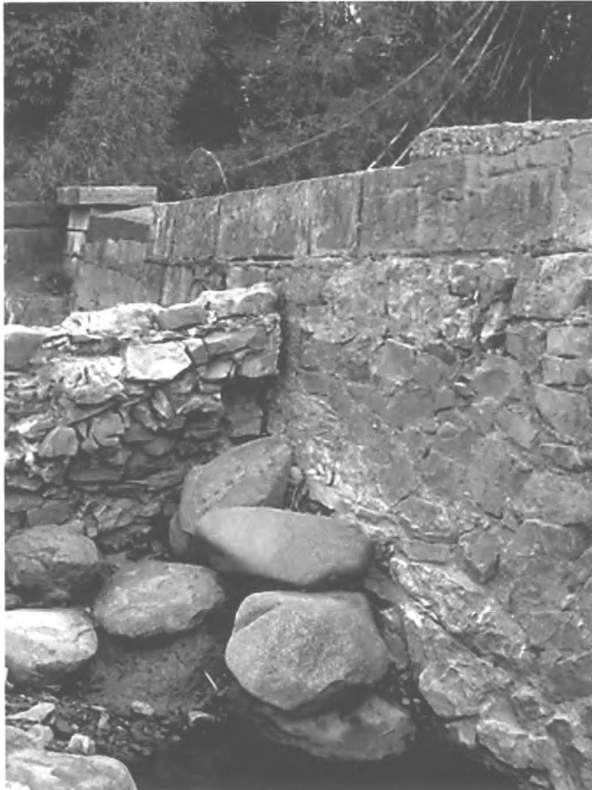
PHOTO #54. Weir, structural detail, Acueducto de San Juan Historic District.
