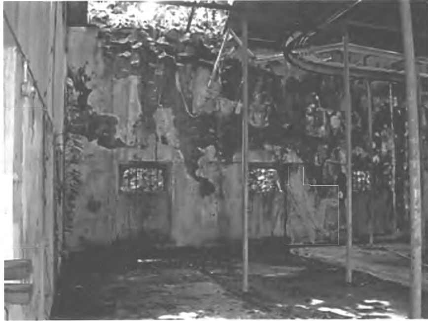
PHOTO #24. Pumping Station, interior, Acueducto de San Juan Historic District.
