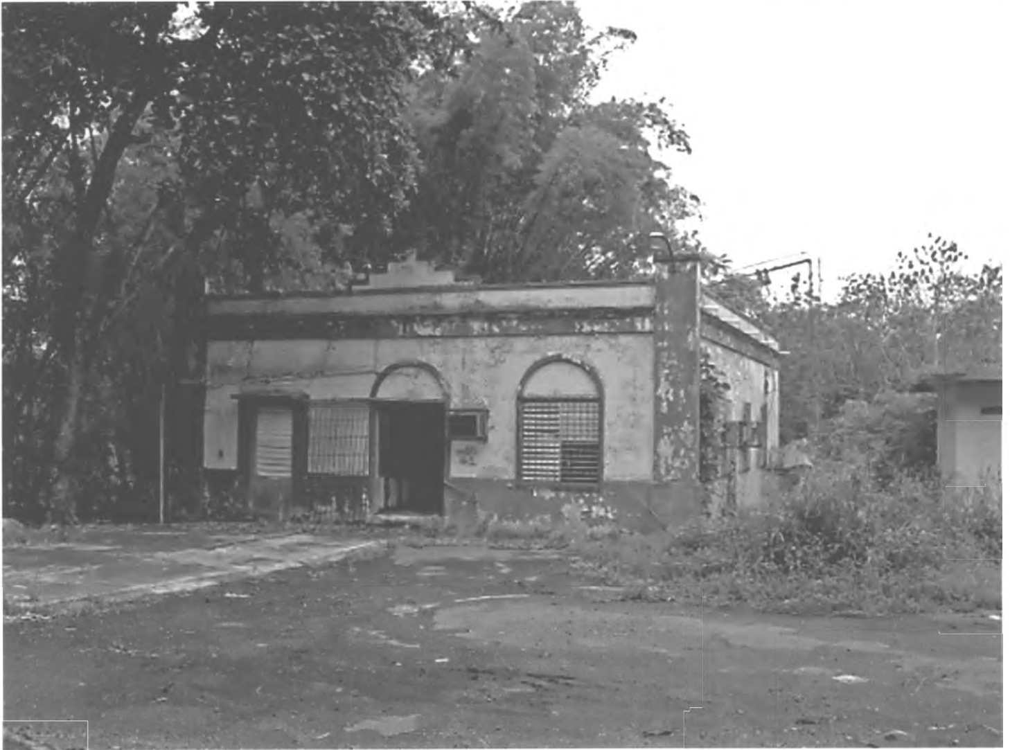
PHOTO #42. Valve and Mixing House, exterior, Acueducto de San Juan Historic District.
