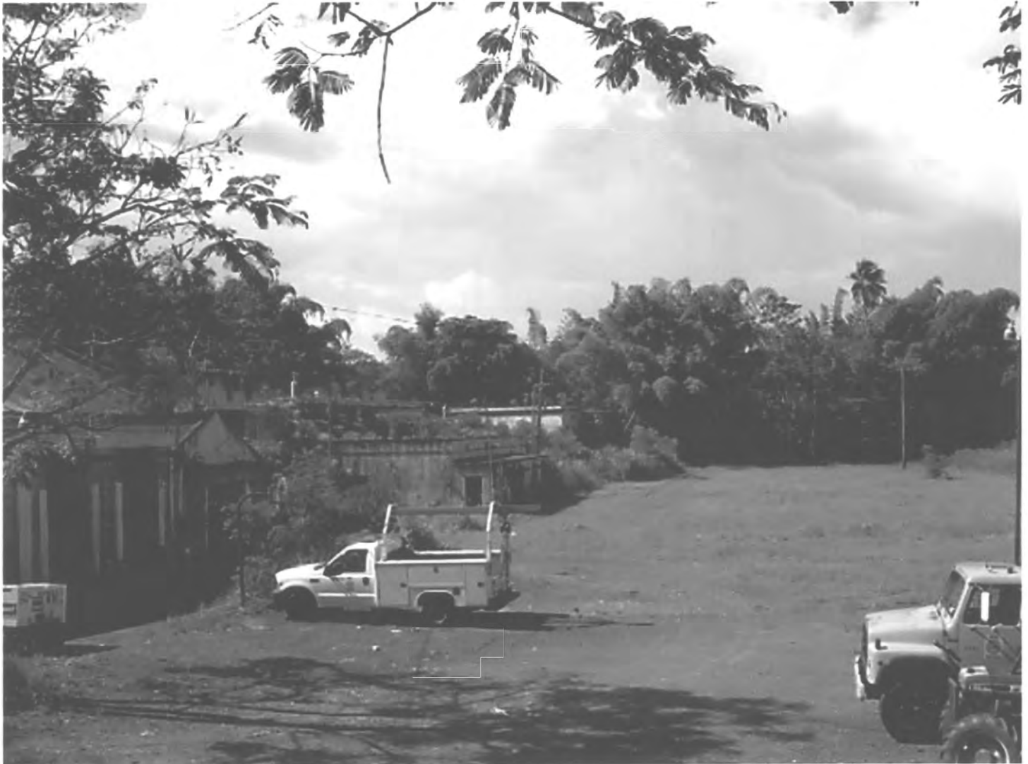
PHOTO #83. Settling basins area, Acueducto de San Juan Historic District.
