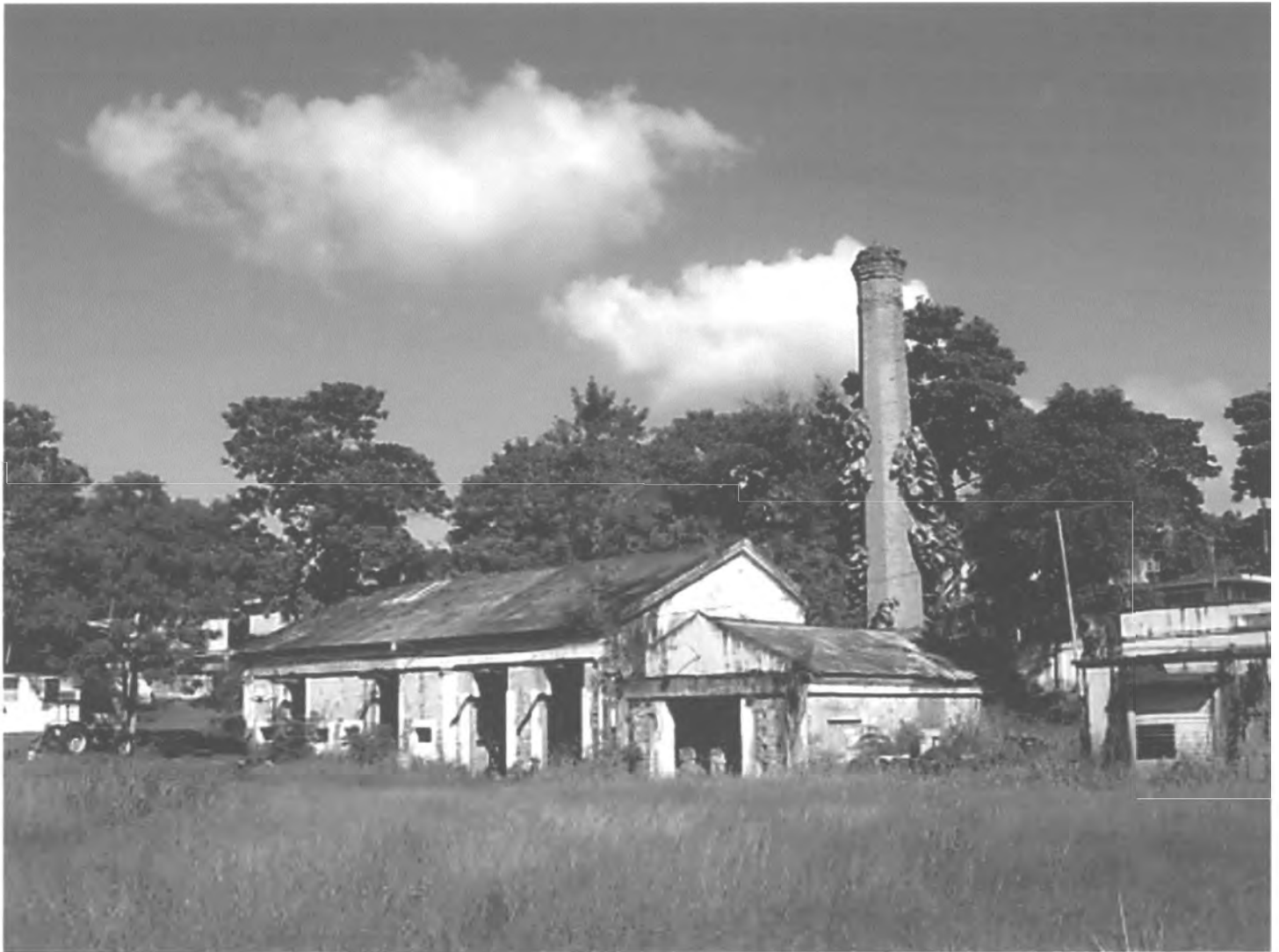
PHOTO 23. Pumping Station, exterior, Acueducto de San Juan Historic District.
