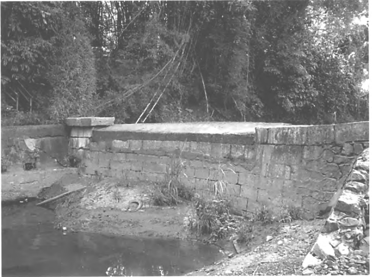
PHOTO #51. Weir, Acueducto de San Juan Historic District.
