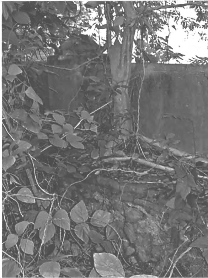
PHOTO #101. Water reservoir, construction materials, Acueducto de San Juan Historic District.
