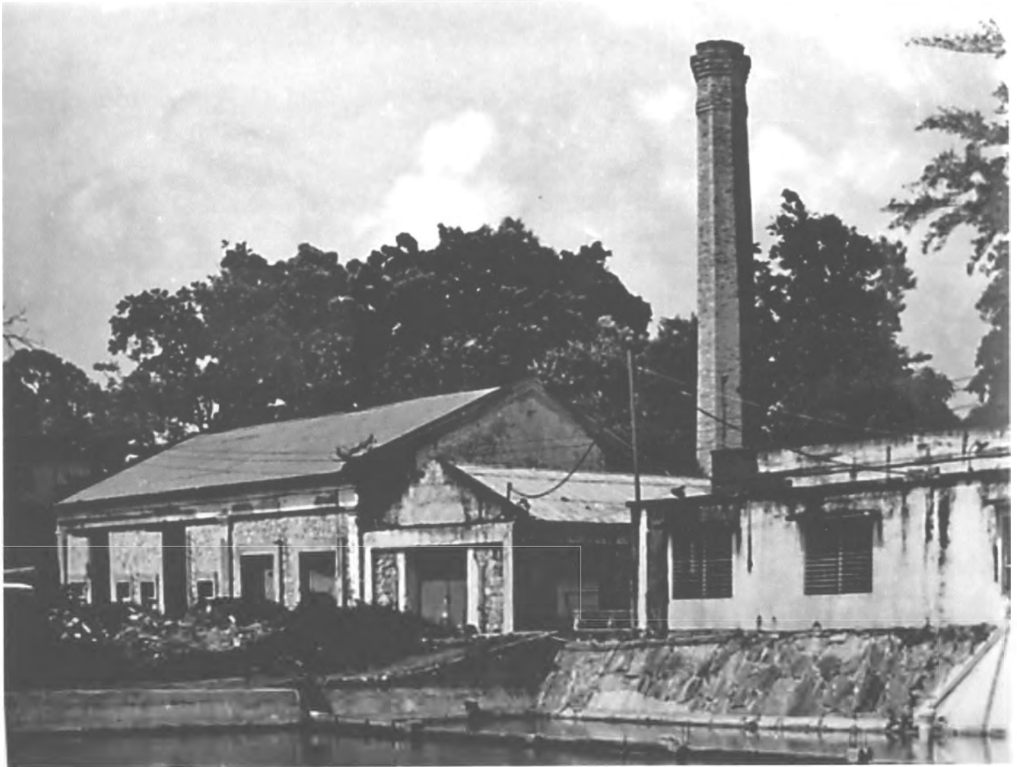
PHOTO #22. Settling Basin and Pumping Station, 1977, Acueducto de San Juan Historic District.
