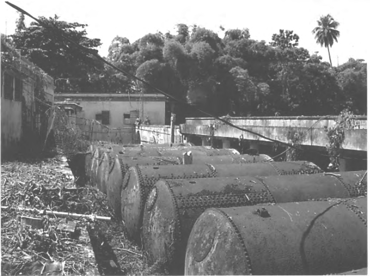
PHOTO #35. Chemical and Mechanical Filter 77 House, filters, Acueducto de San Juan Historic District.
