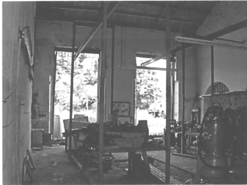
PHOTO #26. Pumping Station, boiler house, Acueducto de San Juan Historic District.
