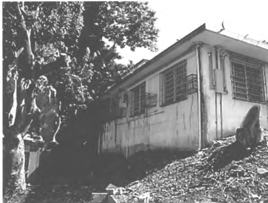
PHOTO #76. Engineer's Offices II, exterior, Acueducto de San Juan Historic District.
