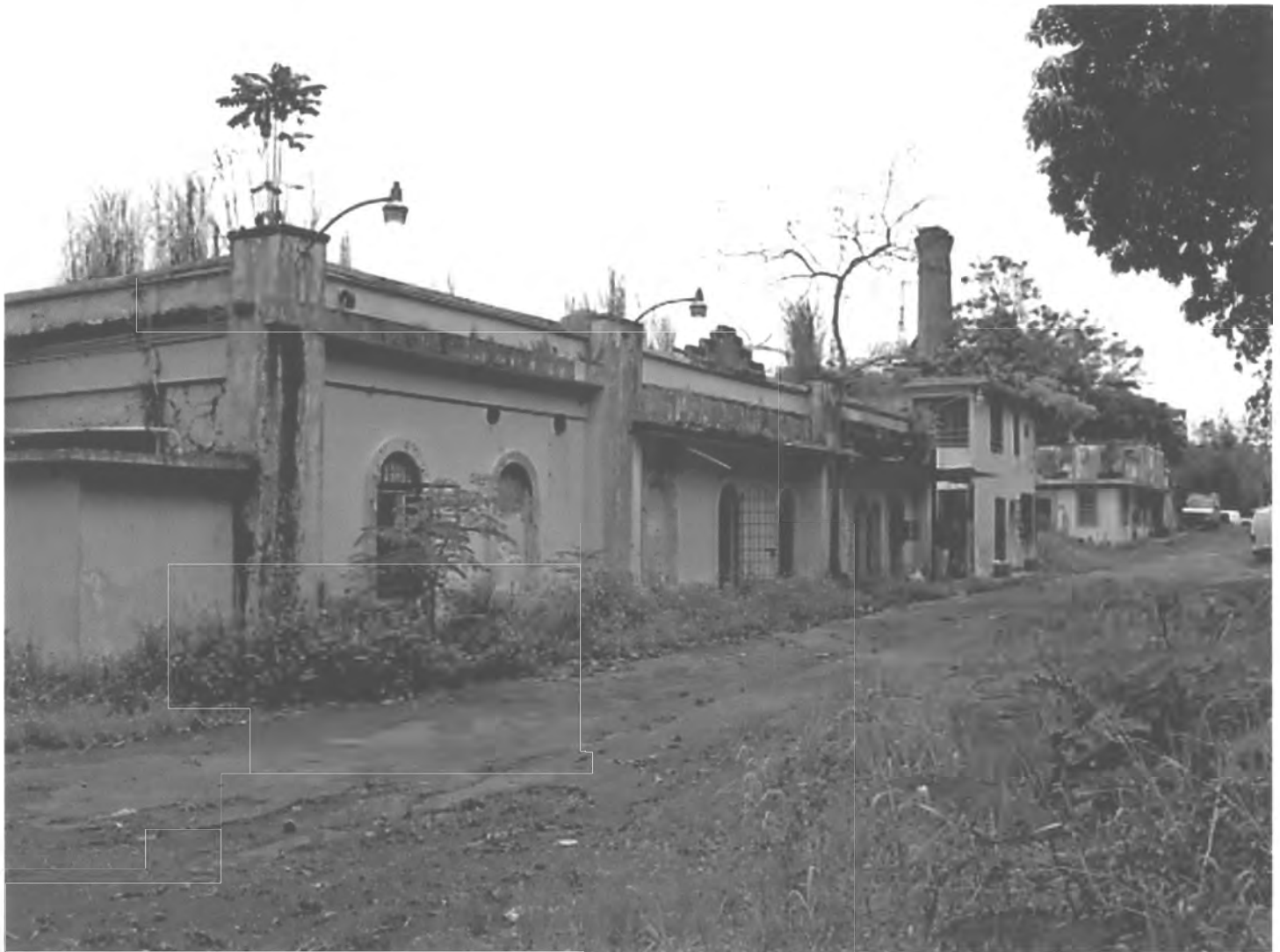
PHOTO #66. Engineers and Caretaker's Residence, exterior, Acueducto de San Juan Historic District.
