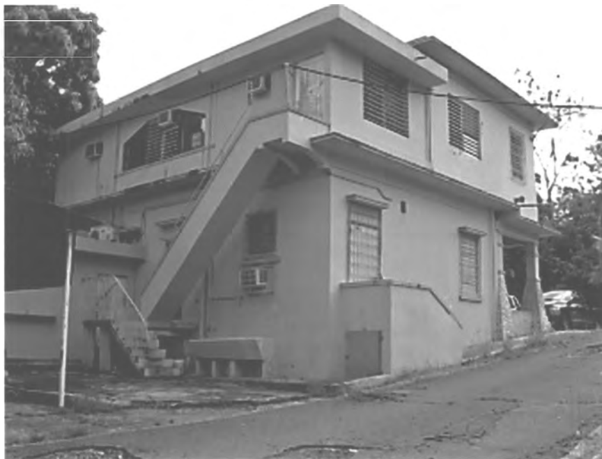
PHOTO #16. Director's residence, exterior, Acueducto de San Juan Historic District.
