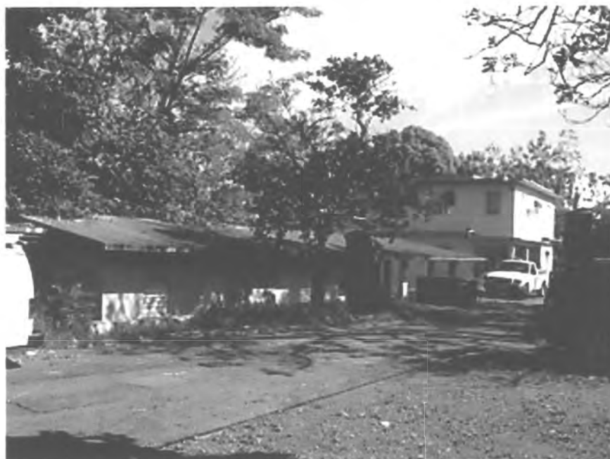
PHOTO #78. Employees' lounge, exterior, Acueducto de San Juan Historic District.
