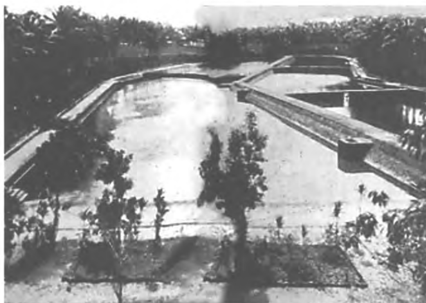
PHOTO #87. Settling basins 1923, Acueducto de San Juan Historic District.
