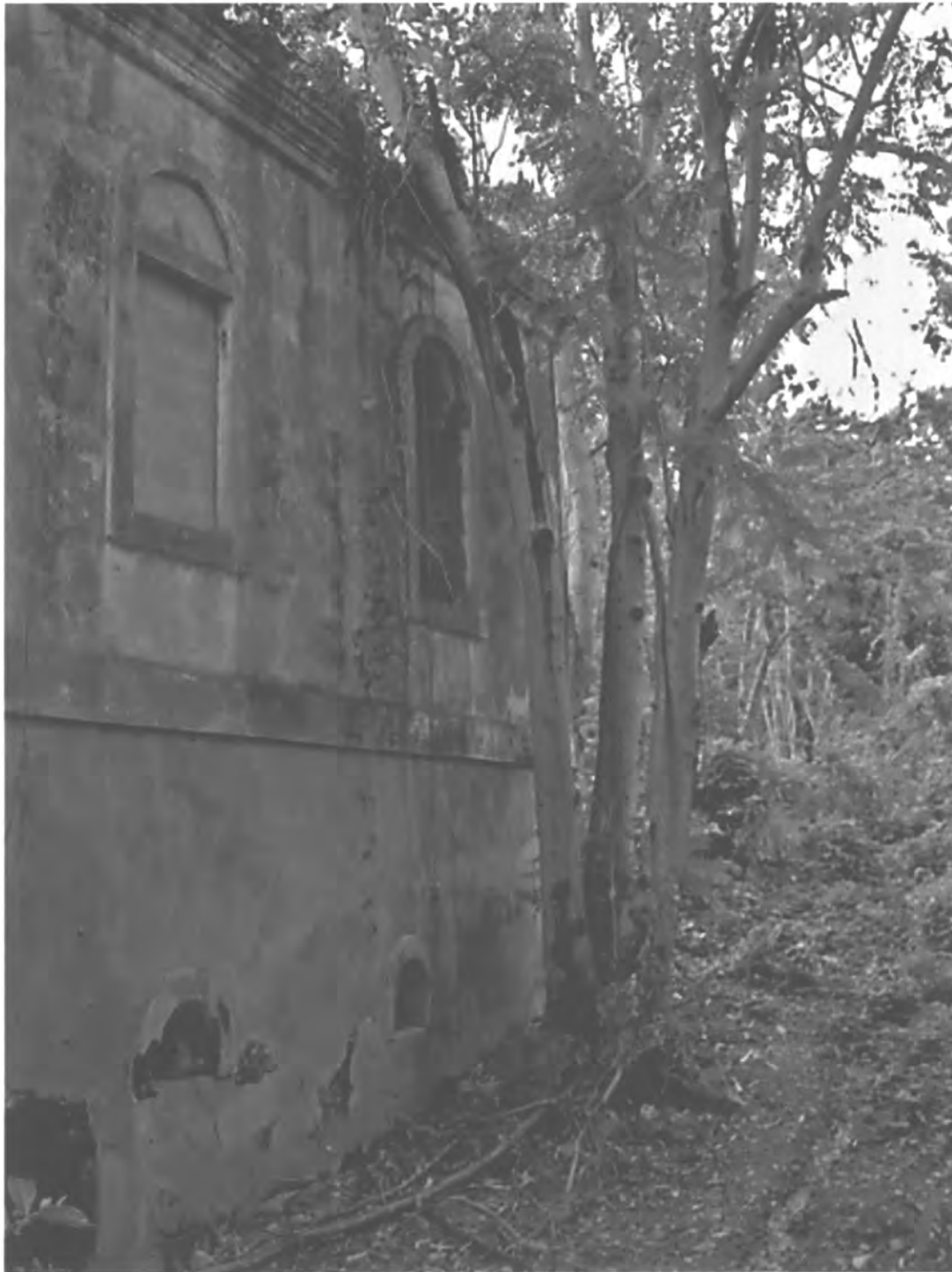
PHOTO #95 , Water reservoir, valve house, Acueducto de San Juan Historic District.
