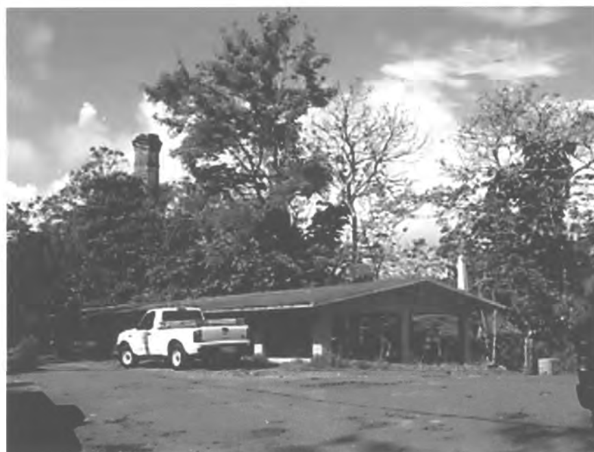
PHOTO #79. Employees' lounge, exterior, Acueducto de San Juan Historic District.
