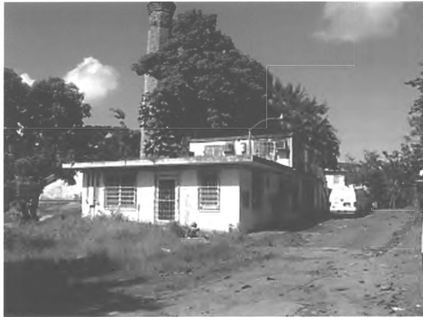
PHOTO #75. Engineer's Offices II, exterior, Acueducto de San Juan Historic District.
