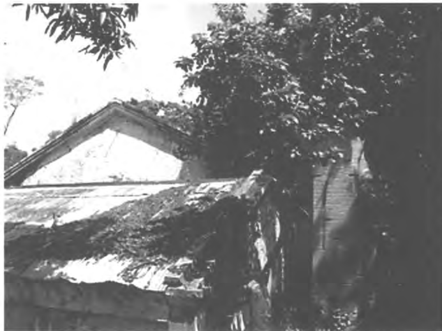
PHOTO #28. Pumping Station, Chimney, Acueducto de San Juan Historic District.
