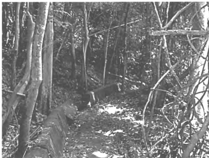
PHOTO #86. Settling basins, Acueducto de San Juan Historic District.
