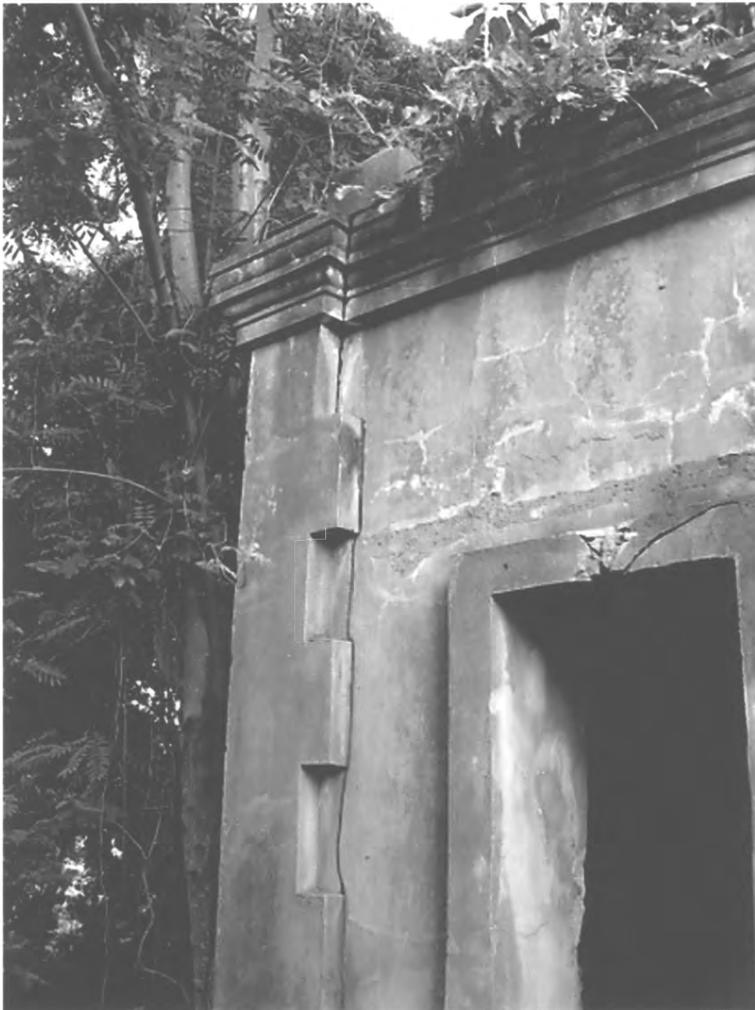
PHOTO #97. Water reservoir, valve house, Acueducto de San Juan Historic District.
