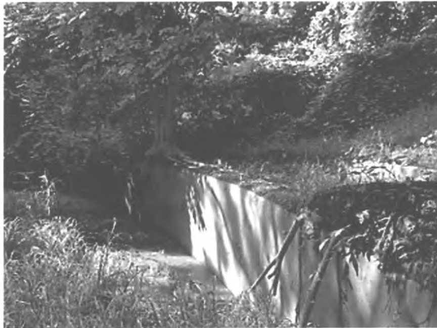
PHOTO #84. Settling basins, Acueducto de San Juan Historic District.
