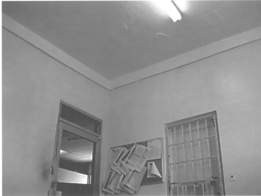
PHOTO #19. Director's residence, interior, Acueducto de San Juan Historic District.
