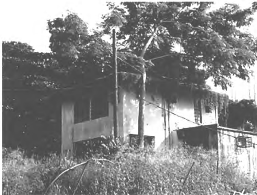
PHOTO #74. Engineer's Offices I, exterior, Acueducto de San Juan Historic District.
