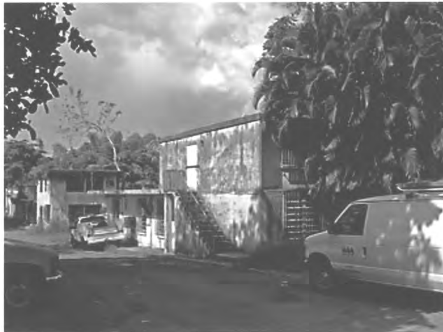
PHOTO #77. Engineer's Offices II, exterior, Acueducto de San Juan Historic District.
