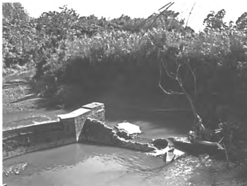
PHOTO #62. Weir, left embankment, Acueducto de San Juan Historic District.
