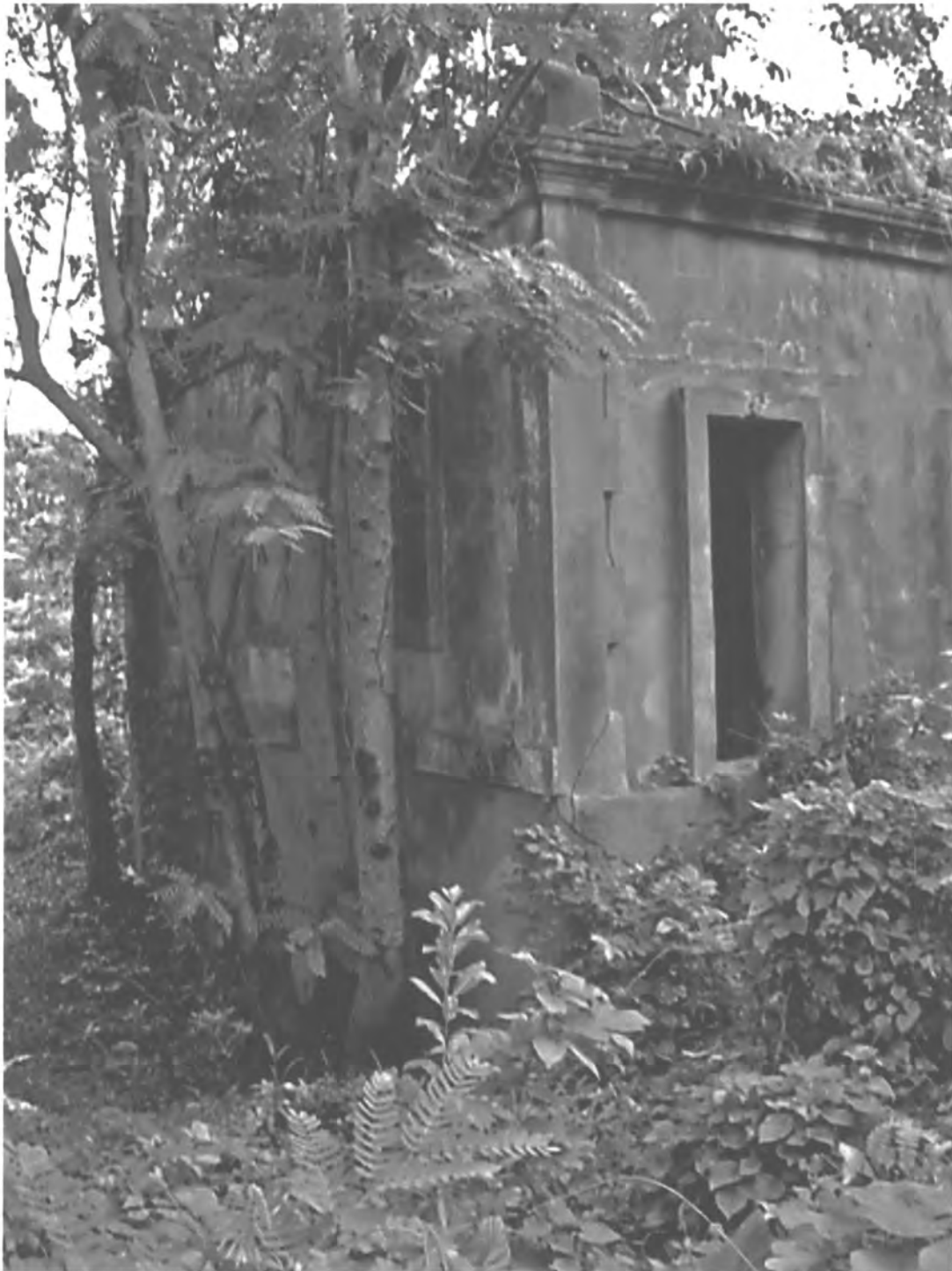
PHOTO #94. Water reservoir, valve house, Acueducto de San Juan Historic District.
