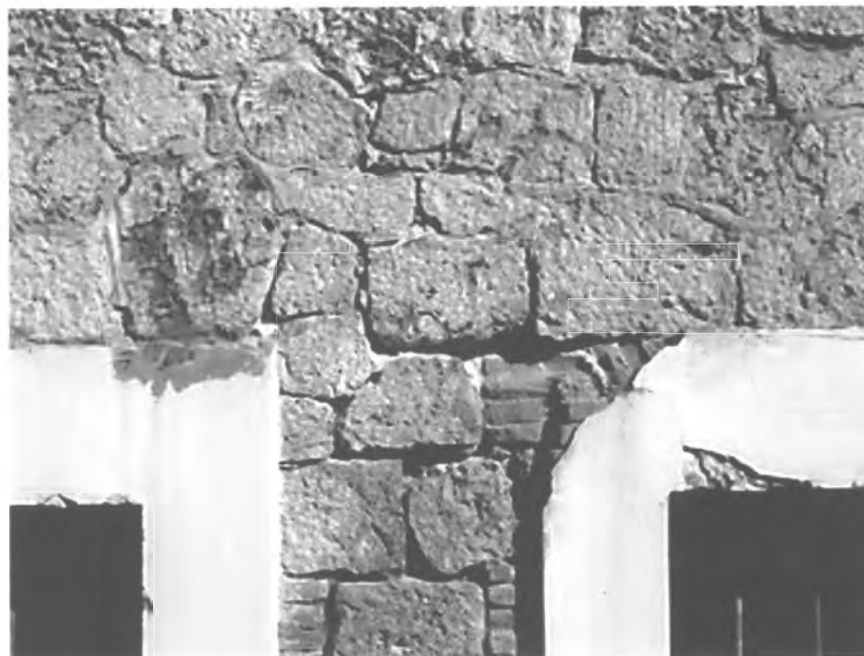
PHOTO #32. Pumping Station, Wall Detail, Acueducto de San Juan Historic District.
