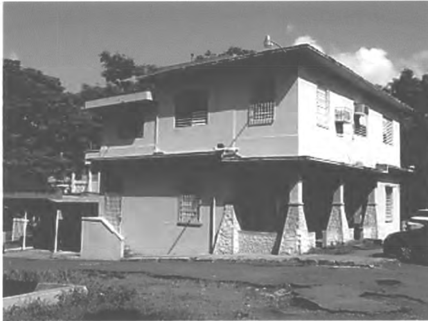
PHOTO #15. Director's residence, exterior, Acueducto de San Juan Historic District.
