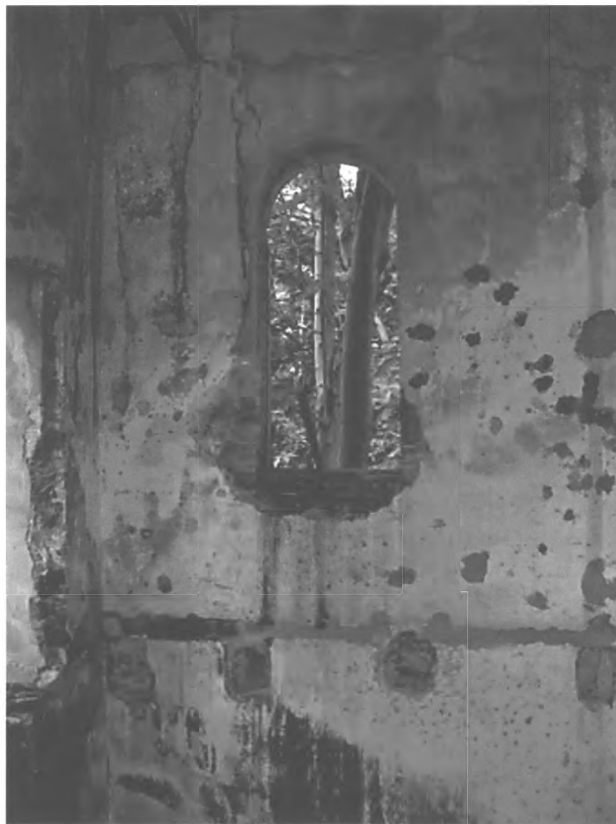
PHOTO #96. Water reservoir, valve house, Acueducto de San Juan Historic District.
