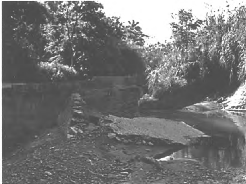
PHOTO #64. Weir, left embankment, Acueducto de San Juan Historic District.
