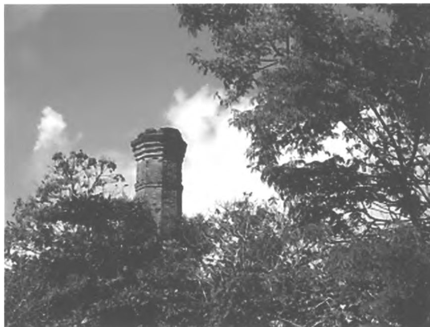
PHOTO #29. Pumping Station, Chimney, Acueducto de San Juan Historic District.
