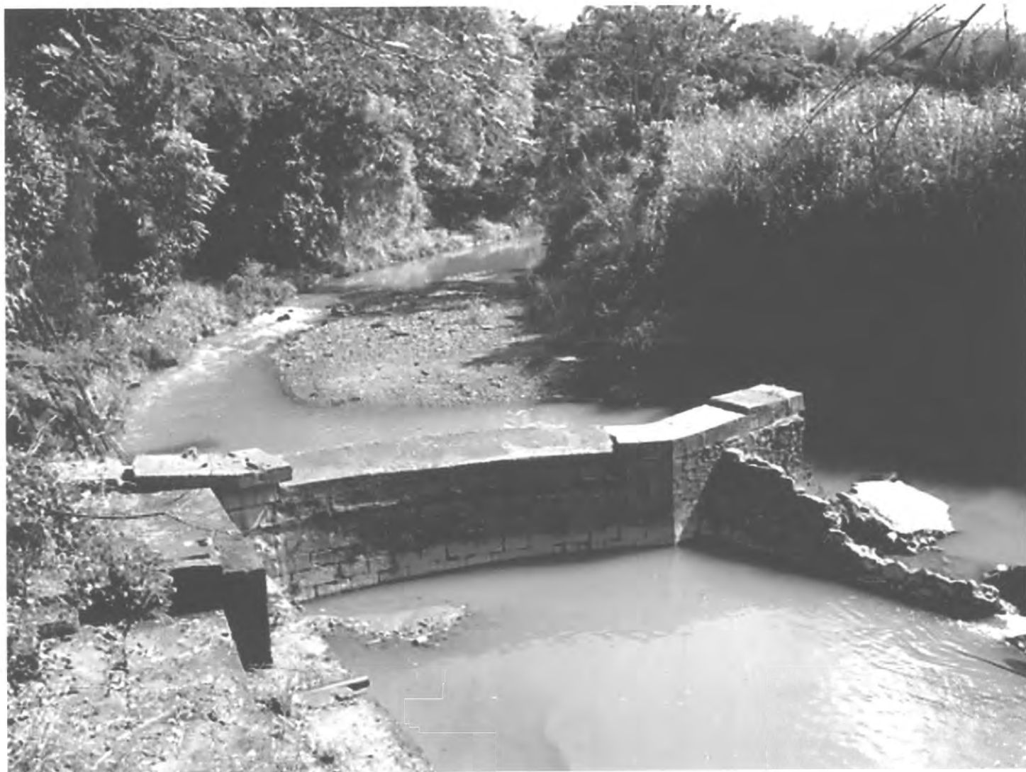
PHOTO #50. Weir, Acueducto de San Juan Historic District.
