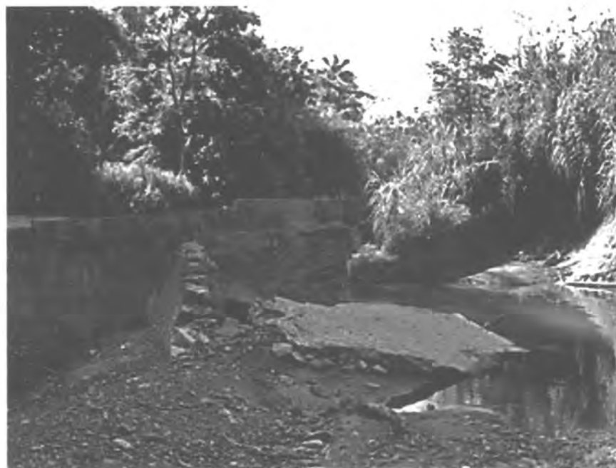
PHOTO #63. Weir, left embankment, Acueducto de San Juan Historic District.
