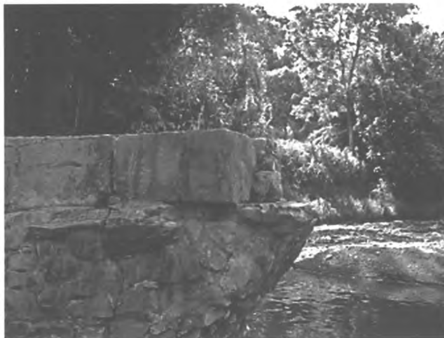
PHOTO #65. Weir, left embankment, Acueducto de San Juan Historic District.
