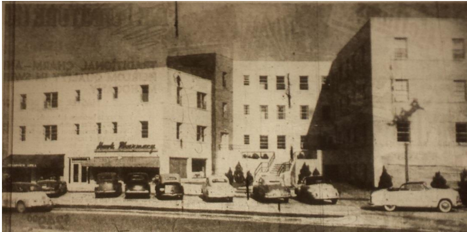
Figure 2 – Historic View of Building at opening, The Wichita Eagle 12 March 1950, page 15.
