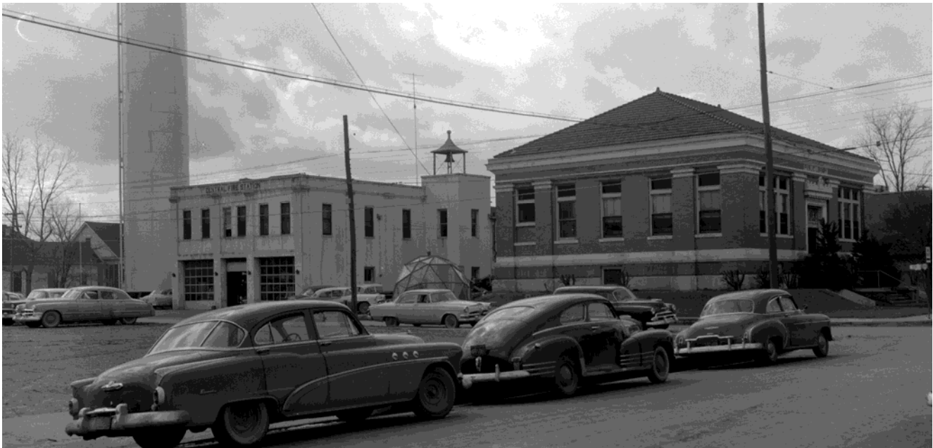
Figure 8: View of previous Central Fire Station on site, Alexandria Public Library, Lee Street Water Standpipe along 5 th St. at Washington St., 1957. Image courtesy of the Joe Dellmon Photograph Collection, Cammie G. Henry Research Center, Watson Library, Northwestern State University.
