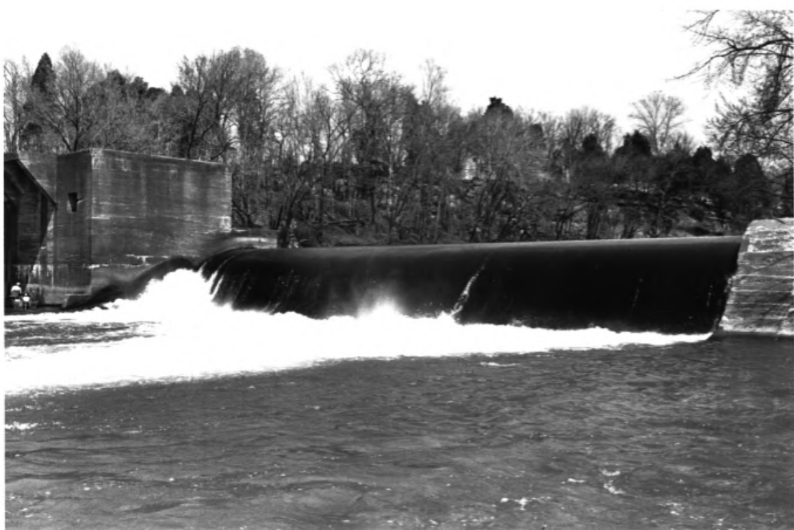
Lillard's Mill Hydroelectric Station Milltown vicinity, Marshall County, TN
