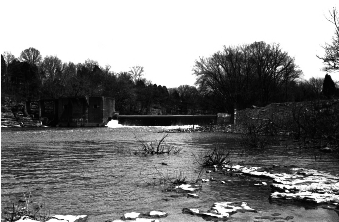
Lillard & Mill Hydroelectric Station Milltown vicinity, Marshall County, TN
