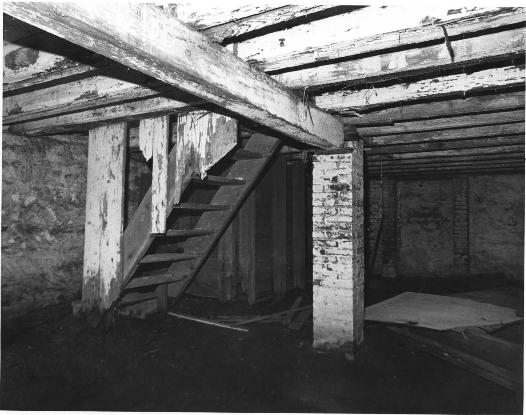
MAURICE RIVER LIGHTHOUSE, CUMBERLAND COUNTY, NJ # 19 of 34
