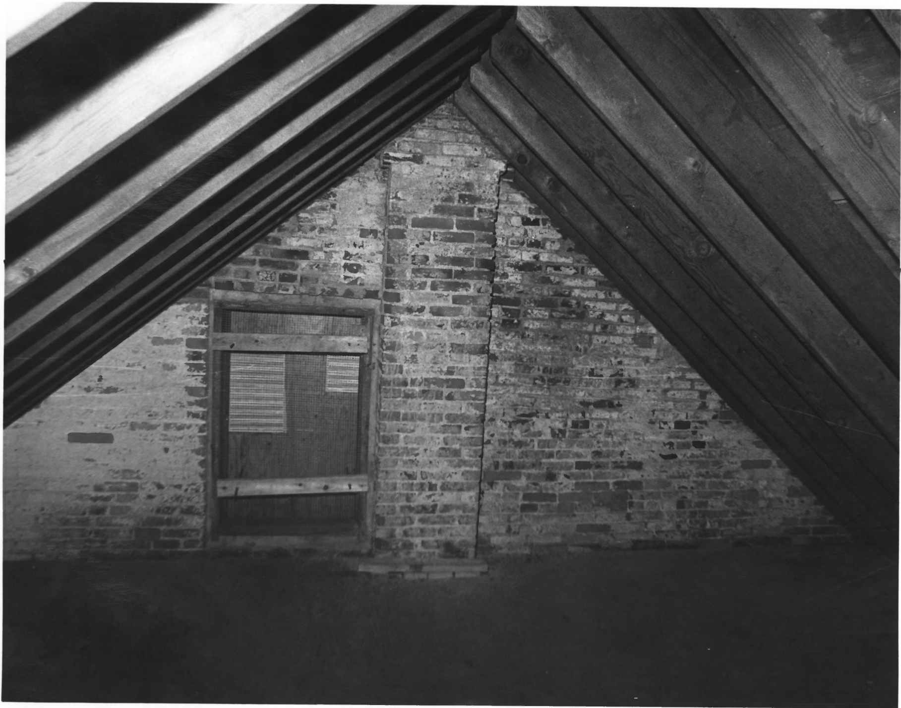
MAURICE RIVER LIGHTHOUSE, CUMBERLAND COUNTY, NJ #25 of 34
