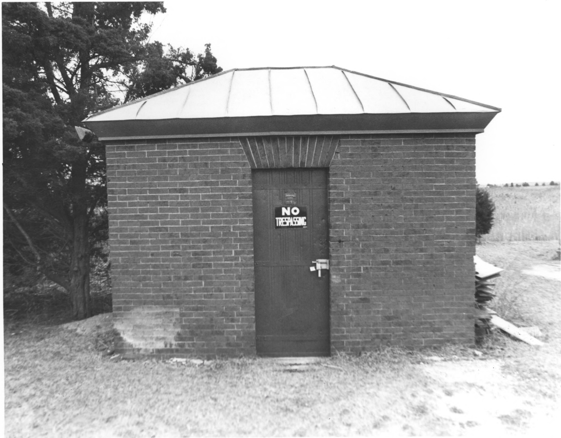
MAURICE RIVER LIGHTHOUSE, CUMBERLAND COUNTY, NJ # 31 of 34
