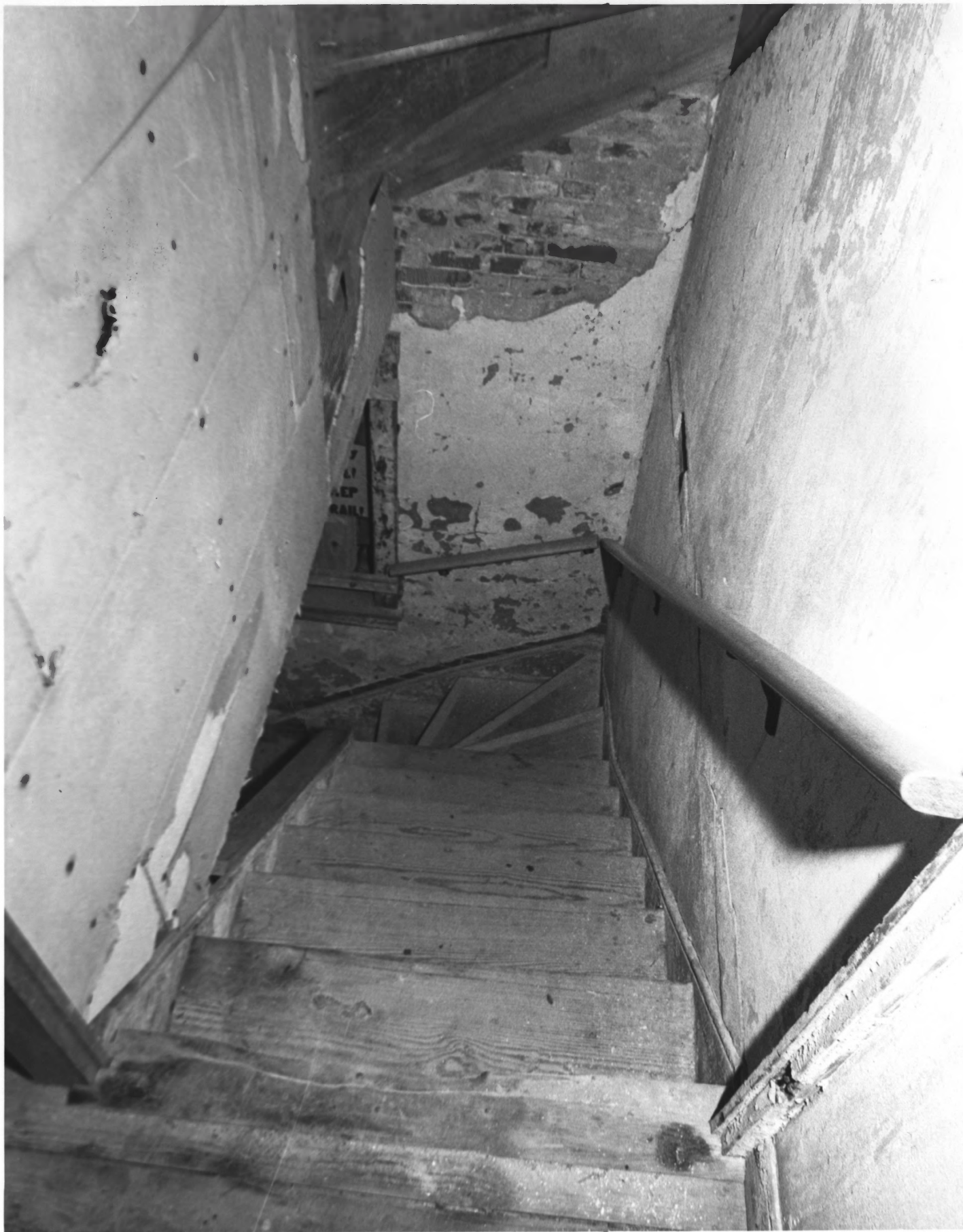
MAURICE RIVER LIGHTHOUSE, CUMBERLAND COUNTY, NJ # 22 of 34
