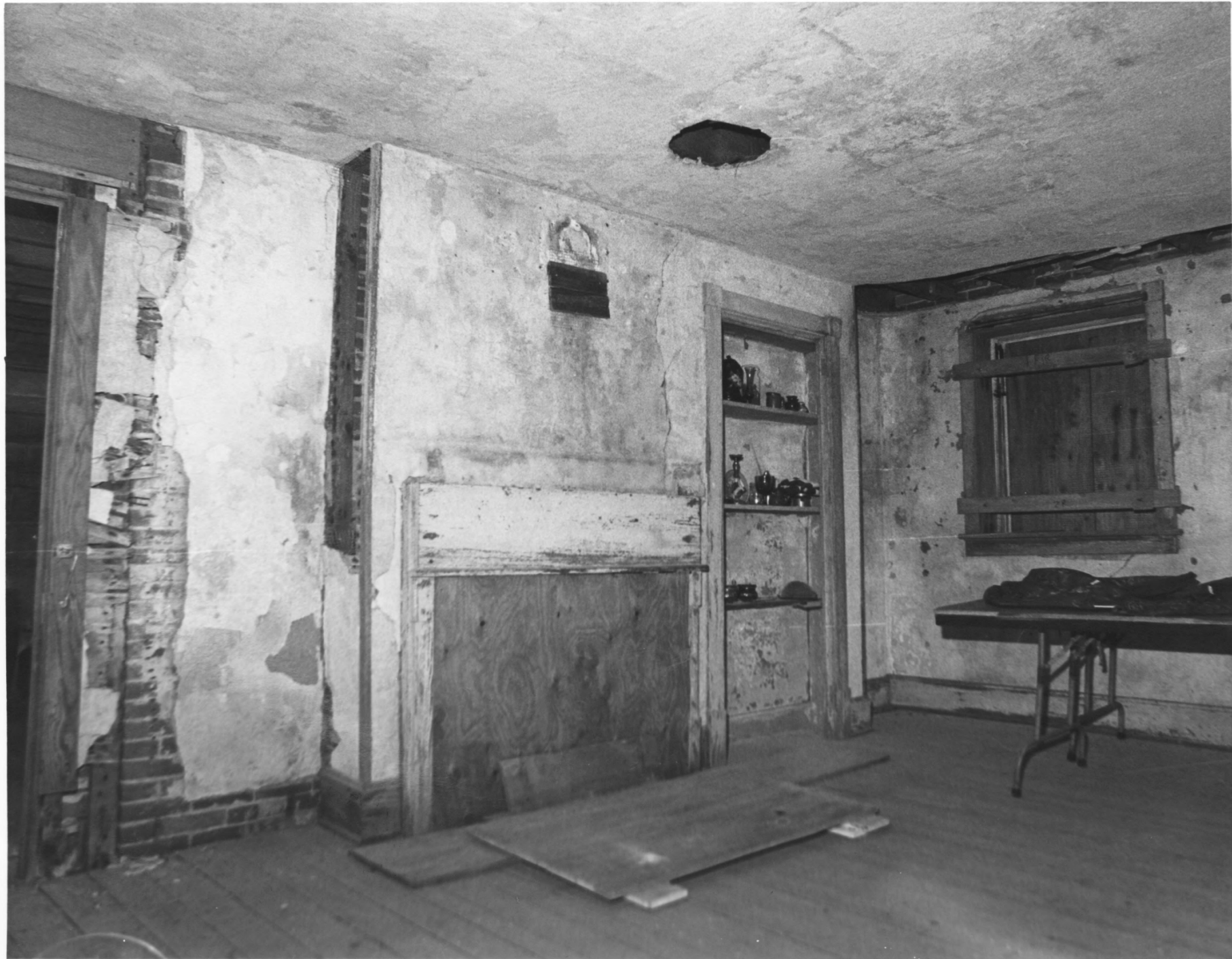
MAURICE RIVER LIGHTHOUSE, CUMBERLAND COUNTY, NJ # 17 of 34
