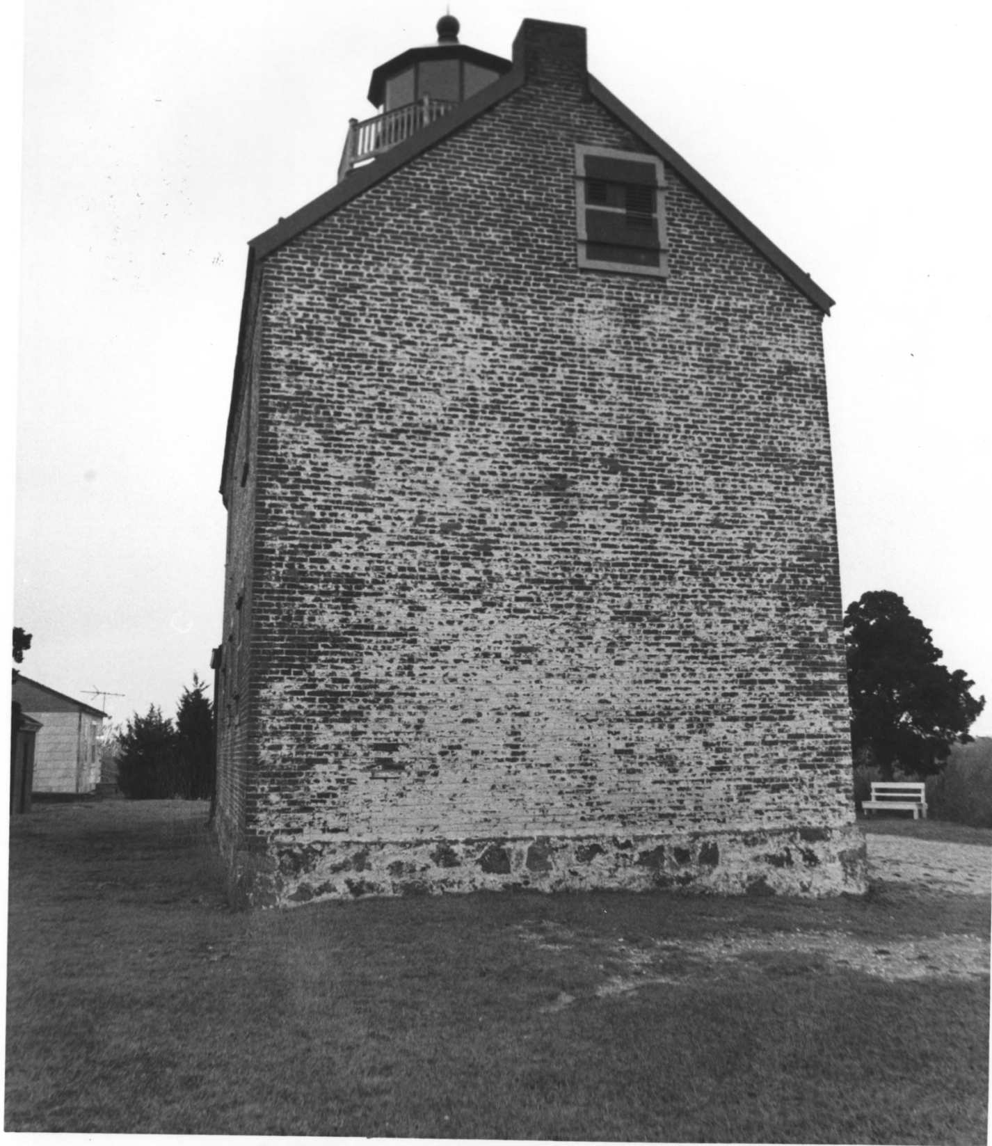
MAURICE RIVER LIGHTHOUSE, CUMBERLAND COUNTY, NJ # 10 OF 34
