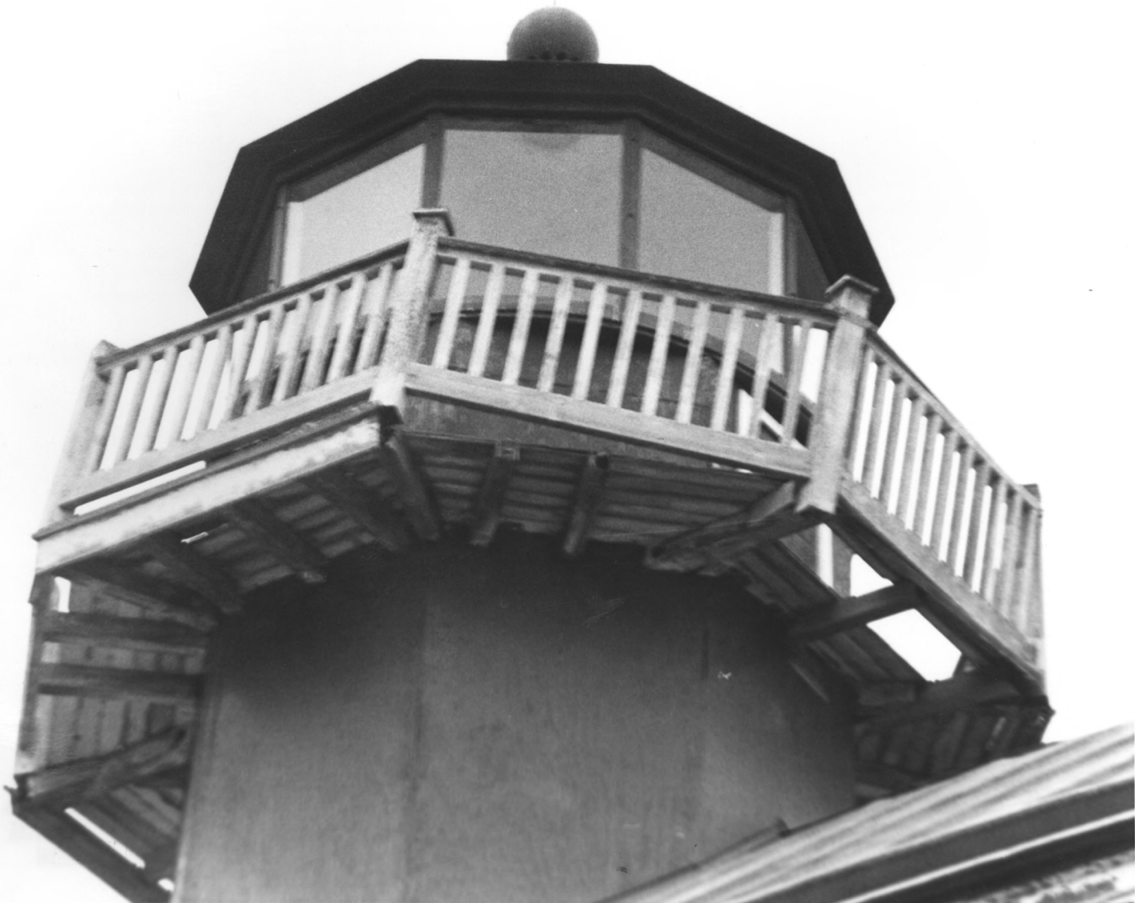
MAURICE RIVER LIGHTHOUSE, CUMBERLAND COUNTY, NJ # 14 OF 34
