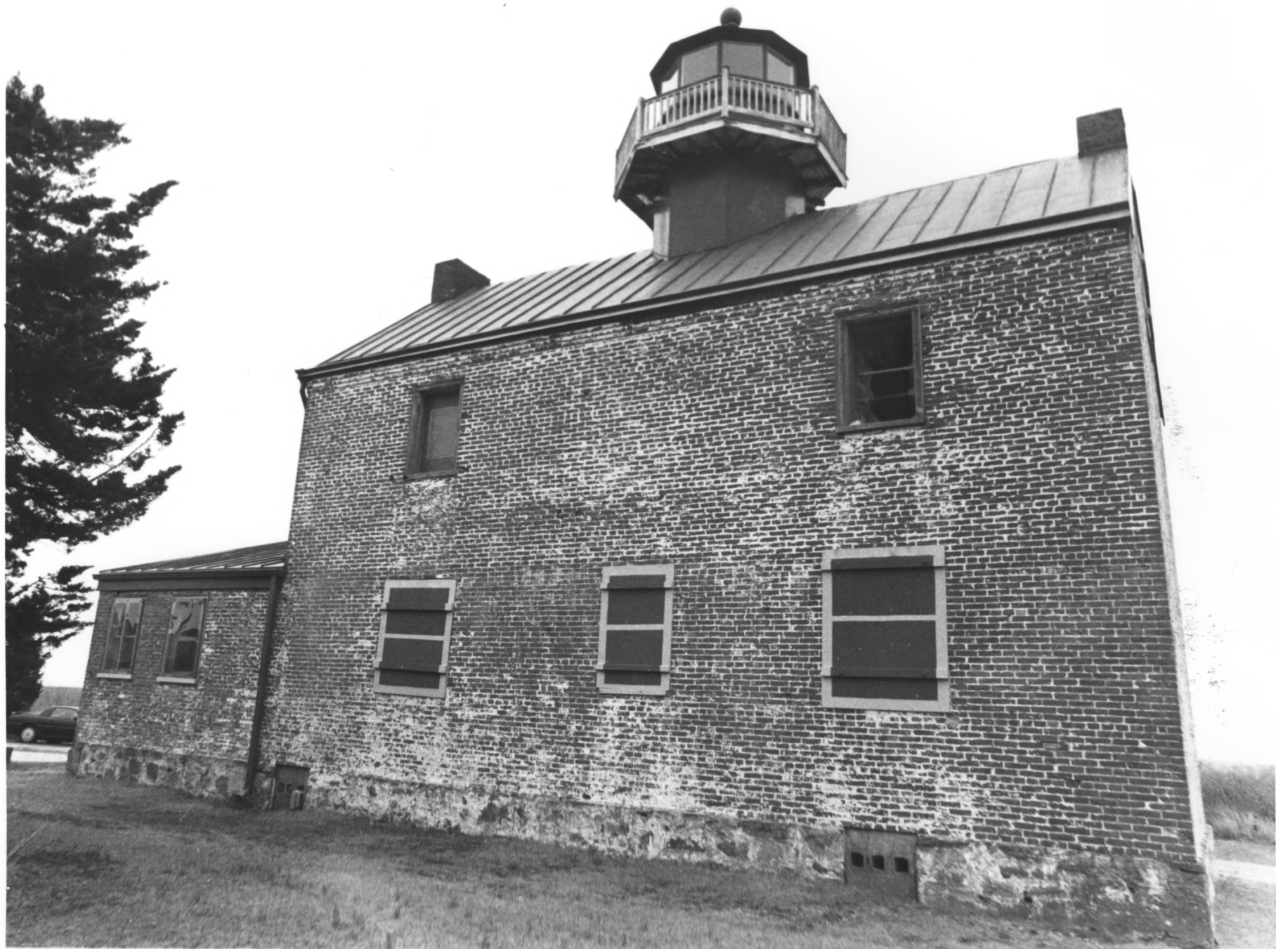
MAURICE RIVER LIGHTHOUSE, CUMBERLAND COUNTY, NJ # 11 of 34
