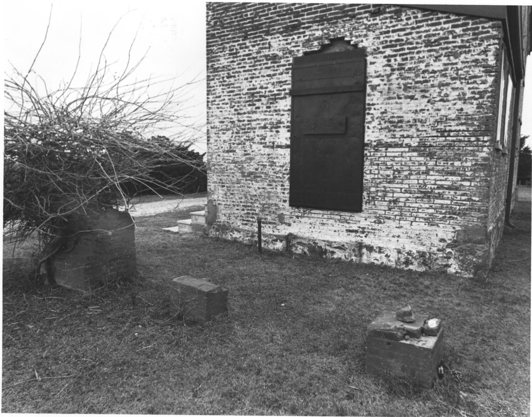
MAURICE RIVER LIGHTHOUSE, CUMBERLAND COUNTY, NJ #13 of 34
