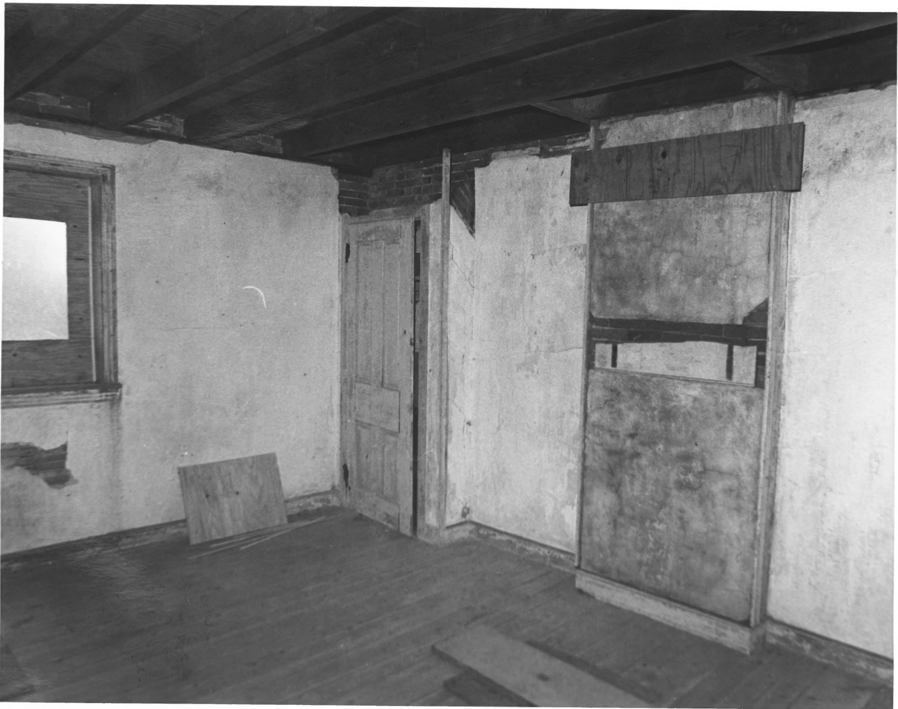
MAURICE RIVER LIGHTHOUSE, CUMBERLAND COUNTY, NJ # 23 of 34
