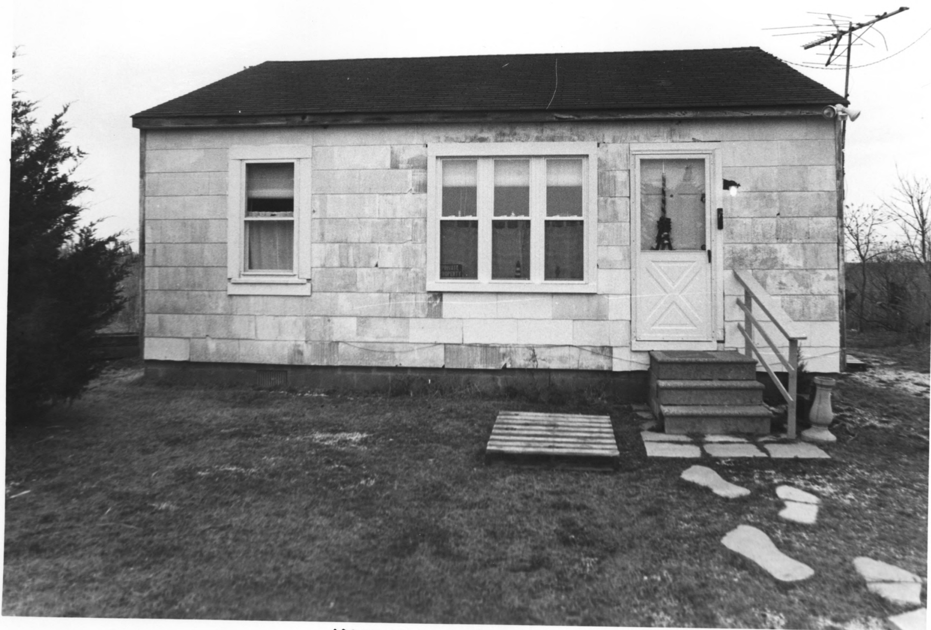
MAURICE RIVER LIGHTHOUSE, CUMBERLAND COUNTY, NJ # 34 of 34
