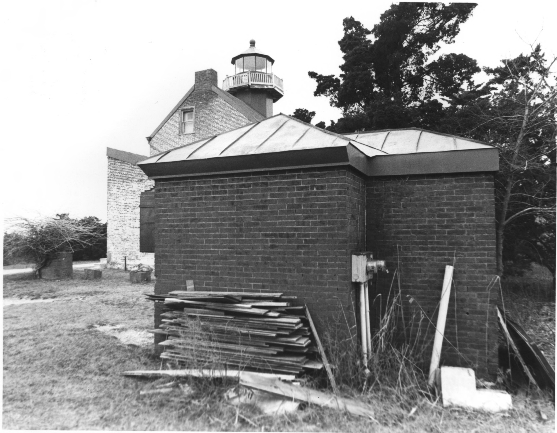
MAURICE RIVER LIGHTHOUSE, CUMBERLAND COUNTY, NJ # 33 of 34
