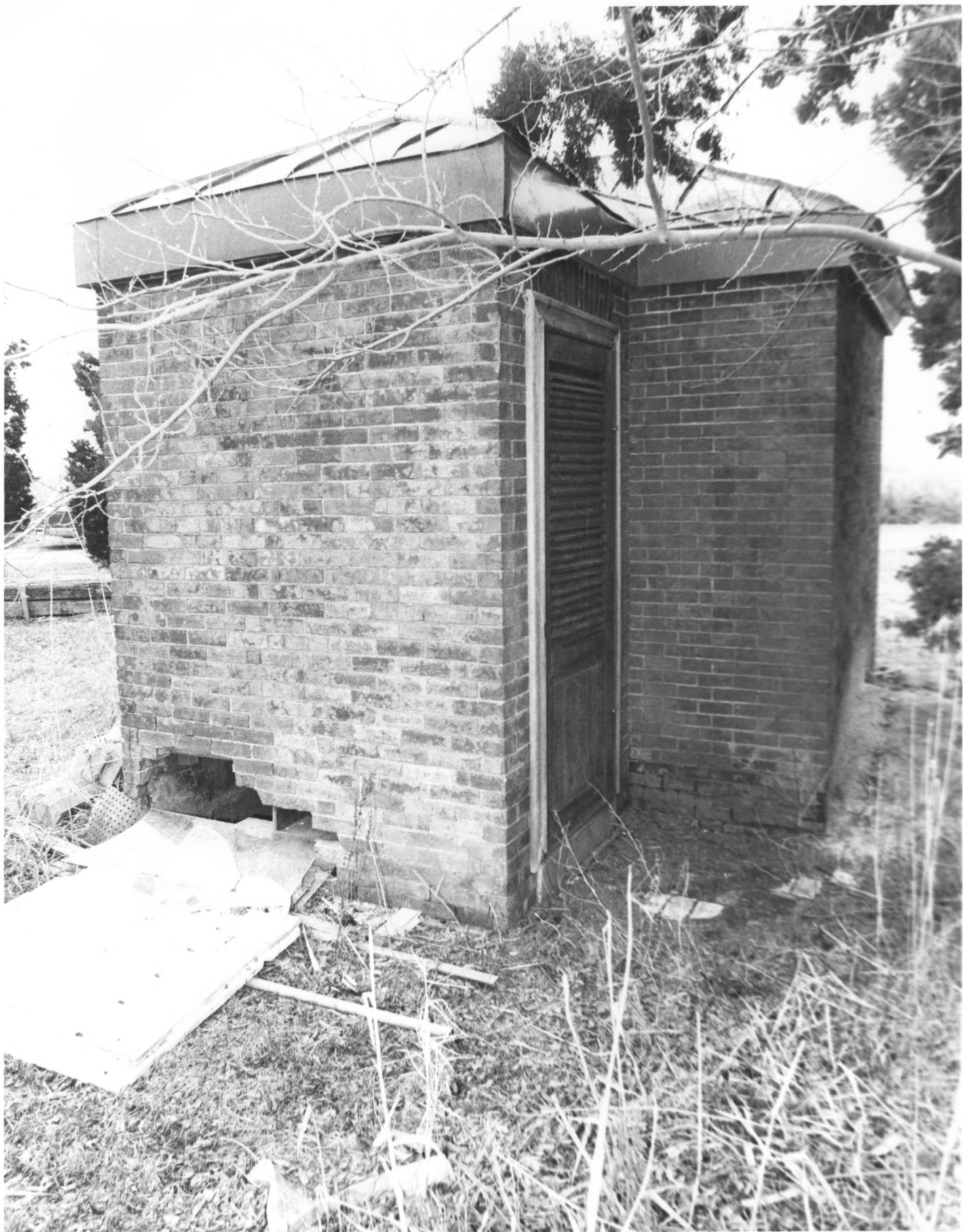
MAURICE RIVER LIGHTHOUSE, CUMBERLAND COUNTY, NJ # 32 of 34
