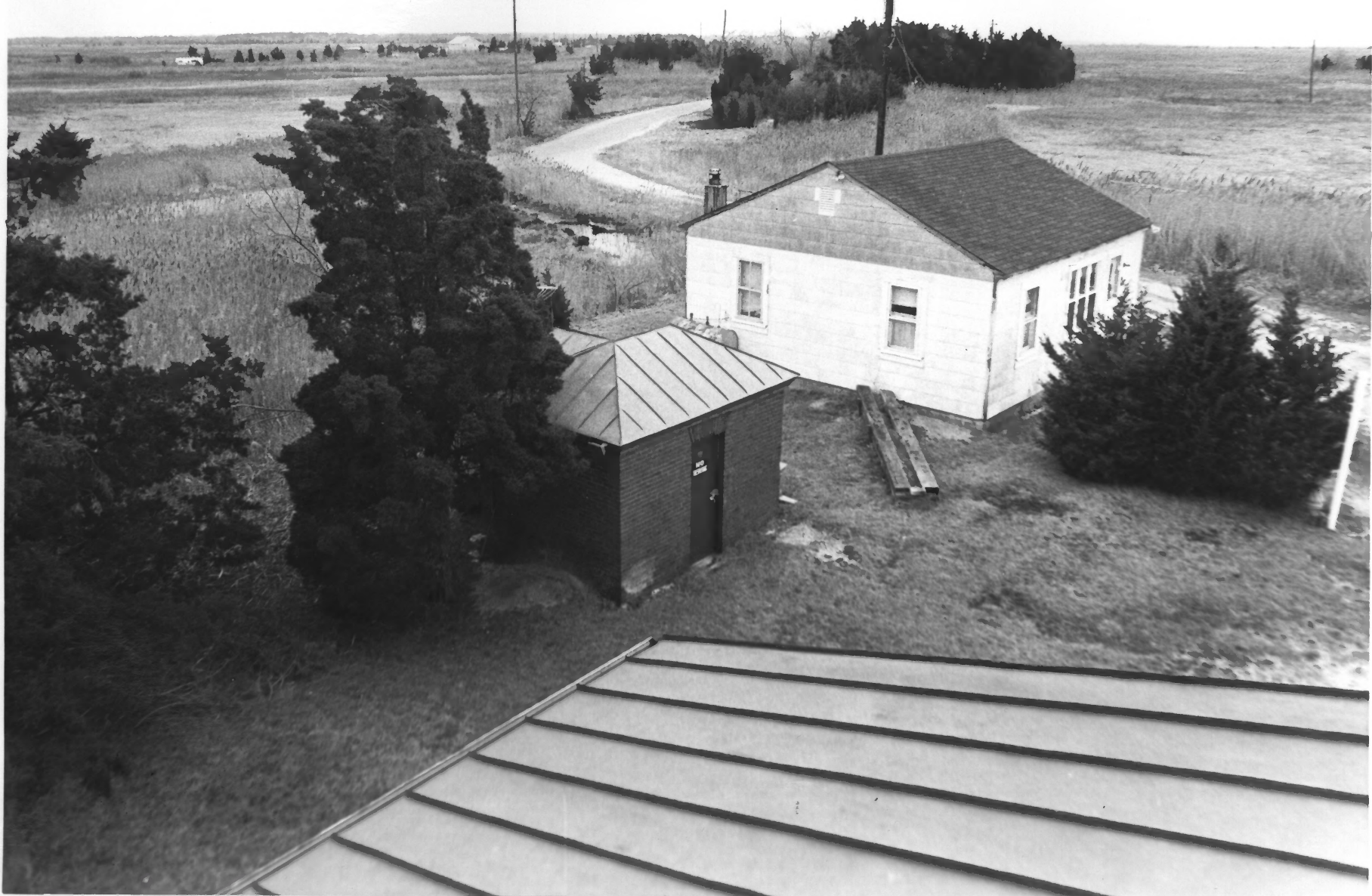
MAURICE RIVER LIGHTHOUSE, CUMBERLAND COUNTY, NJ # 27 of 34
