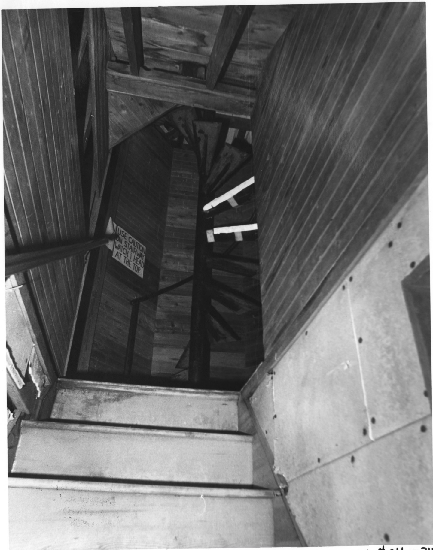
MAURICE RIVER LIGHTHOUSE, CUMBERLAND COUNTY, NJ # 24 of 34
