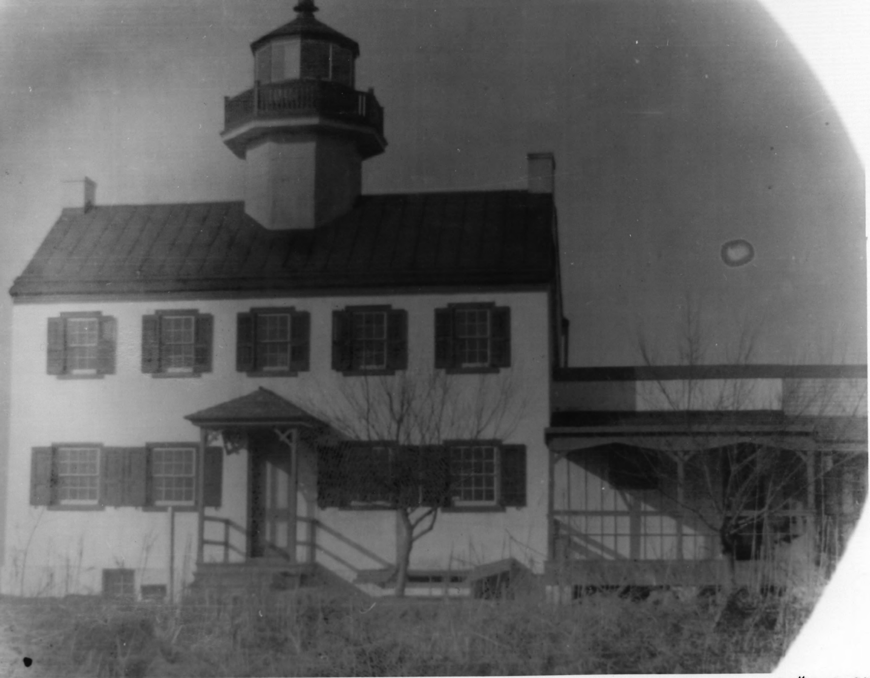
MAURICE RIVER LIGHTHOUSE, CUMBERLAND COUNTY, NJ, # 1 OF 34
