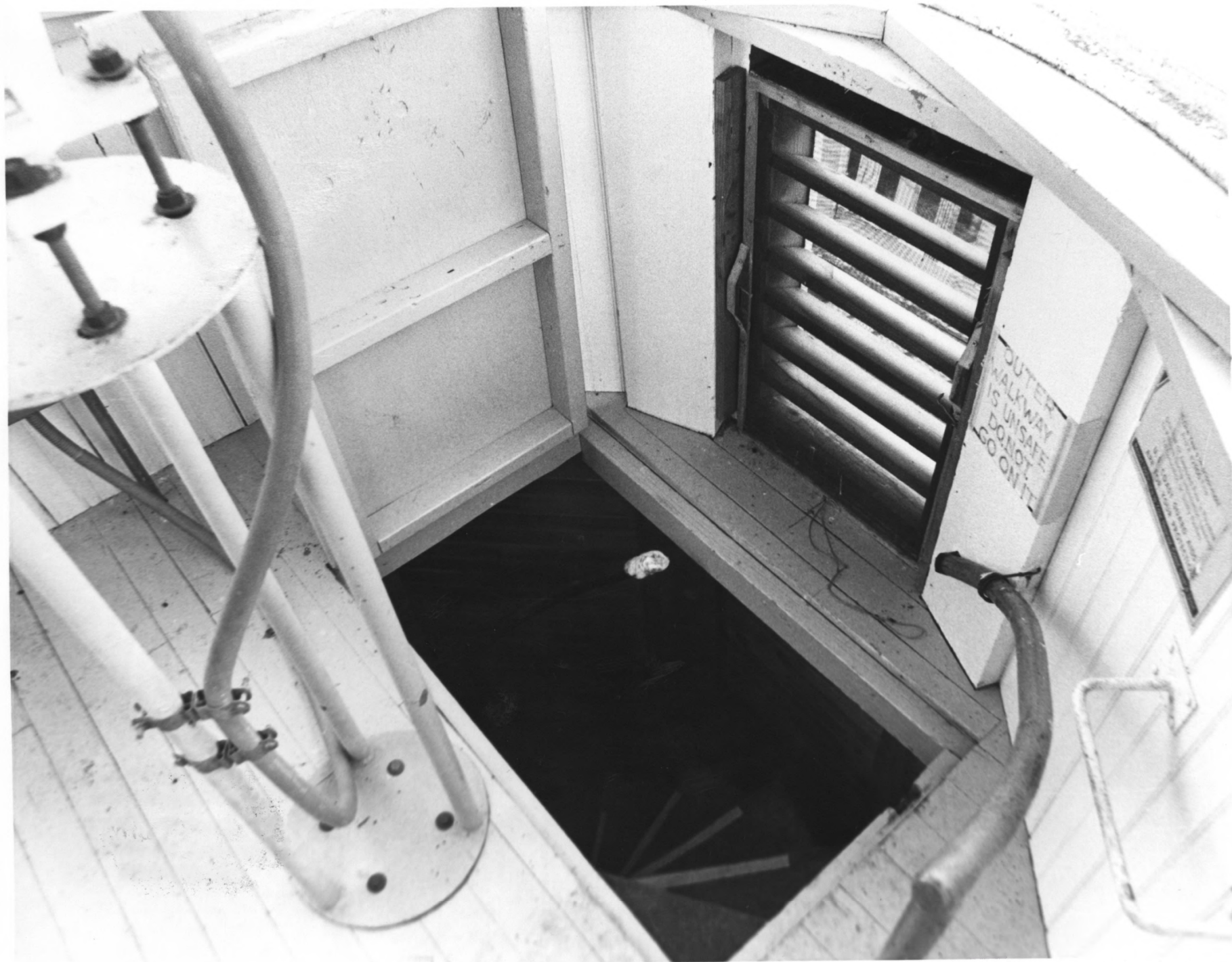
MAURICE RIVER LIGHTHOUSE, CUMBERLAND COUNTY, NJ # 30 of 34
