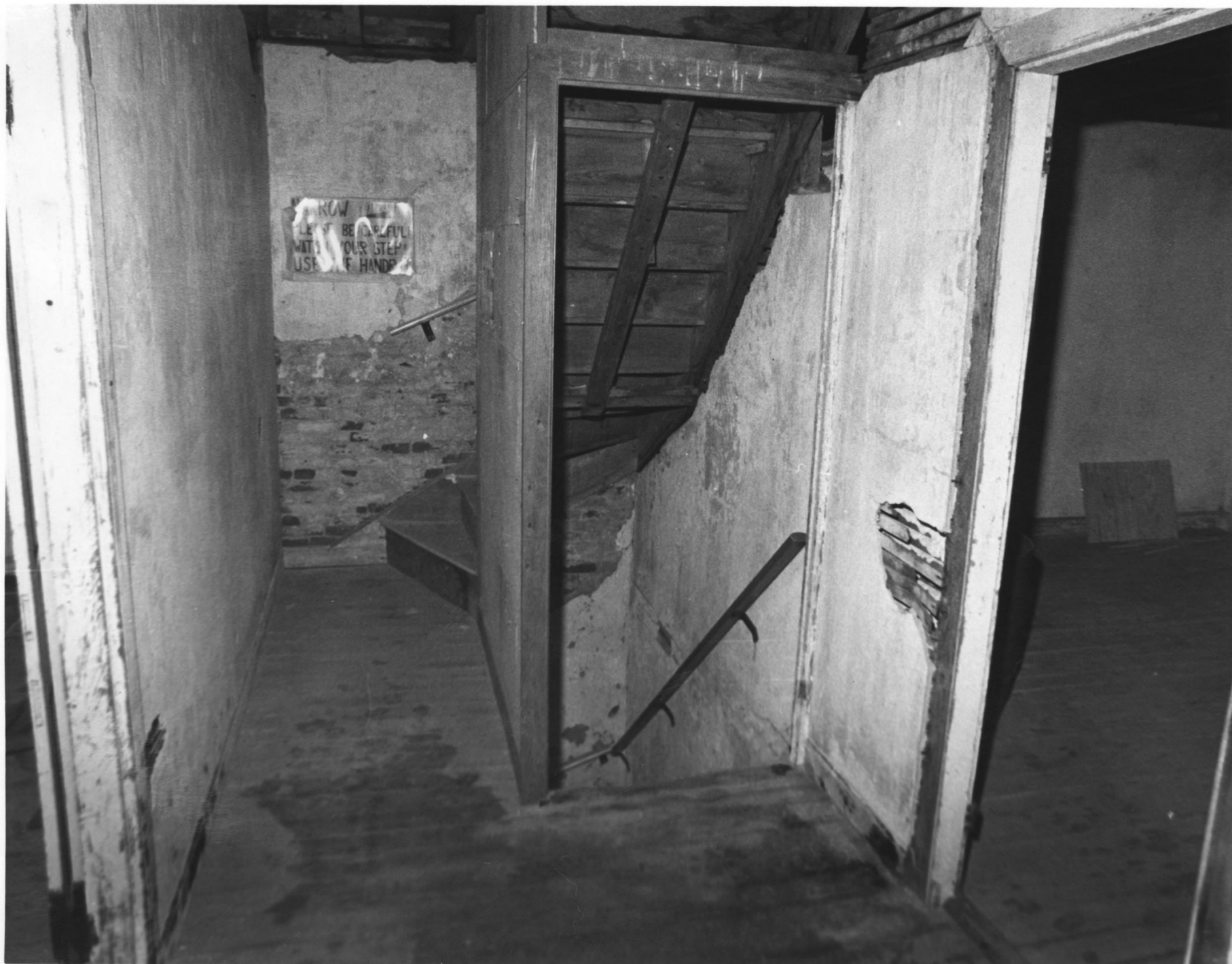
MAURICE RIVER LIGHTHOUSE, CUMBERLAND COUNTY, NJ # 21 of 34
