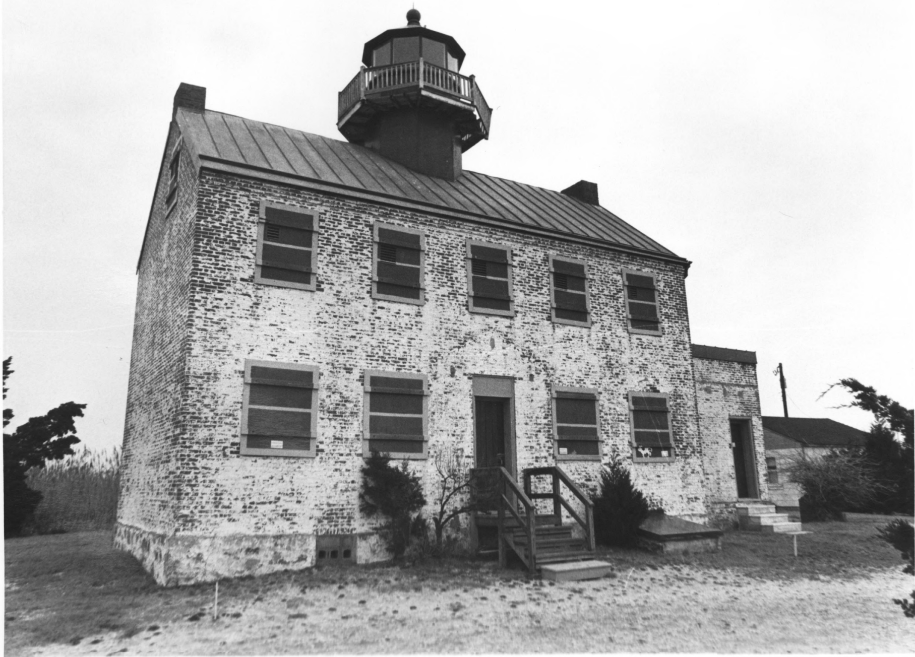
MAURICE RIVER LIGHTHOUSE, CUMBERLAND COUNTY, NJ # 8 of 34
