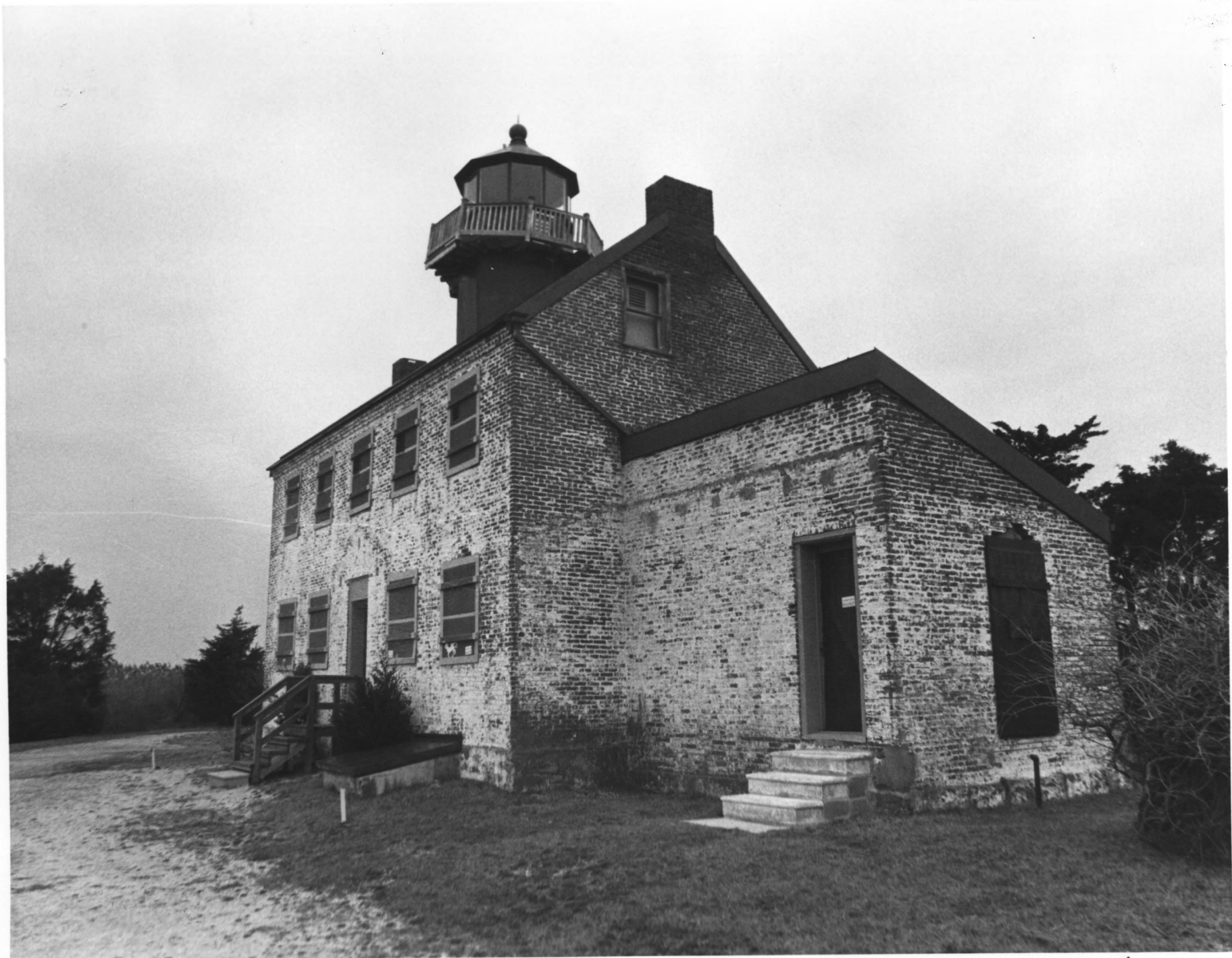
MAURICE RIVER LIGHTHOUSE, CUMBERLAND COUNTY, NJ # 12 of 34
