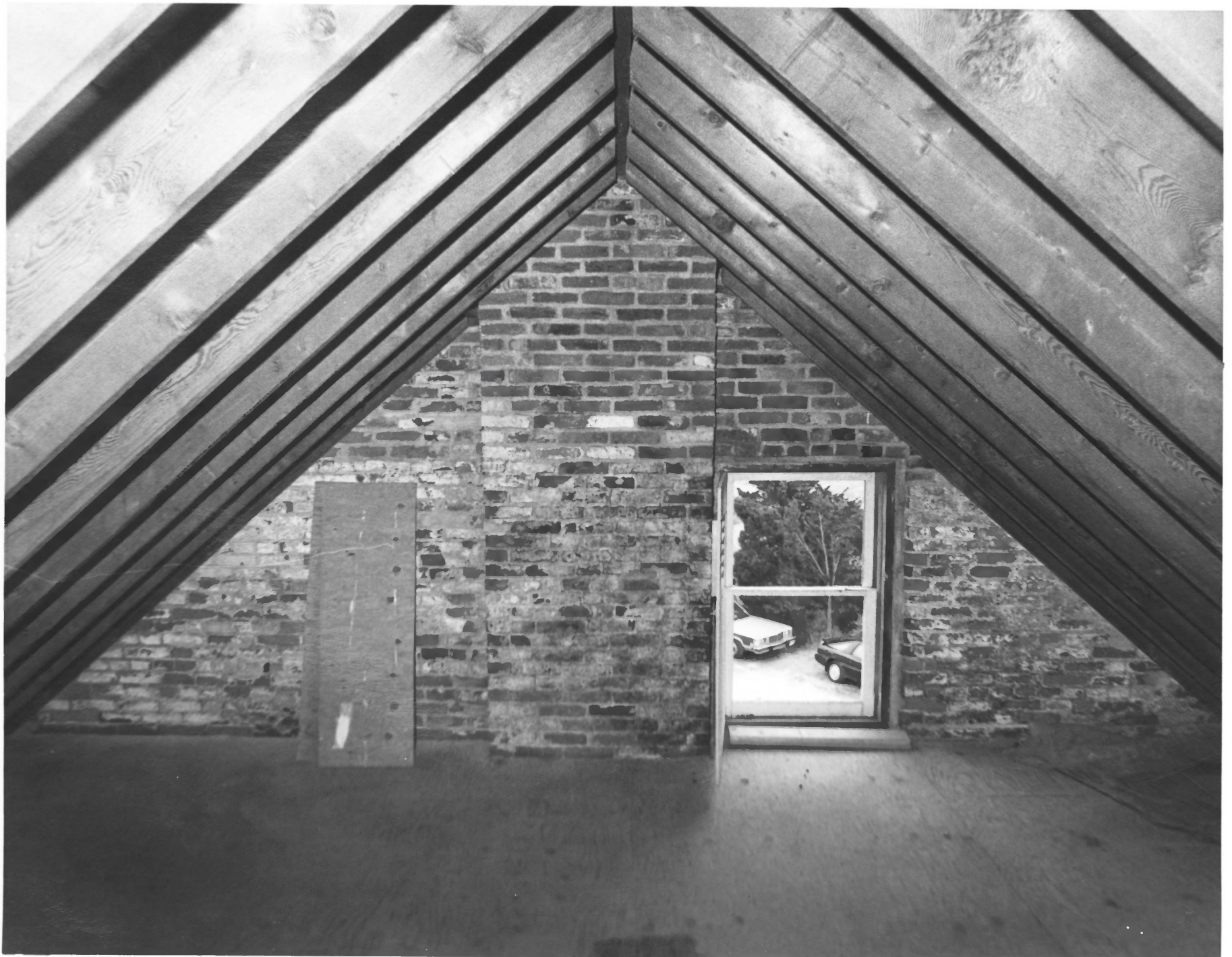
MAURICE RIVER LIGHTHOUSE, CUMBERLAND COUNTY, NJ # 26 of 34
