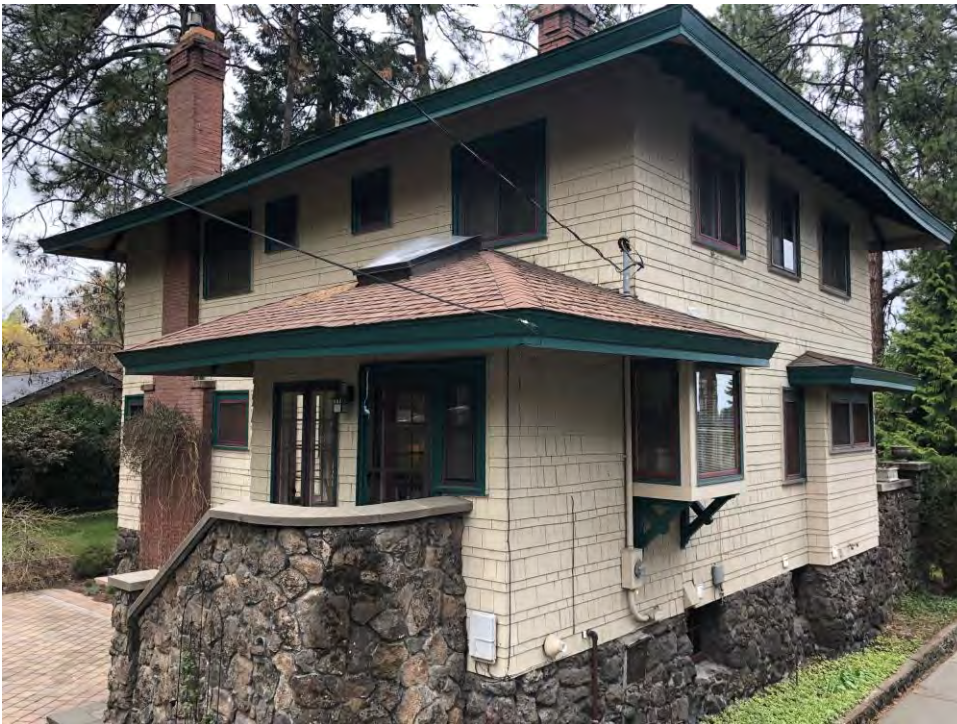
3 of 24. Southeast corner of McMullen-Dyar House showing rear kitchen wing.
