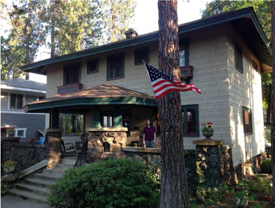
2 of 24. Northwest corner of McMullen-Dyar House showing verandah.
