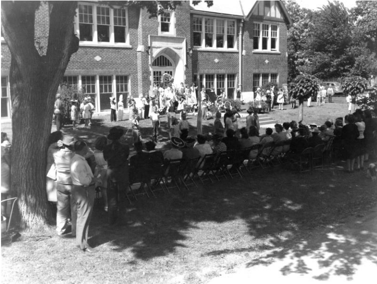
View of school from southwest.
