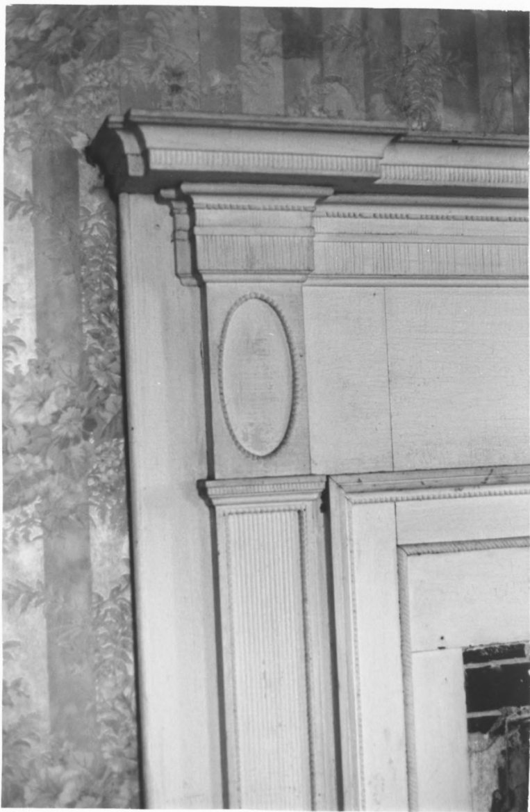
'Cottage Grove' . Bardstown, Nelson Co., Kentucky (NE-238)
