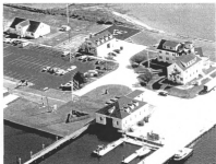
Figure 26: aerial view of the Atlantic City (Atlantic County, NJ) Coast Guard station
