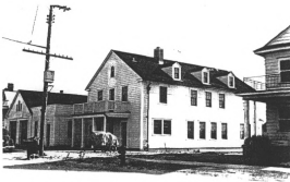
Figure 28: Ocean City Coast Guard station (Cape May County, NJ), 1936
