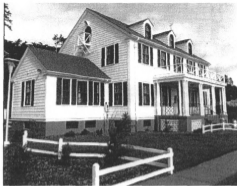
Figure 18: Yaquina Bay (OR) Coast Guard station, built in 1949
