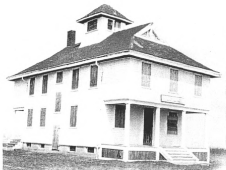
Figure 13: Chatham (Massachusetts) life-saving station, built in 1914
