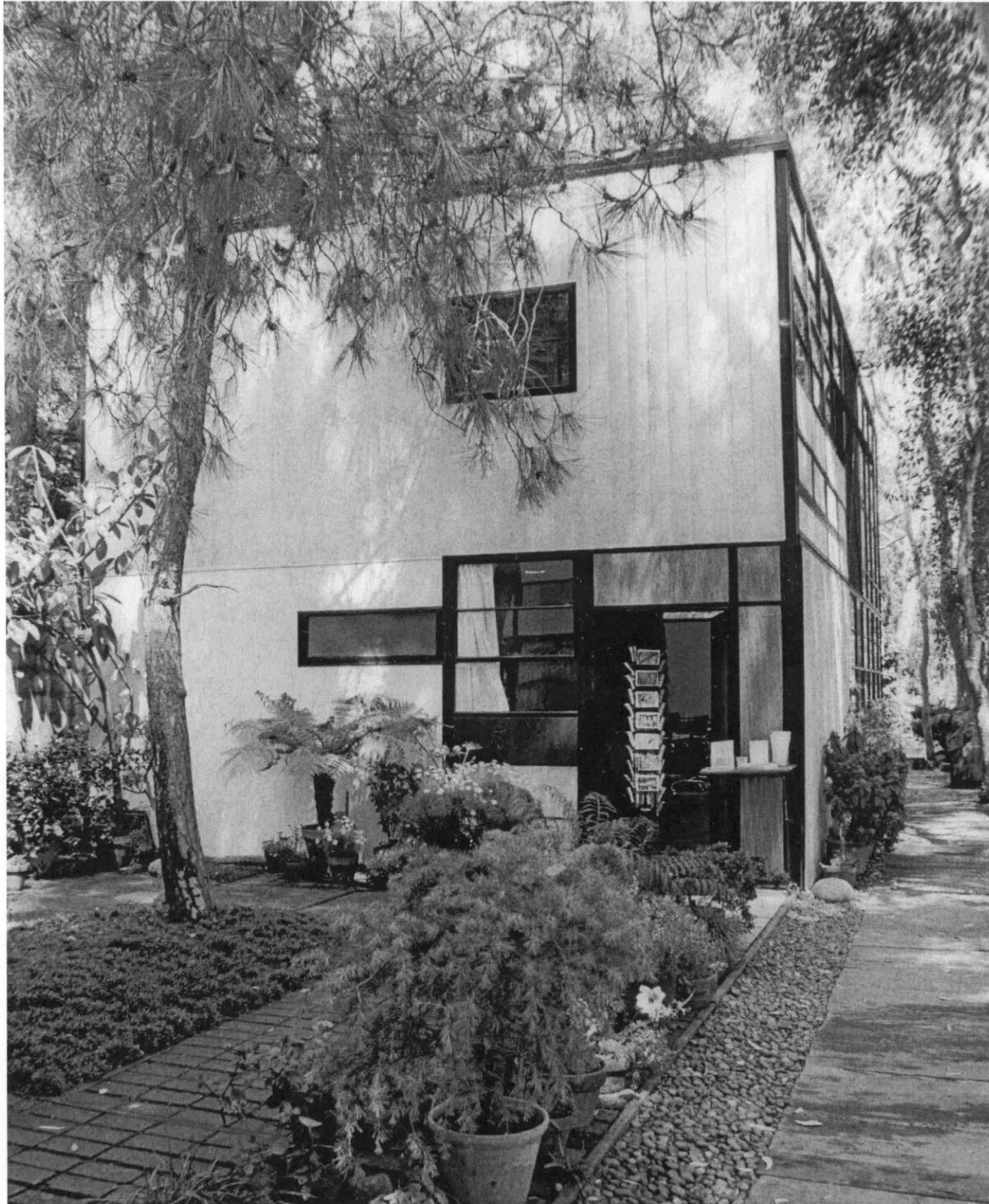
Eames House, Los Angeles, CA. South and East elevations of studio. Photo by Carly Caryn, April 2005.
