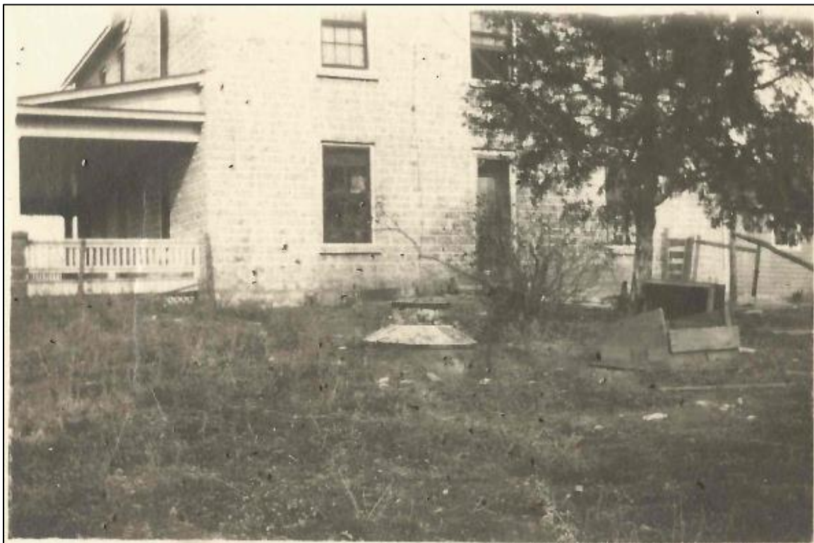
Figure 9: Circa 1920 photo of house, looking NE at south elevation and showing Craftsman-era porch.
