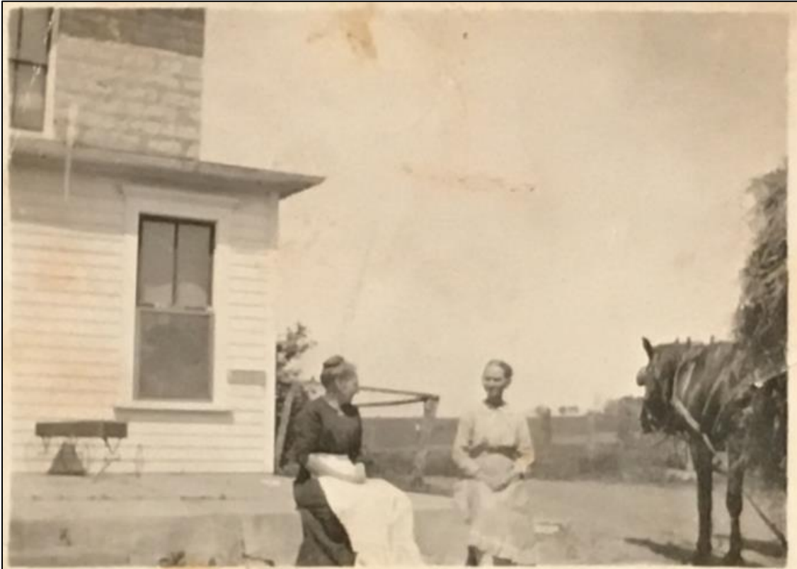
Figure 8: Circa 1917 photo of north side of house, looking WNW and showing one-story wood-framed porch where 1999 addition currently is located. The Craftsman porch had not yet been constructed.
