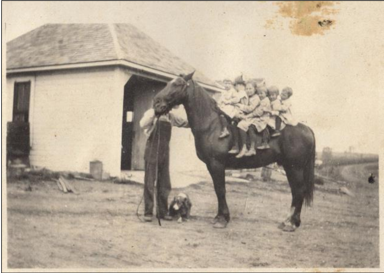
Figure 12: Circa 1920, showing garage in background.
