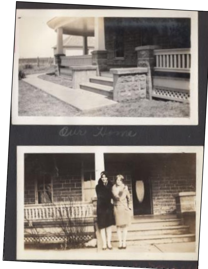
Figure 13: Circa 1939 photos showing house porch.
