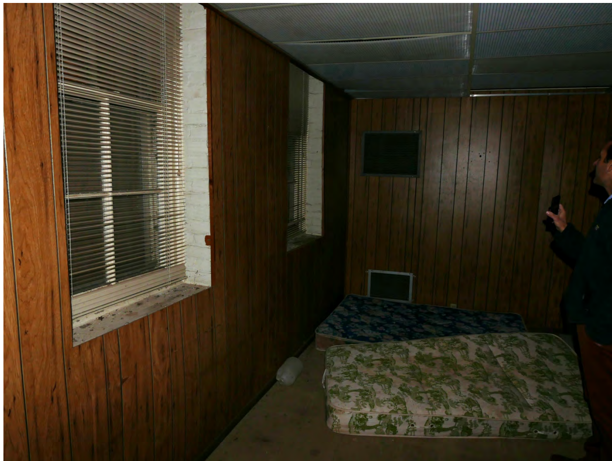
Figure 14: View inside of the first floor office area. Photograph by the preparer, January 2019.
