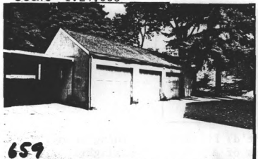
Building 659 serves as garage for Building 568 . The garage was constructed in 1947.
