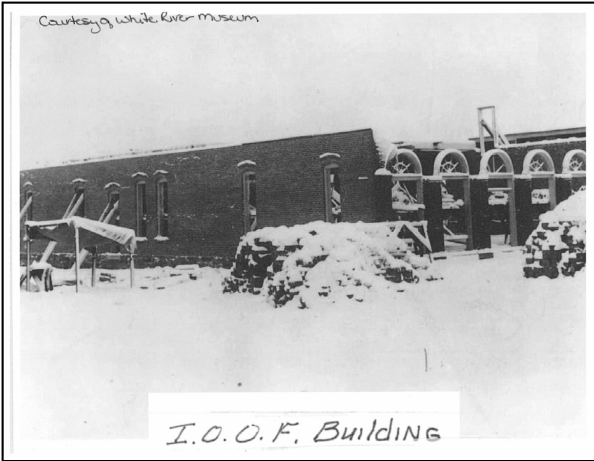
Figure 3: First floor of I.O.O.F. nearly complete, fall 1896 (Courtesy of White River Museum)
