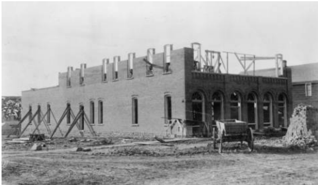
Figure 4: Start of I.O.O.F. second floor, fall 1896 (Courtesy Denver Public Library X-12458)
