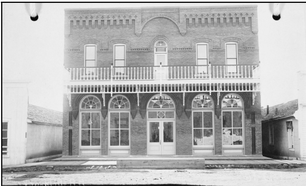
Figure 6: The Meeker Hotel after completion, circa August 1896, H. A. Wildhack, photographer (Courtesy of Denver Public Library X-12428)
