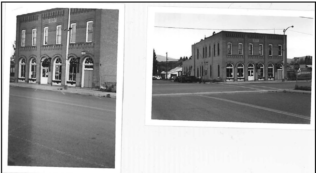
Figure 12: I.O.O.F. building 1977, on file with the Office of Archaeology and Historic Preservation, Denver, Colorado
