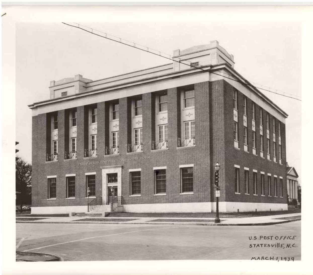
Figure 1 – Photograph of United States Post Office and Court House, Statesville, North Carolina, March 1, 1939 (National Archives and Records Administration RG121-BS_66_A_1)
