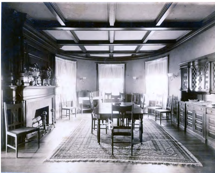
Figure 7: Wm. F. Clark photograph of the Reed House dining room, n.d. This view shows the original built-in sideboard and the unpainted oak finish of the trim Wm F. Clark, View Photographer, 338 Washington Street, Boston. Collection of Judith Rosbe.
