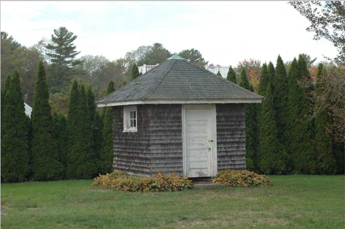
14. Reed pump house, camera facing northwest. (Photograph: Claire W. Dempsey, October 2016).
