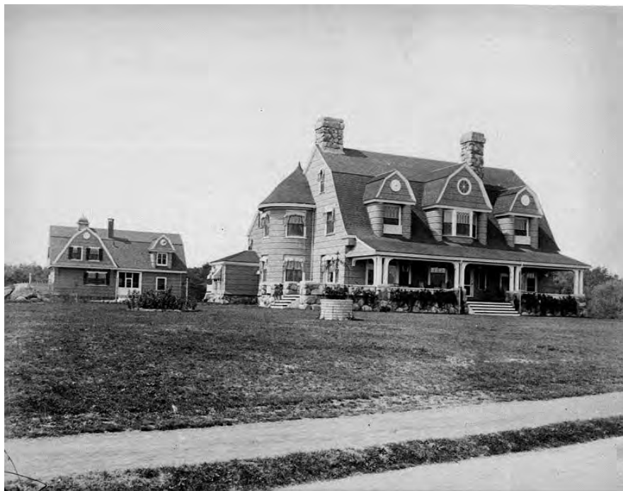
Figure 6: Soule Art Company photograph of the Reed House exterior, probably 1893. This image is one of a group probably commissioned by the architect, James T. Kelley. Courtesy of Historic New England.
