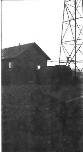
Figure 6. Site 32 Power house with the ground directional arrow visible in the foreground looking northwest (circa 1929). Arrow is pointing southeast towards Site 33, Rock River. Cole-Keller Collection.
