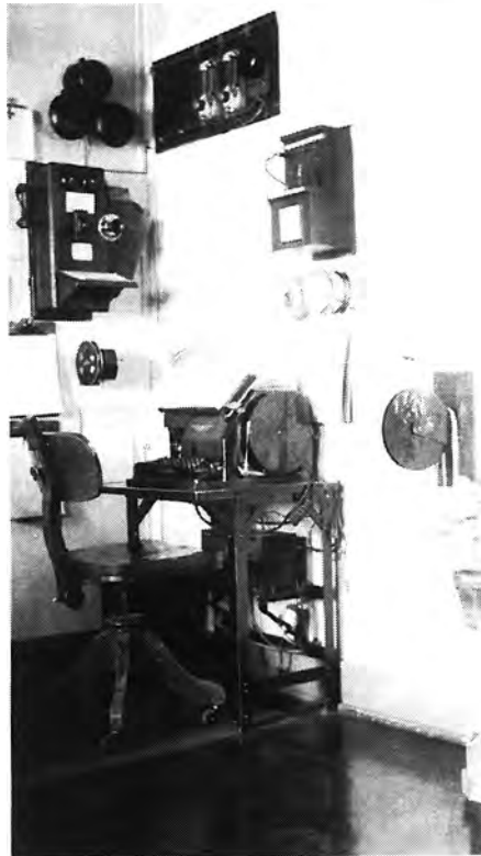
Figure 7. Site 32 interior of the two room office looking northeast. The teletype machine is against the east wall. The barometer, and wind speed and direction indicator are circular objects above the teletype machine. Above the telephone are bells to alert the operator when to begin entering station conditions after previous station was through transmitting. Airway Keepers were certified weather observers and were required to have a teletype capability of 35 words per minute. The presence of the telephone indicates this photo was taken about 1935. Cole-Keller Collection.
