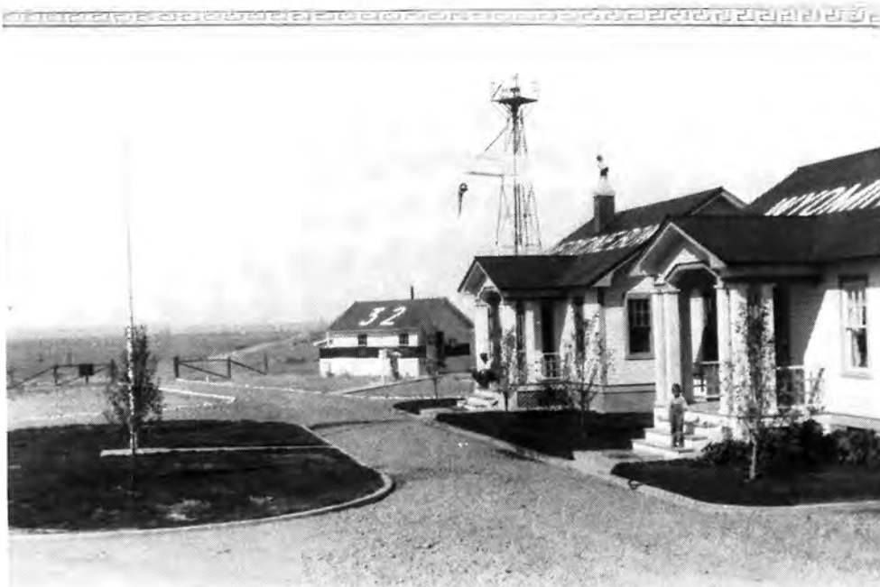
Figure 8. Site 32 office, tower, Airway Keeper's quarters, and flag pole looking northwest (circa 1933) Note well kept grounds and roof lettering to identify the site to pilots. Airway patrol pilots would often note the condition of the site in addition to the operation of the beacon and radio range and report such things as unmown lawns and weeds against buildings to district headquarters.
