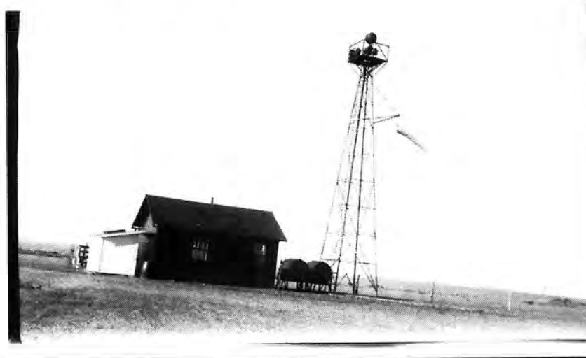
Figure 4. Site 32 power house and beacon tower looking north. Note the presence of the two 515 gallon fuel tanks between the tower and power house. White lean-to structure attached to the west end of power house held coal (circa 1929). Cole-Keller collection.
