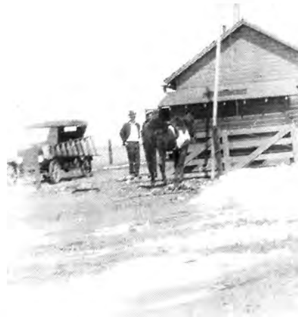
Figure 9. Site 31 Medicine Bow— between 1924-1929 one mile west of Site 32 and partially located on the present site of the Wyoming Department of Highways maintenance facilities. U.S. Highway 30 bisects the former site.
