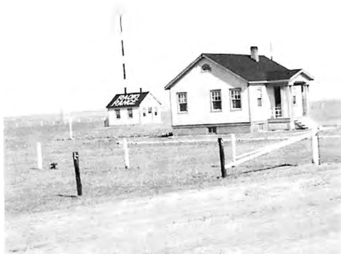
Figure 5. Site 32 Supervisor's house and radio range transmitter building looking northeast (circa 1933). Dimensions of the house were 22 x 28 feet and referred to as "K" quarters. The striped wooden poles, of which there were five, supported the antenna array of the low frequency radio range. Cole-Keller Collection.
