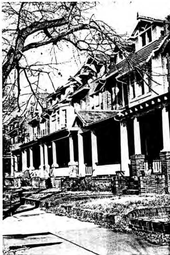
17 - 100 block N. Boulevard, view looking NE
