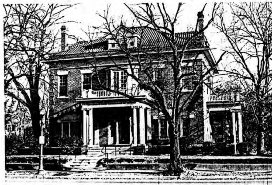
13 - 311 S. Boulevard; view looking E
