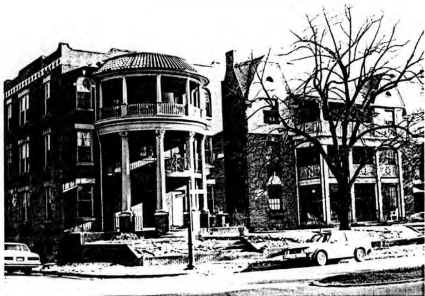
23- 301 and 303 S. Boulevard view looking SE
