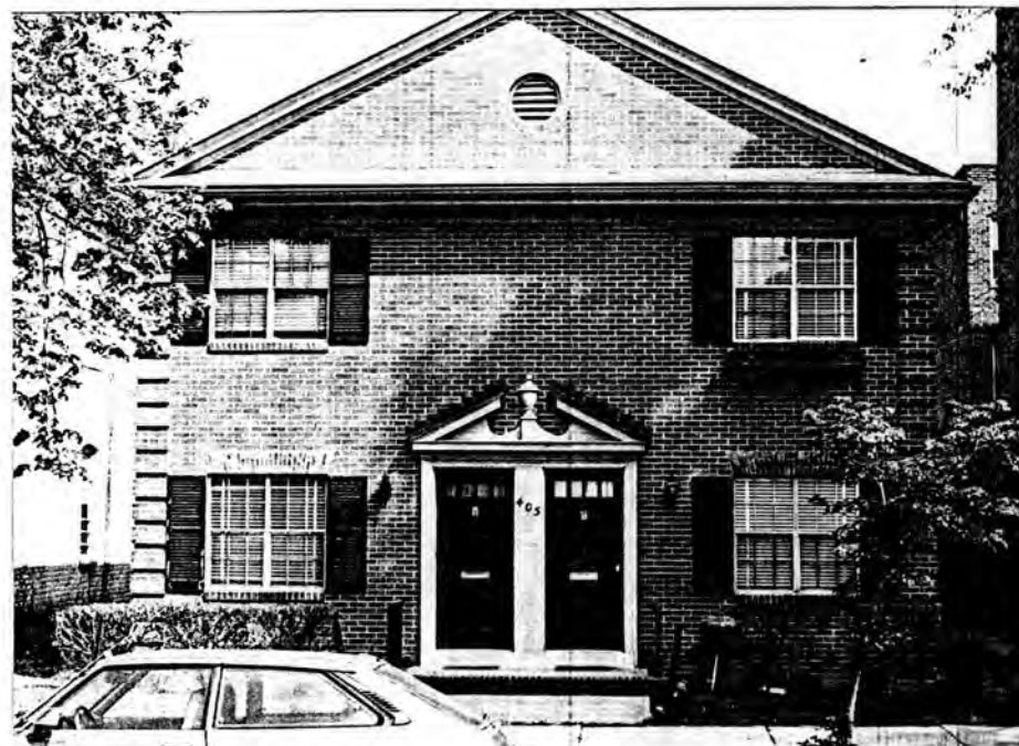
26 - 405 N. Boulevard; view looking E noncontributing building
