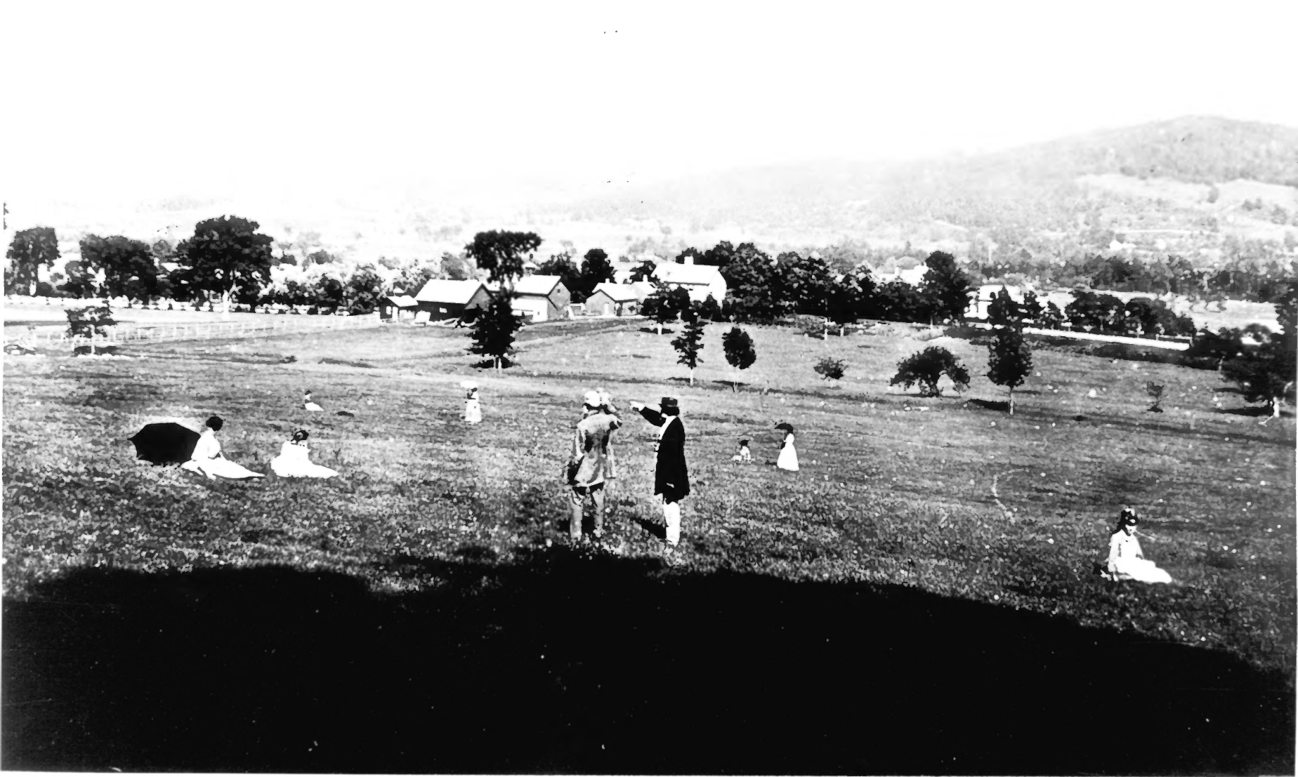
Photo B: Looking northeast across Arrowhead lands toward the Melville House and farm buildings. Berkshire County Historical Society. Date 1870.
