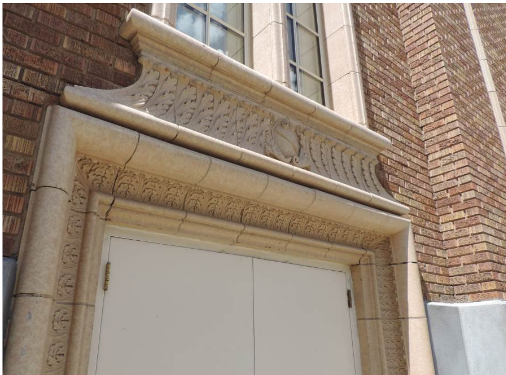
Photo 12 of 22: Door and window trim detail. Camera facing north.
