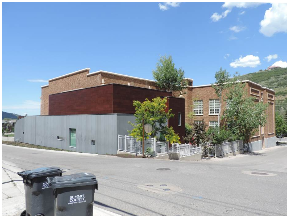
Photo 4 of 22: South and west elevations. Camera facing northeast.
