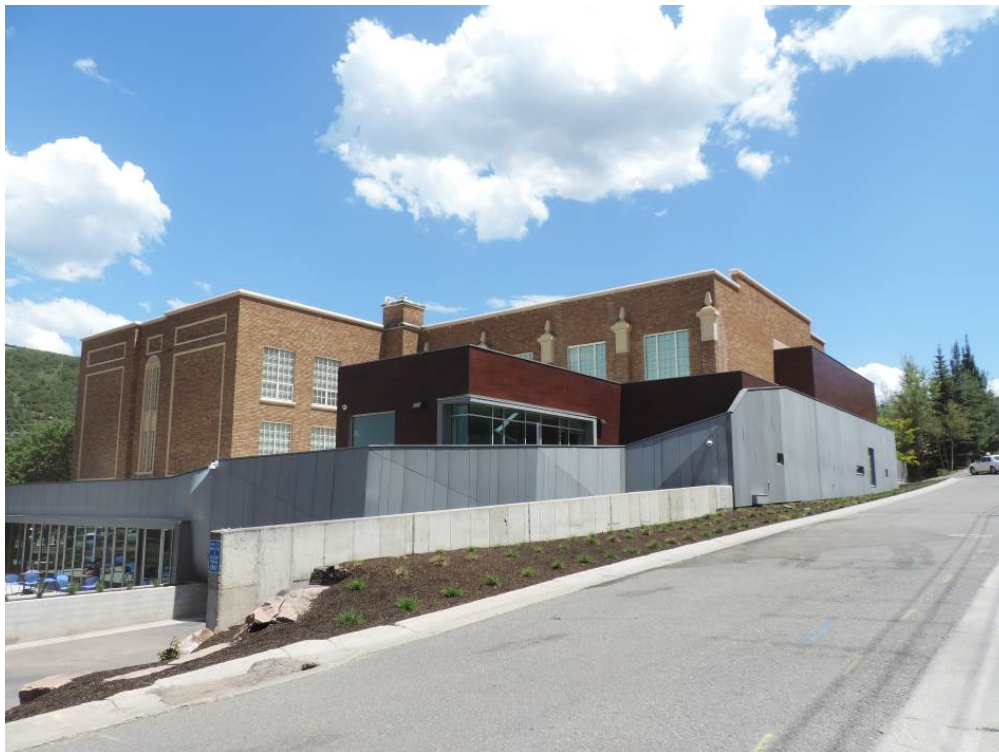
Photo 6 of 22: North and west elevations. Camera facing southeast.
