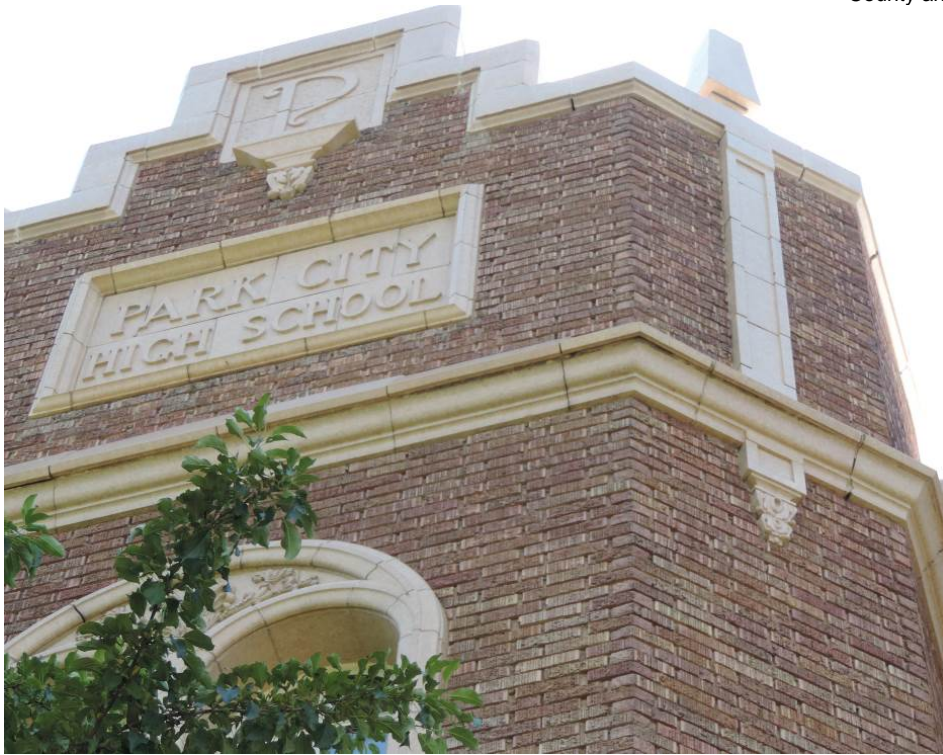
Photo 11 of 22: Portico top detail. Camera facing west.
