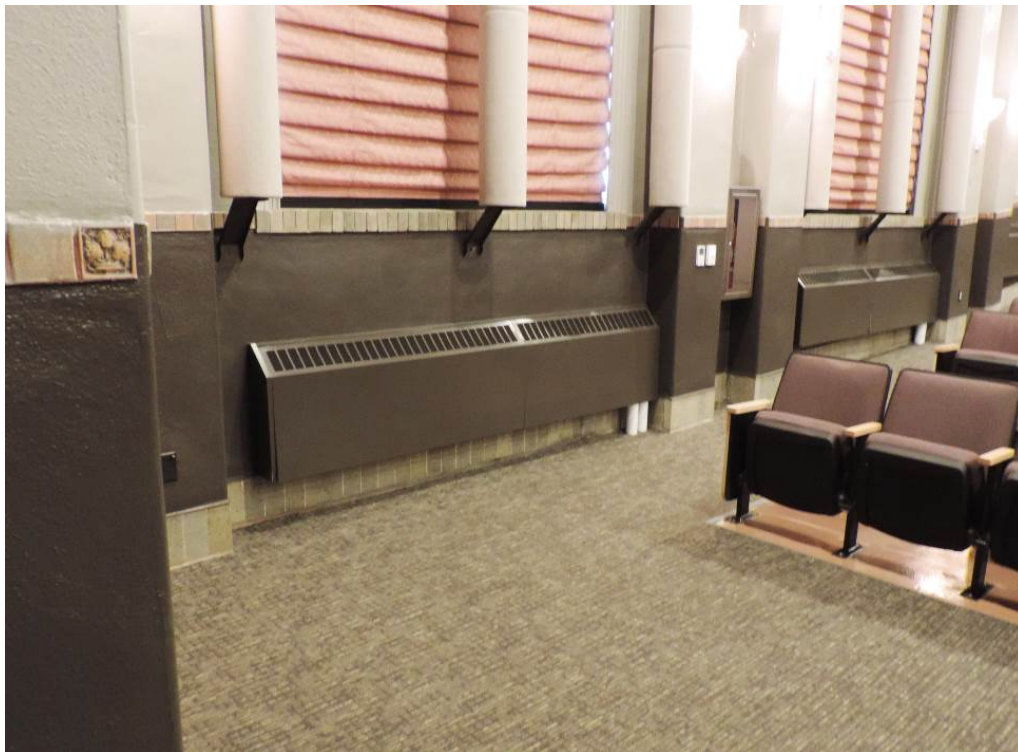
Photo 16 of 22: Santy Auditorium wainscot detail. Camera facing north.
