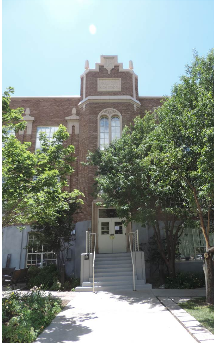
Photo 2 of 22: East portico. Camera facing west.
