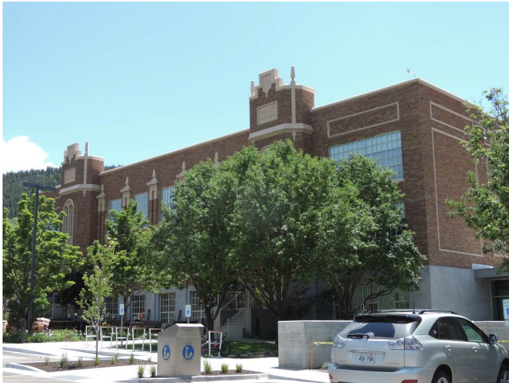
Photo 1 of 22: North and east elevations. Camera facing southwest.
