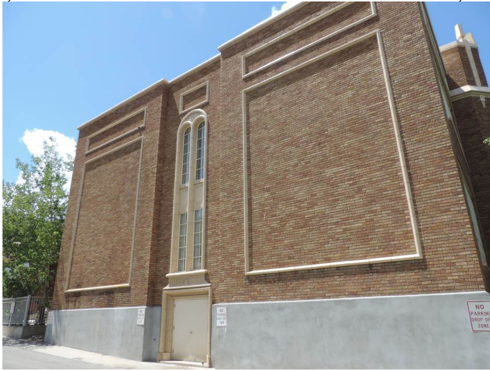
Photo 3 of 22: South elevation. Camera facing northwest.
