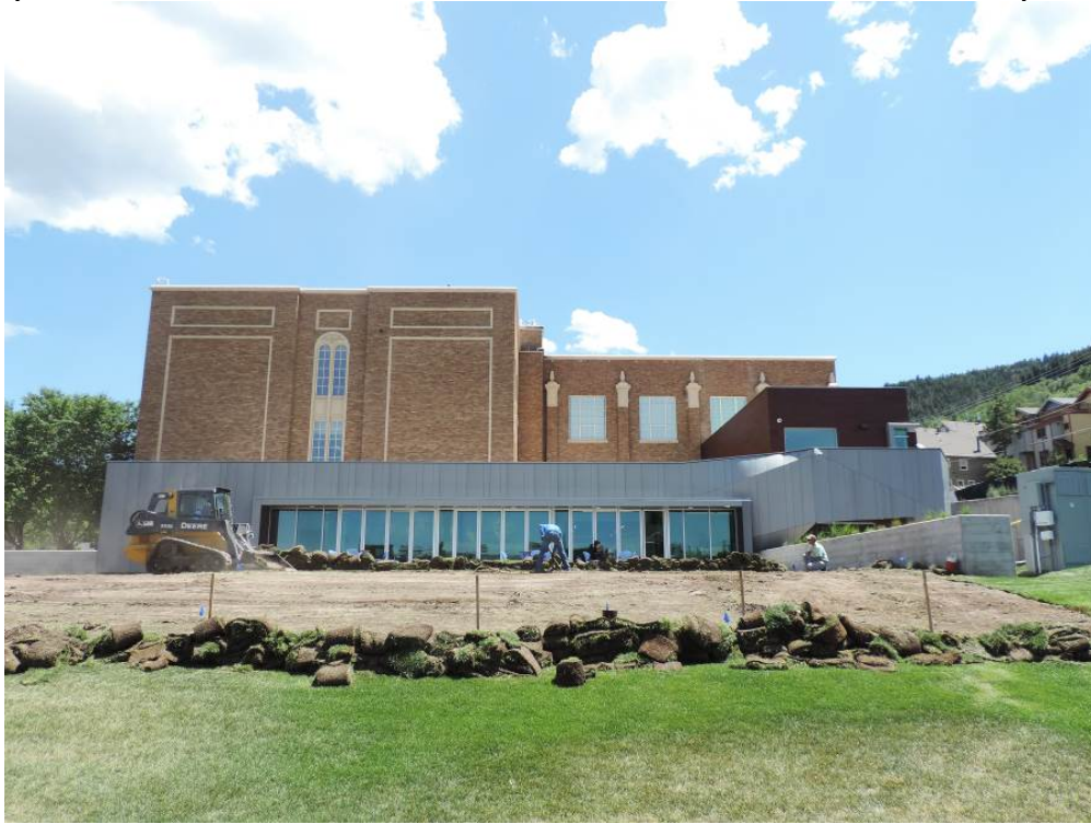
Photo 7 of 22: North elevation. Camera facing south.
