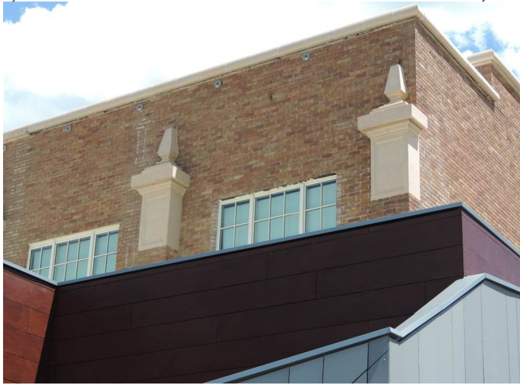
Photo 13 of 22: Pilaster crown detail. Camera facing southeast.
