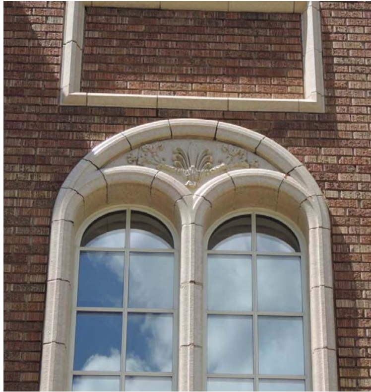
Photo 9 of 22: Terra cotta window trim detail. Camera facing south.
