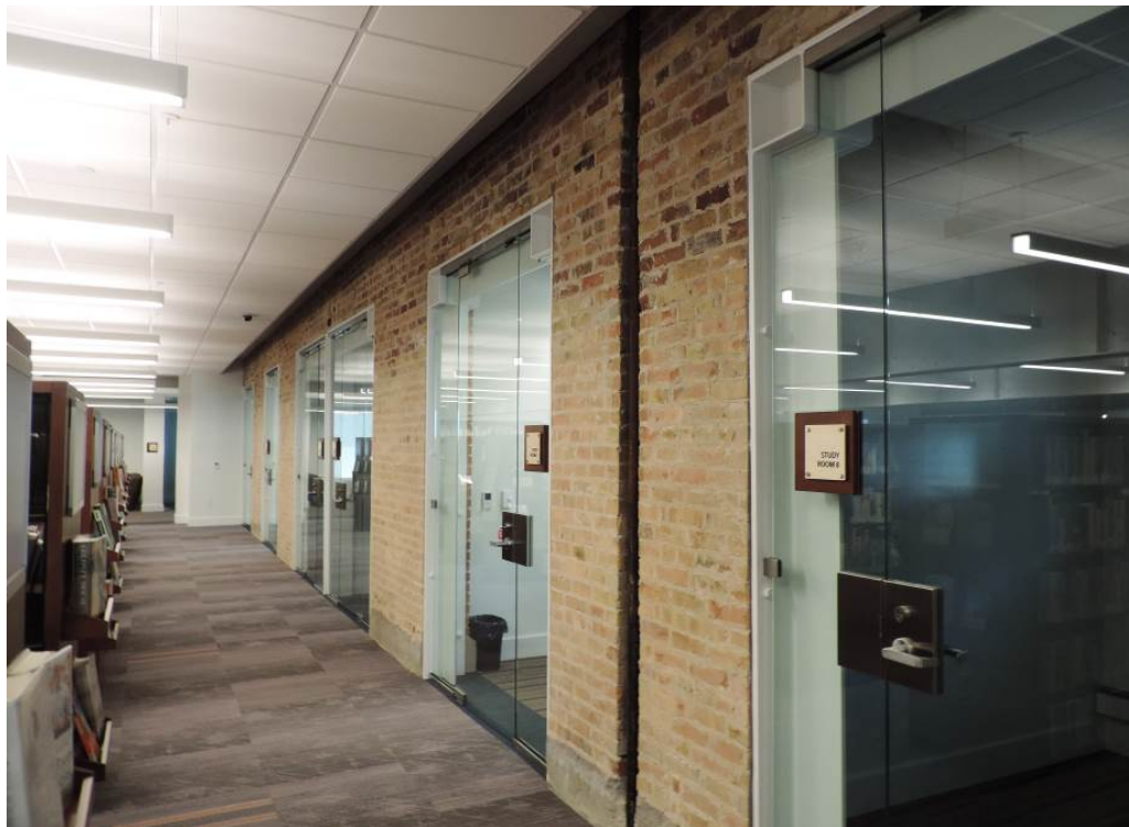
Photo 20 of 22: Inside of original exterior wall. Camera facing south.
