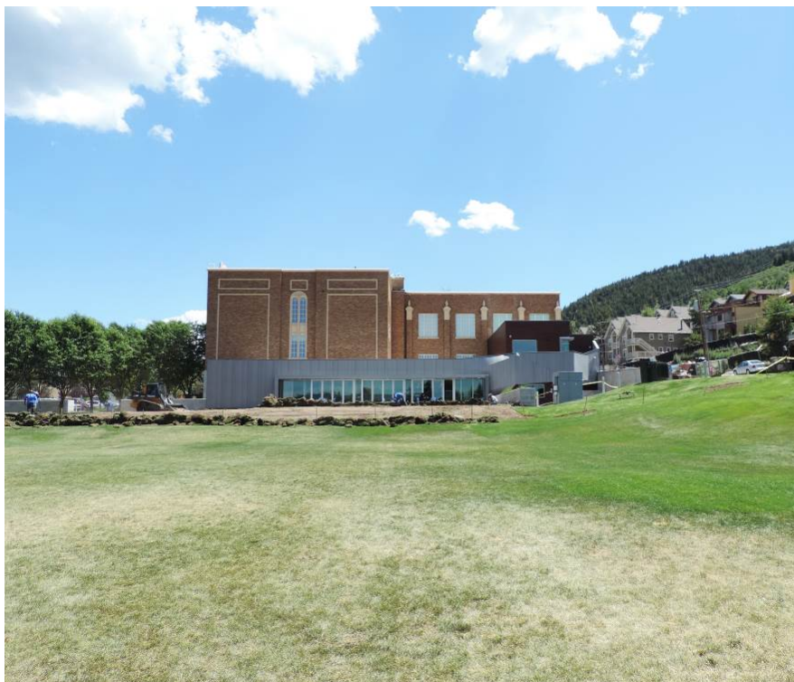
Photo 8 of 22: North elevation. Camera facing south.
