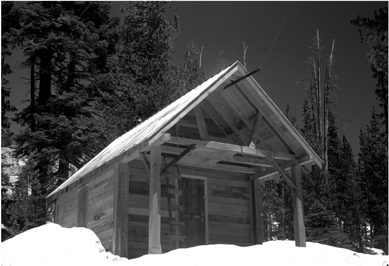
Historic Photo #1. Snow Flat Snow Survey Shelter, 1949. Southwest corner (west and south elevations), camera facing roughly northeast. Photographer: unknown.
