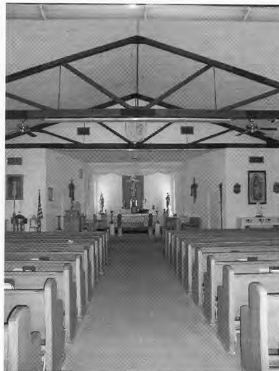
Photo 14. Interior of Our Lady of Lourdes Catholic Church. View towards altar showing trusses and oak pews.
