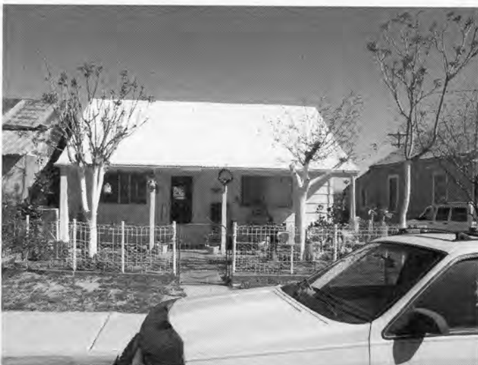
Photo 11. 387 E. Fifth Street. A second generation "railroad house" built in 1925. This is a side-gabled linear-plan type with shed additions to the rear.
