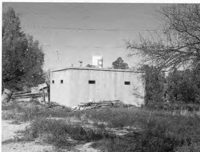
Photo 15. The Old Jail House. Built in 1915, it is located on what was for many years the Mejia property. Constructed of concrete, it has a trapezoidal plan and an overhanging, slightly gabled, concrete roof.
