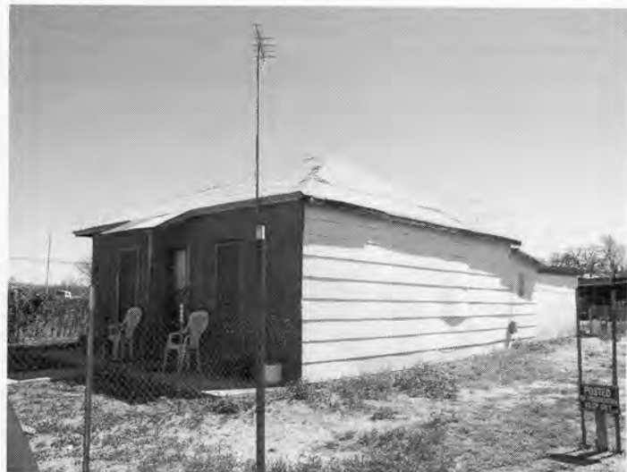
Photo 10. 550 E. Fifth Street. This is a classic pyramidal cottage built in 1930 of stuccoed adobe. The west wall has blue, horizontal, composition siding.
