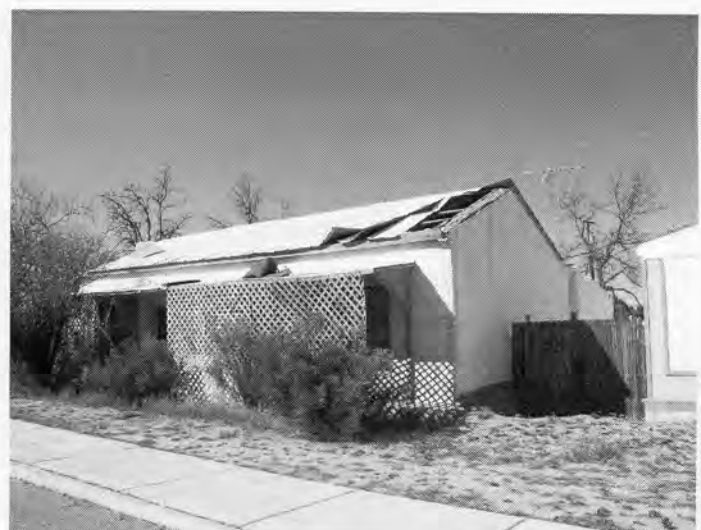
Photo 12. 463 E. 5 th Street. The 1900 Genaro Figueroa house was originally a Sonoran, parapet-walled, flat-roofed dwelling. It was later transformed by the addition of a pitched roof, exemplifying the "transitional" tradition.
