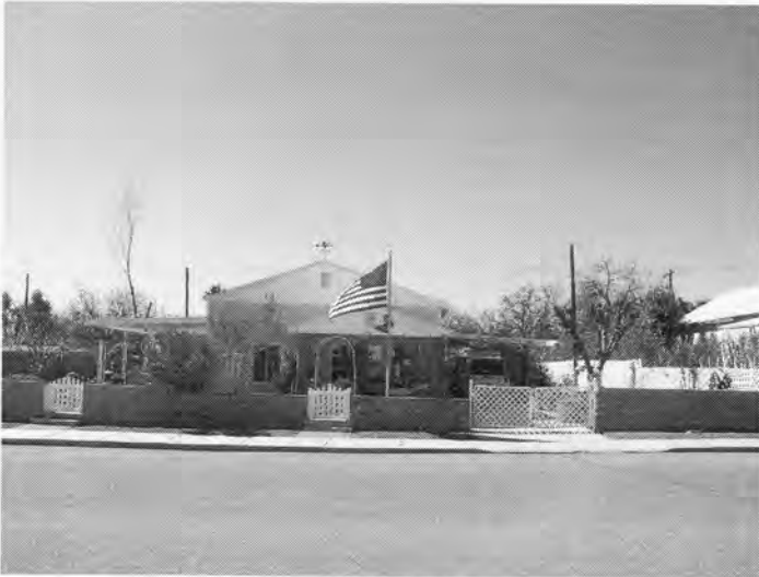
Photo 9. 418 E. Fifth Street, the Ellsworth House. This gable-front, massed-plan dwelling acquired its current form and front porch through a 1950s remodel of the original ca. 1900 adobe walls. The siding is painted a vibrant mint green color.
