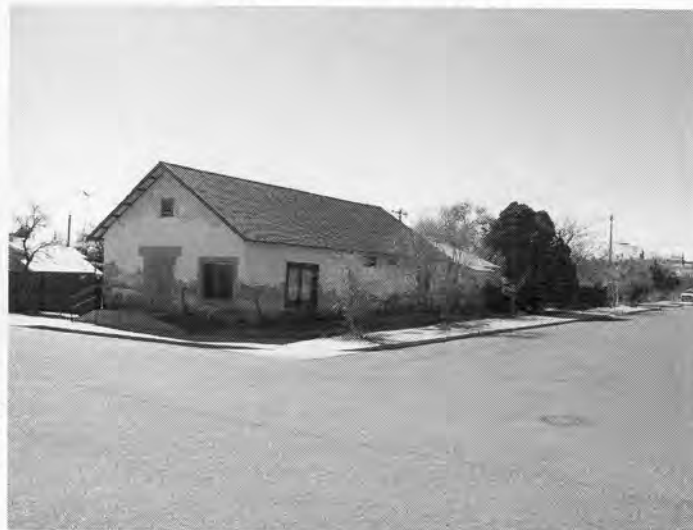
Photo 16. Original Quihuiz Grocery Store, built in 1925. Owned and operated by the Quihuiz family who resided in back. Unusual for a corner commercial building is its elongated, gabled form.
