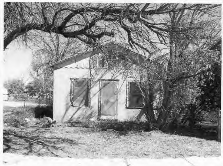
Photo 8. 419 E. Fifth Street. A second-generation, front-gabled, tan colored, stuccoed dwelling built in 1928 by Joaquin and Ana Figueroa Meza. The dwelling has only two rooms.
