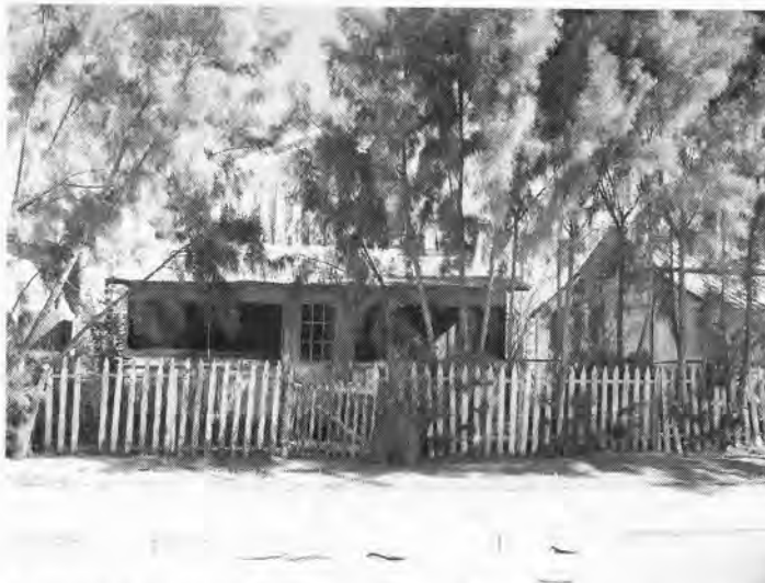
Photo 7. 369 E. Fifth Street. A 1900 "railroad house" west of Gila Street. This is a gable-front, massed-plan dwelling, a Euroamerican vernacular type. Built of frame, it may be an example of "box construction."
