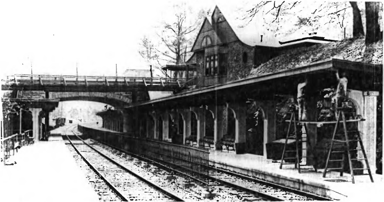
The Montclair Branch is photogenic in only one location along its four miles — at Glen Ridge where the track hugs Toney's Brook. It was also probably the reason why the line was single track until 1912. There wasn't enough room between the stream and the hillside. For double tracking, the hill was cut back. In this picture, taken in March 1913, painters are at work on the wood canopy. A temporary walkway over the tracks is still in place.
