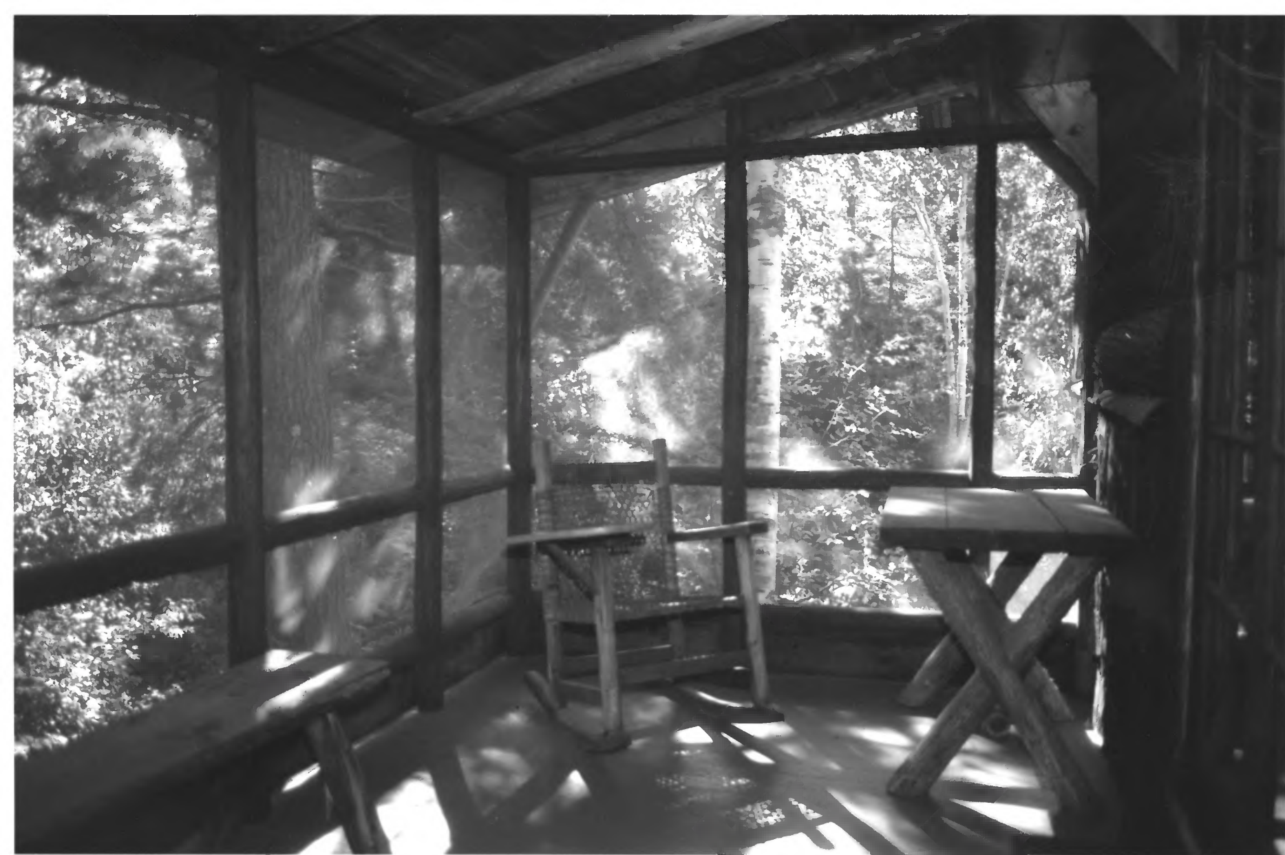
Ernest C. Oberholtzer Rainy Lake Islands Historic District Big House #8 (Porch) Koochiching Co., Mn 013066-17
