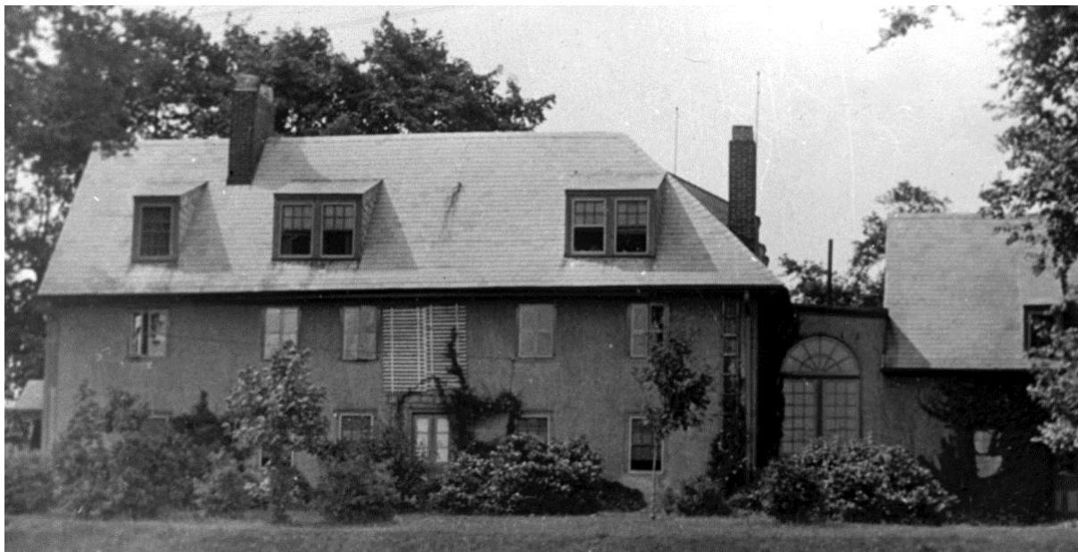
Figure 32: View of the south (main) façade of Sellers Hall, c.1936, showing combination of double-hung windows on first story and casement on second, front door modified to set of two doors, stucco added to exterior stone walls, breezeway modified and dormer added to outbuilding (see Photo 1 for current appearance). Courtesy of Upper Darby Historical Society.
