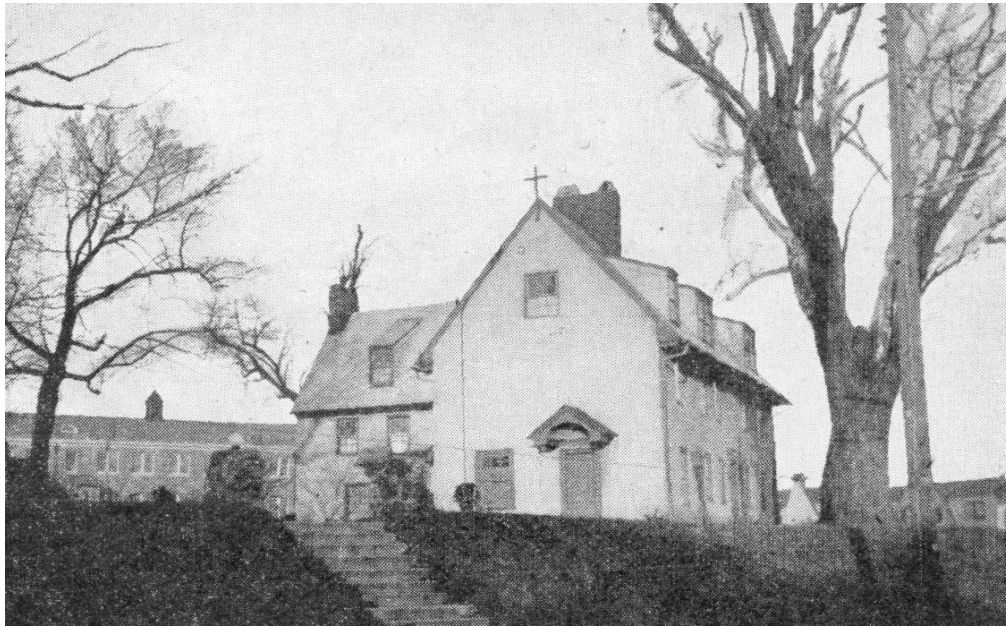
Figure 30: View of the west elevation of Sellers Hall, in use as the chapel and rectory for St. Alice Parish, c.1923. Two dormers on south elevation have been modified to double-wide, pent roof was added over door on west elevation, and paneled shutters have been removed (see Photos 1, 6 and 7 for current appearance). Courtesy of Upper Darby Historical Society.
