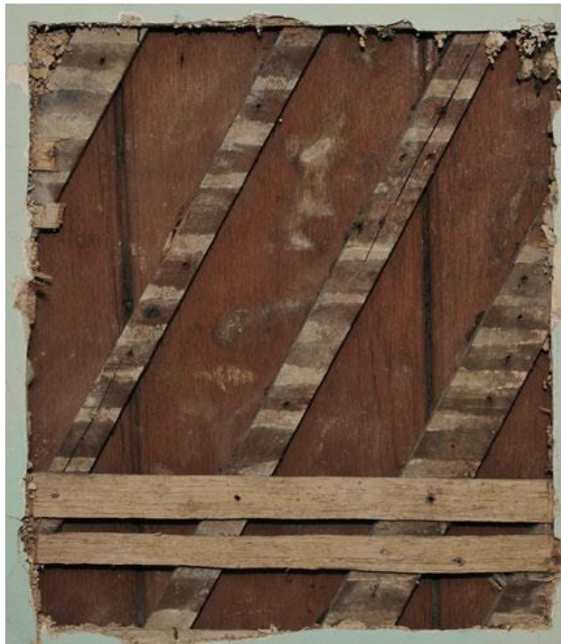
Photo 10: Original wood board partition on second floor (University of Pennsylvania, 2010).
