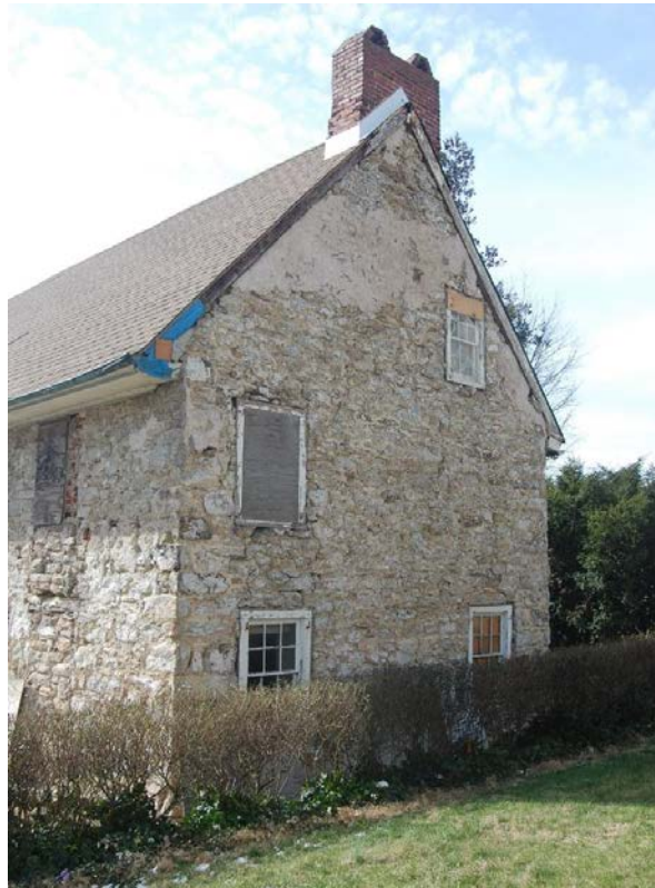
Photo 4: View facing southwest towards the north elevation of the addition.
