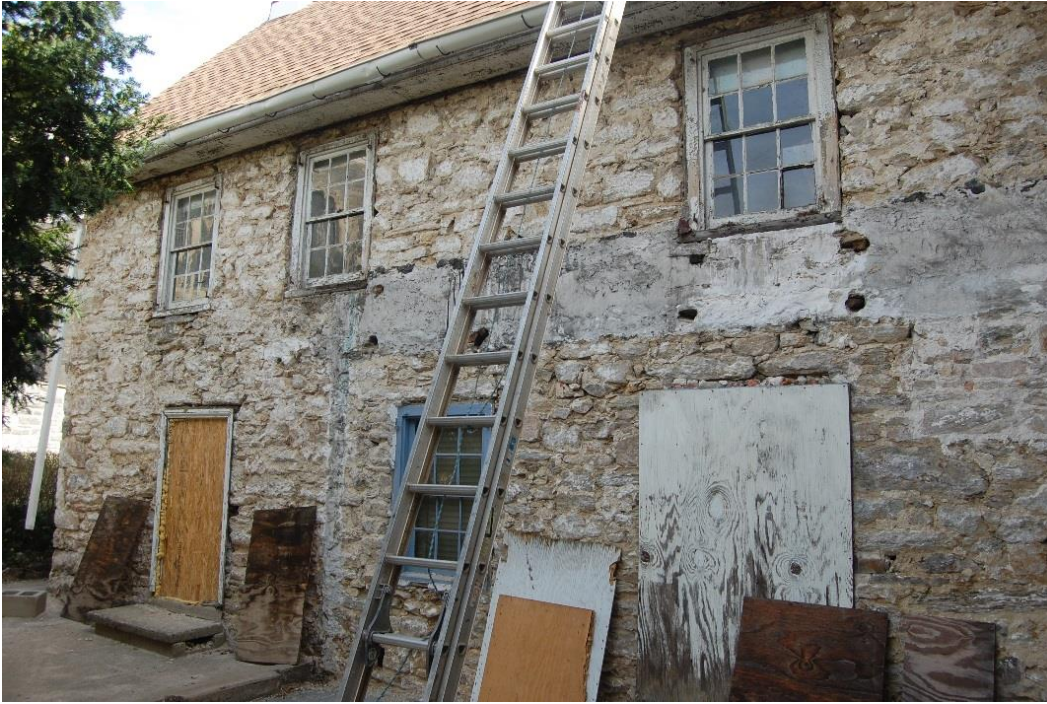
Photo 7: View facing northeast towards the west elevation of the addition.
