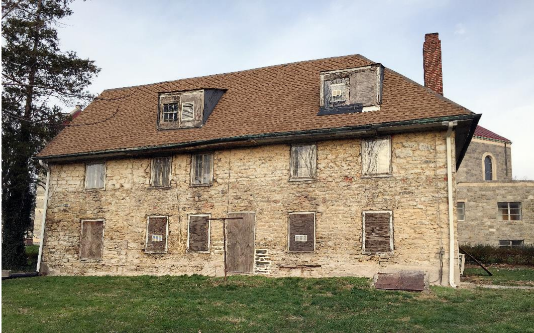
Photo 1: View facing northwest towards the south (main) façade. Church is visible on north side of Sellers Hall.
