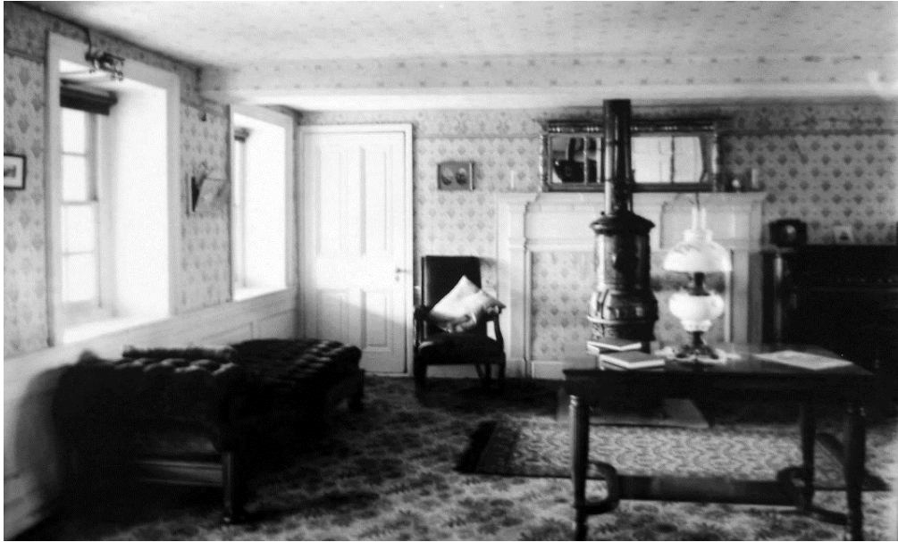
Figure 22: Room 102, facing west, c.1906.
