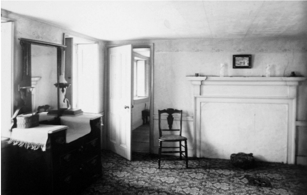
Figure 24: Room on south side of second floor, facing west, c.1906.
