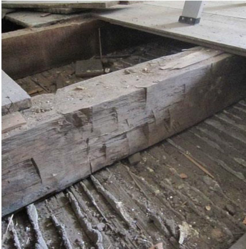
Photo 16: Hand hewn joist in Room 302 (University of Pennsylvania, 2010).
