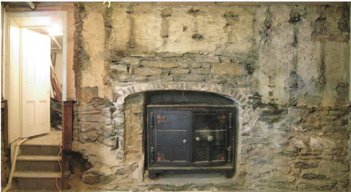
Photo 14: Fireplace on west wall of Room 102 showing brick arch of firebox and north cove (University of Pennsylvania, 2011).
