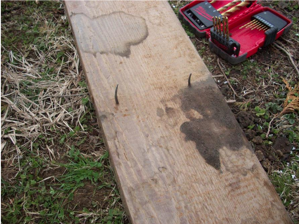
Photo 13: Interior side of soffit board from south elevation with hand-planed wood and hand-wrought nails (University of Pennsylvania, 2011).
