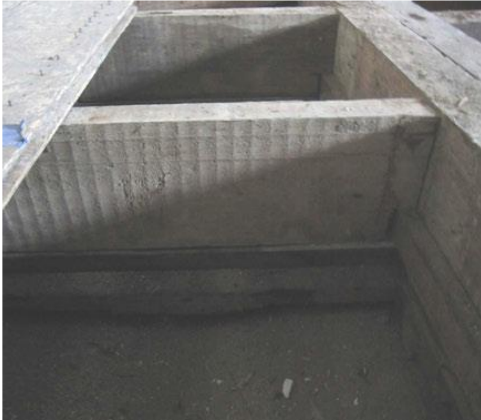
Photo 17: Vertical sawmill marks on floor joists (University of Pennsylvania, 2010).
