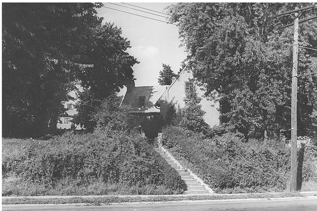
Figure 33: View of the west façade of Sellers Hall from Walnut Street in 1946. Currently, the view from Walnut Street is obscured by heavy vegetation. Courtesy of Upper Darby Historical Society.
