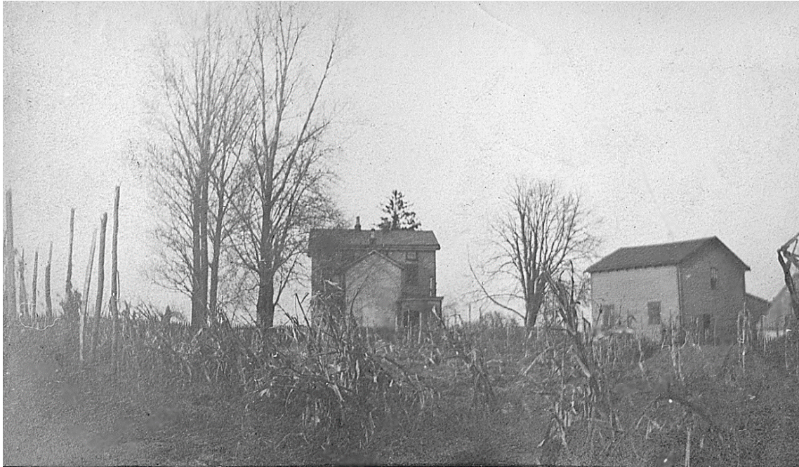
Figure 18: Tenant houses at Sellers Hall Farm, later renamed Elim Farm, c.1906. All associated farm and tenant resources believed no longer extant. Courtesy of Upper Darby Historical Society.
