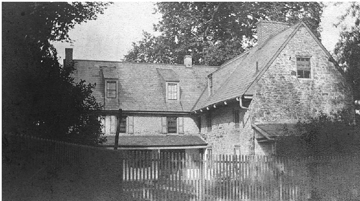
Figure 15: View of west elevation of Sellers Hall in 1902, with exposed stone façade, pent roof/porch on north section of west elevation, shed dormers and paneled shutters on the first and second-story windows (see Photos 6 and 7 for current appearance). Courtesy of Upper Darby Historical Society.
