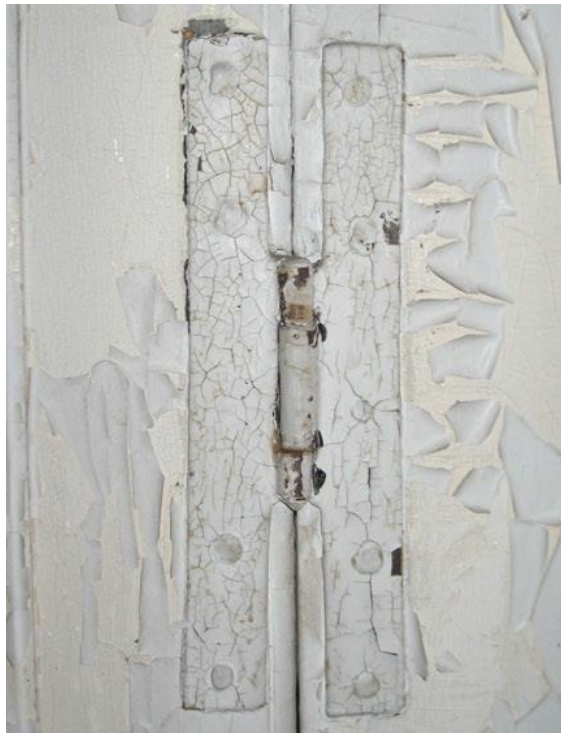
Photo 12: H-hinge on third floor board door, likely dating to the early 18th century (University of Pennsylvania, 2011).
