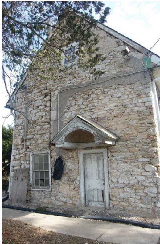
Photo 6: View facing northeast towards the west elevation of the original building.
