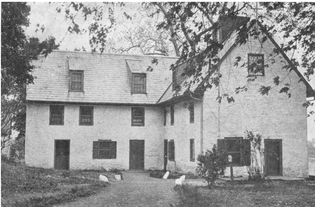
Figure 28: View of west elevation in 1922. Wrap-around porch and pent roof/porch on north section of west elevation have been removed, and a cross has been added on the west gable (see Photos 6 and 7 for current appearance). Courtesy of Upper Darby Historical Society.
