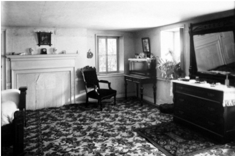
Figure 25: Southeast corner of second floor, c.1906.
