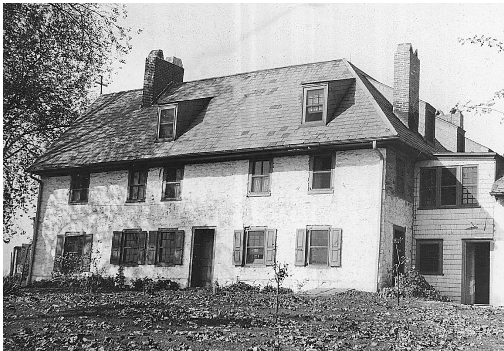
Figure 29: View of the south (main) façade of Sellers Hall, ca. 1923. Chimneys have been modified and the connection/breezeway to outbuilding is visible (see Photo 1 for current appearance). Courtesy of Upper Darby Historical Society.
