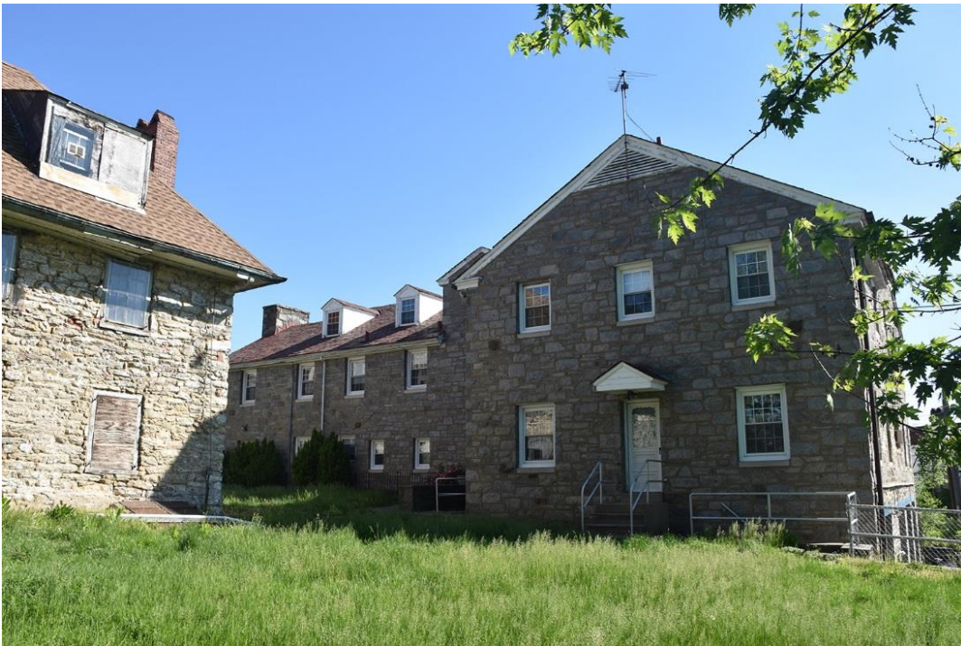
Photo 2: View of southeast corner of Sellers Hall, facing Rectory on east side.
