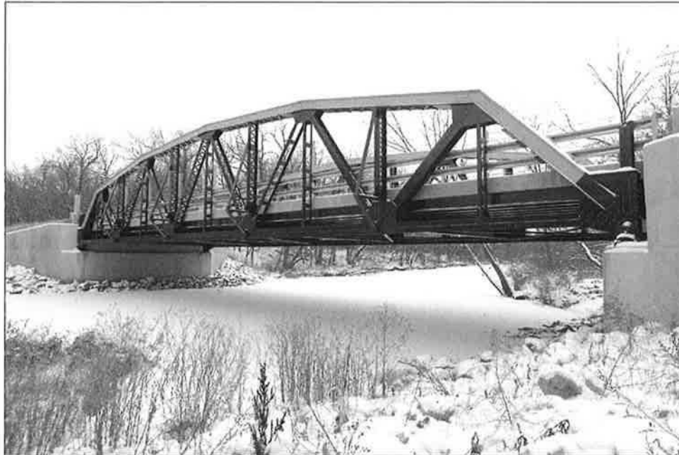
Photo #2: General view north elevation, looking southeast.
