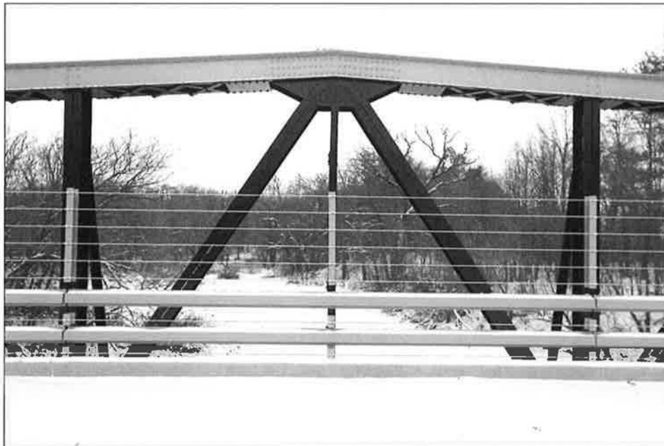
Photo #5: Oblique view of south truss, showing outrigger system, looking east.
