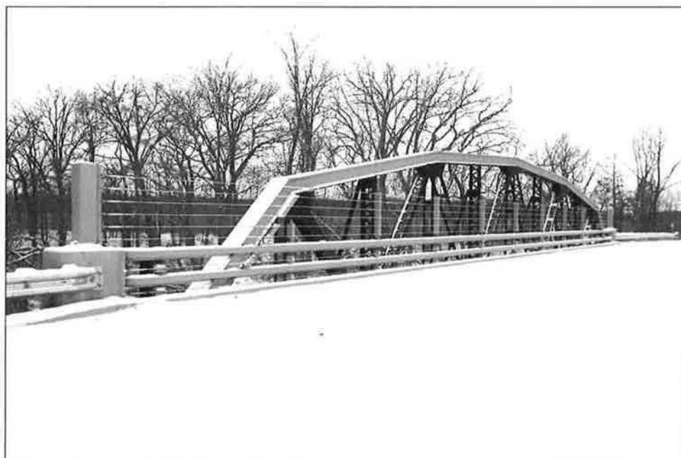
Photo #3: Oblique view of north truss, looking east.
