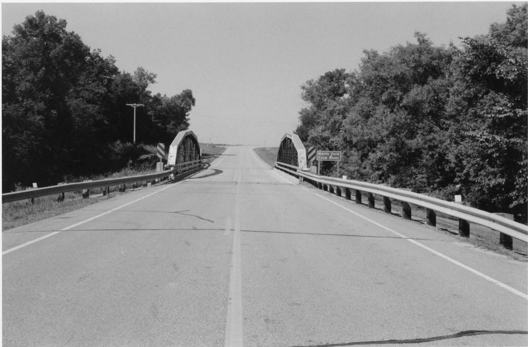
Bridge no. 5388 Mn Highway 24 over North Fork Crow River, Forest City Township Meeker Co., Mn 013059-4
