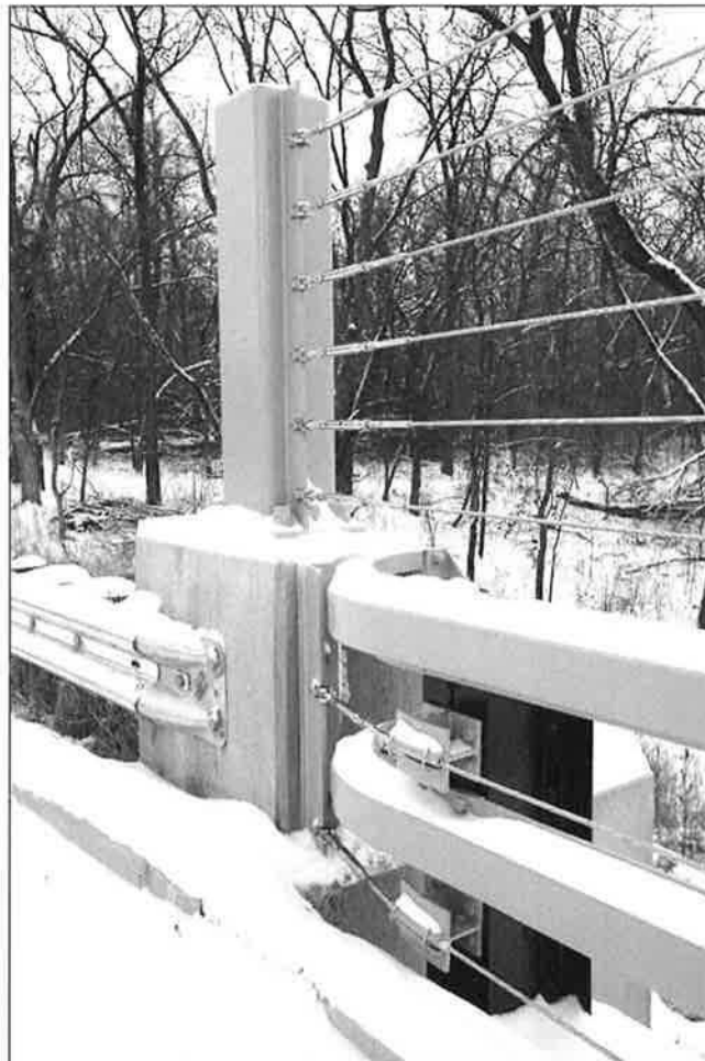
Photo #9: Oblique view of southeast concrete post showing wire railing system, looking southeast.
