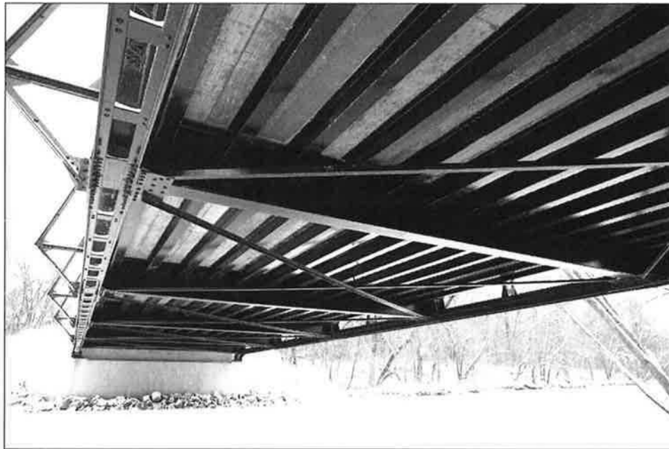
Photo #6: Oblique view of new deck system, looking east-southeast.
