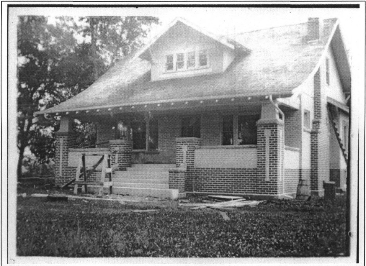
Gustav and Annie Swanson Farmhouse Under Construction - 1918
