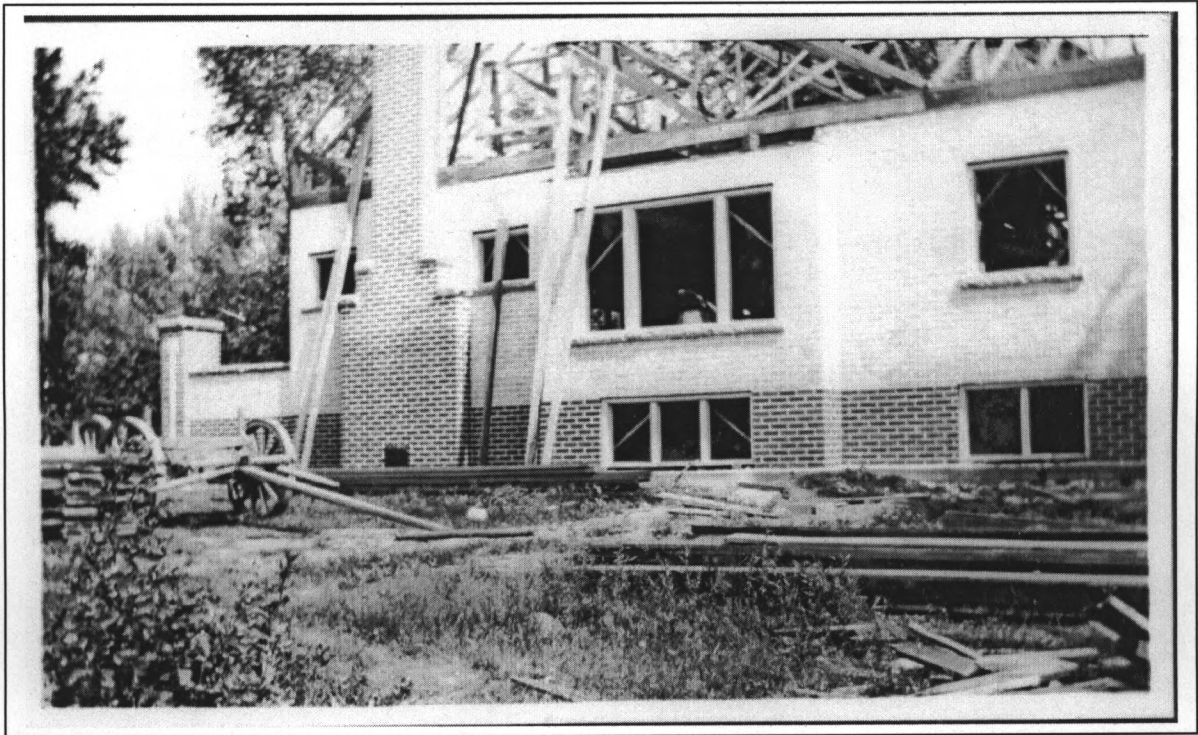
Swanson Farmhouse Under Construction - 1918
