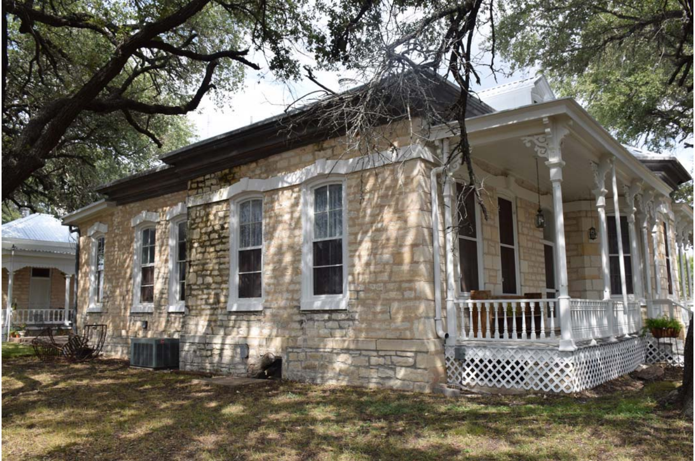
Photo 2 Main house, west oblique Camera facing northeast
