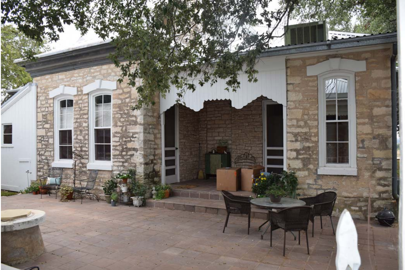
Photo 3 Main house, north oblique Camera facing south/southeast
