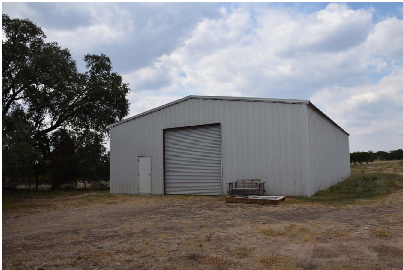
Photo 12 Metal storage barn (noncontributing) Camera facing north
