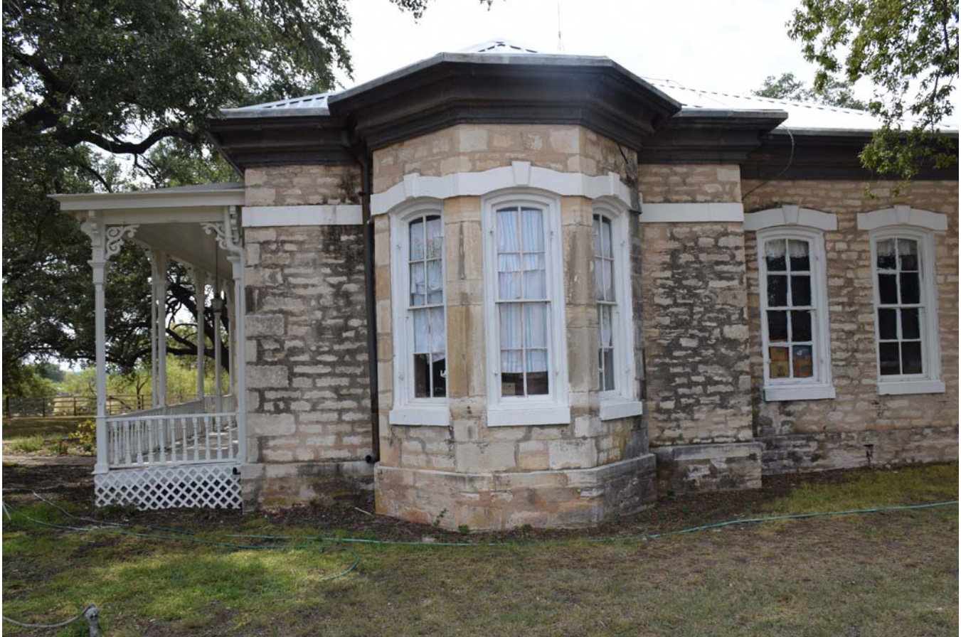
Photo 4 Main house, east elevation Camera facing west
