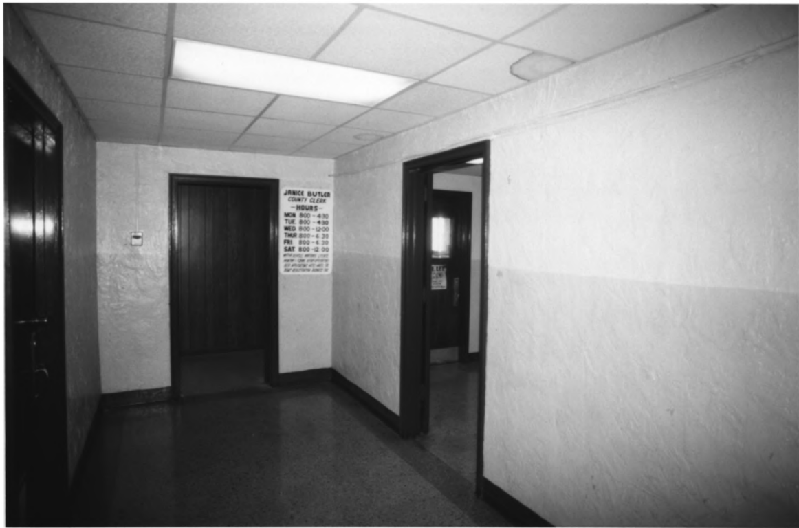
Cooke County Courthouse Cooke County, TN
