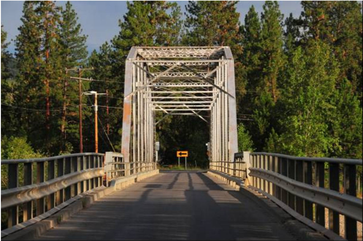
Photo MT_MissoulaCounty_MaclayBridge_0008 (8 of 9) - Maclay Bridge: view to the northwest across the bridge deck.
