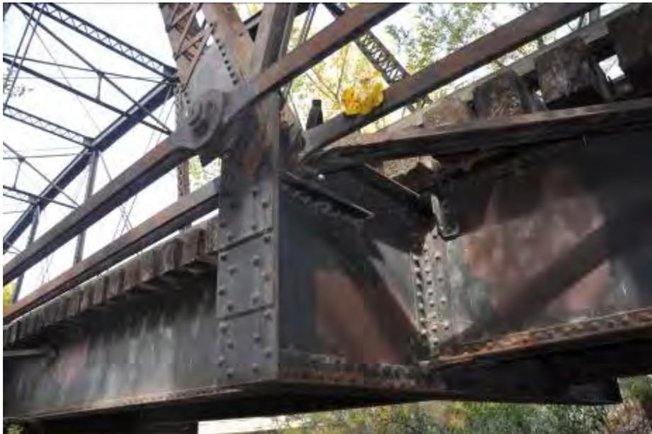
Photo 7 of 9. Eyebar Connection. Camera facing northwest.
