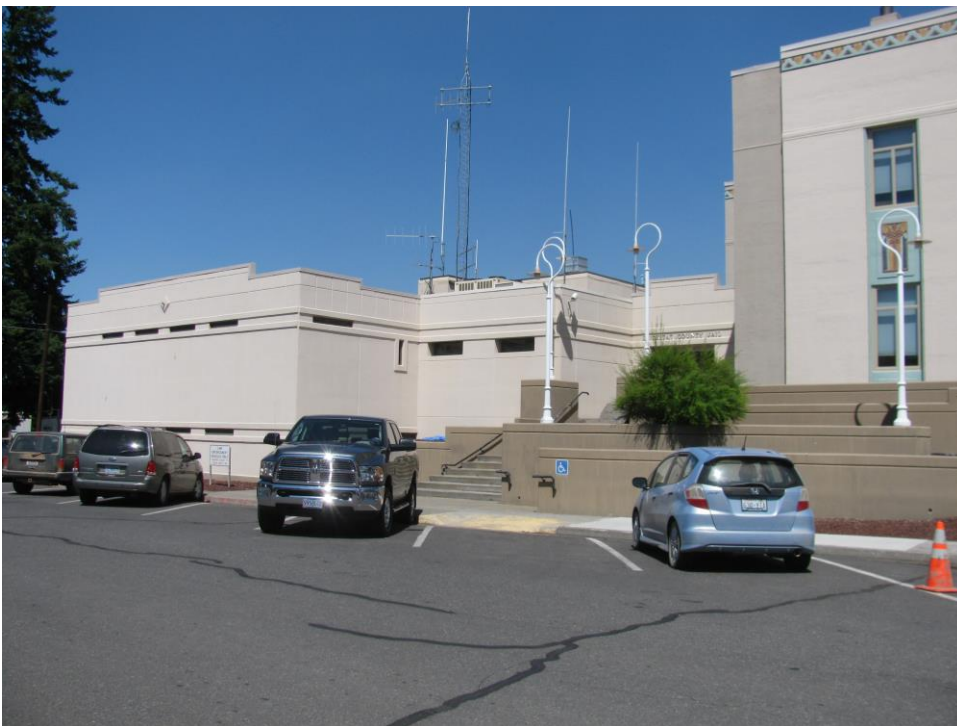
7 of 15: South elevation of Jail annex showing connection to main courthouse.
