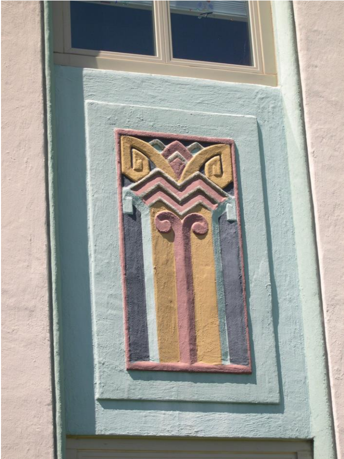
8 of 15: Detail of Spandrel Panels.
