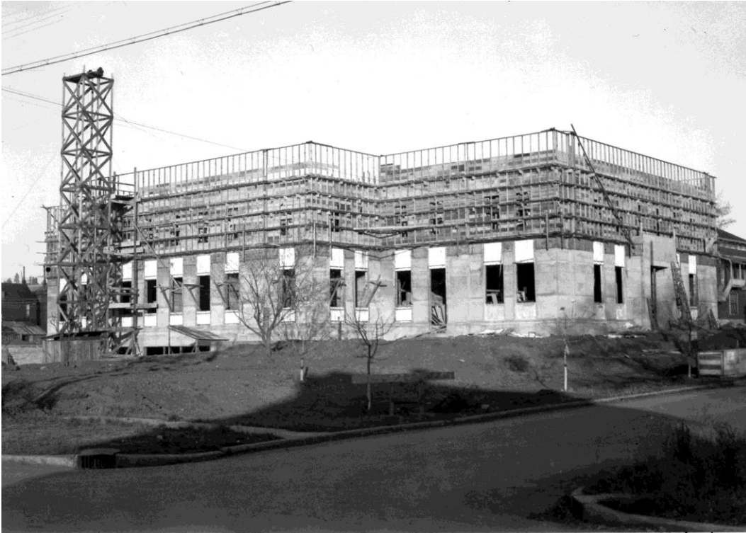
Figure 12: Courthouse southwest corner during construction 1941.
