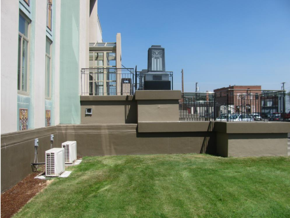
2 of 15: South elevation of entry steps.
