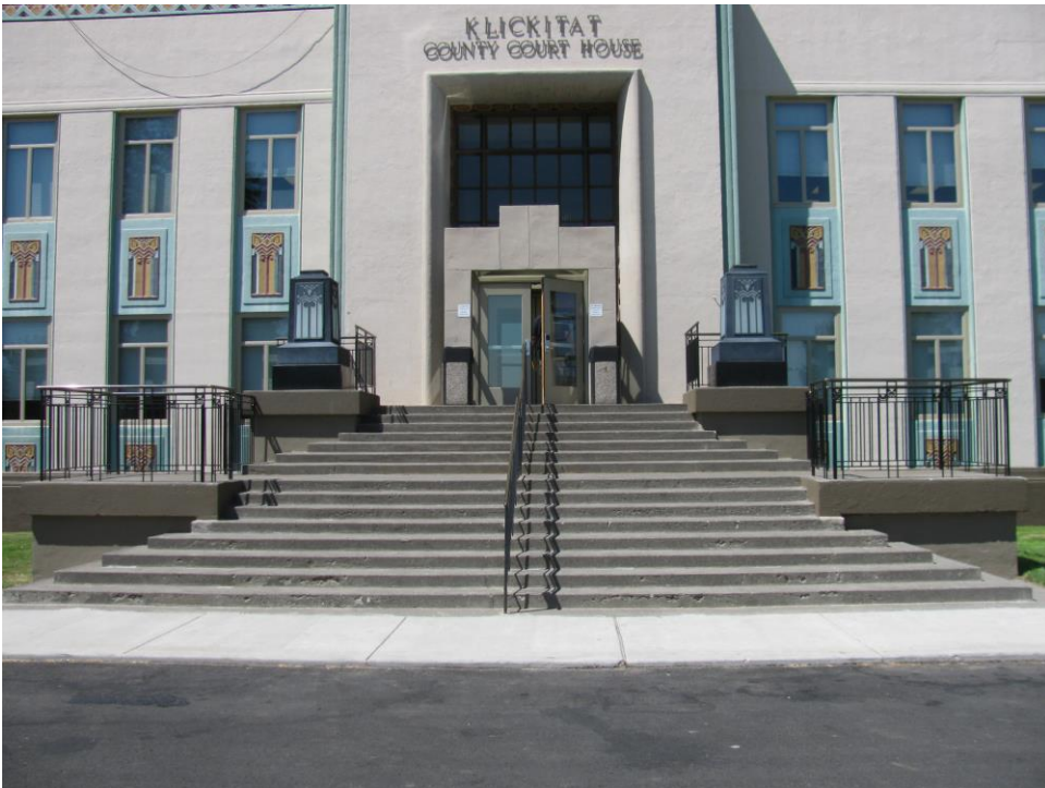
3 of 15: Detail of entry steps.
