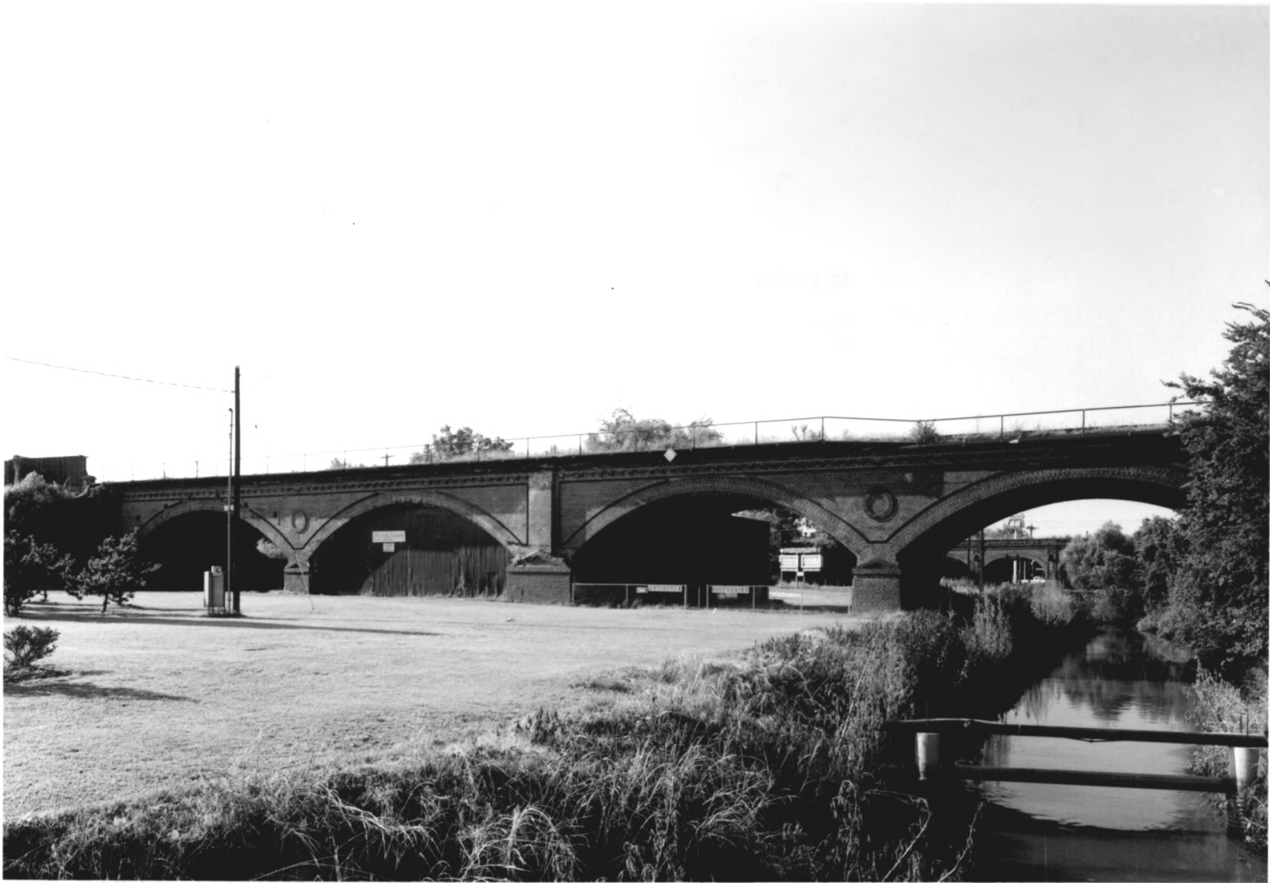
Central of Georgia RR: Dooley Yard Viaduct (1860), Savannah, GA.
