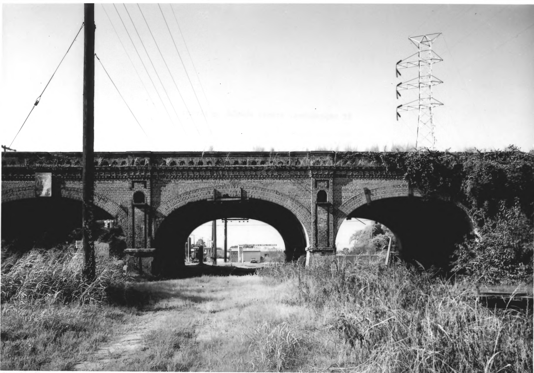
Central of Georgia RR: Main Line Viaduct (1853), Savannah, GA.
