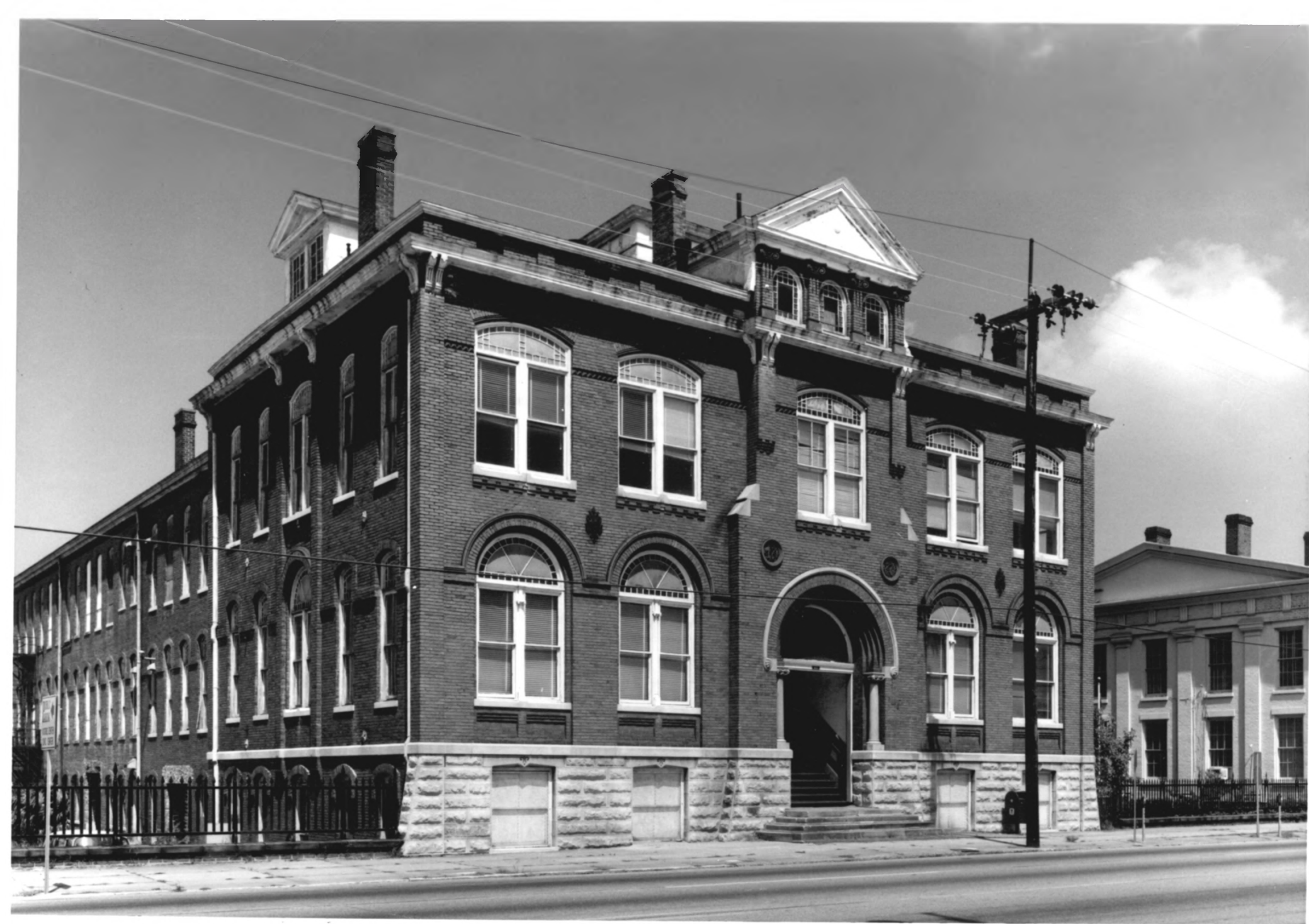
Central of Georgia RR: Red Building (1887), Savannah, GA.
