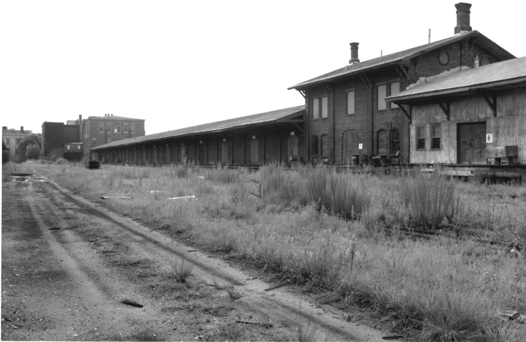
Central of Georgia RR: Down (Produce) Freight Warehouse (1859), Savannah, GA.
