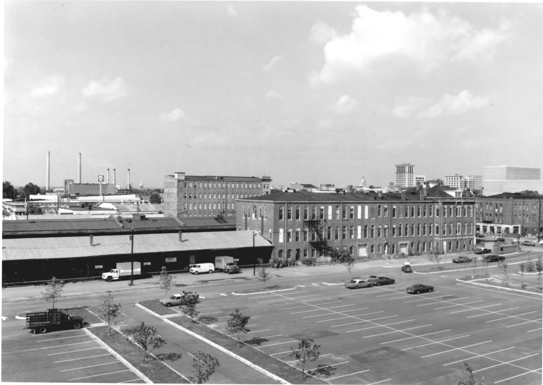
Central of Georgia RR: South Elevation of Red Building showing 1910 addition and Down Freight Warehouse (1859).
