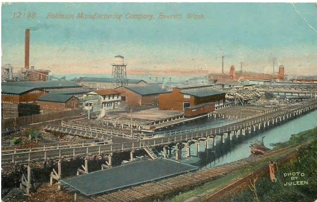
Robinson Manufacturing Co. Plant – Everett – c. 1915
