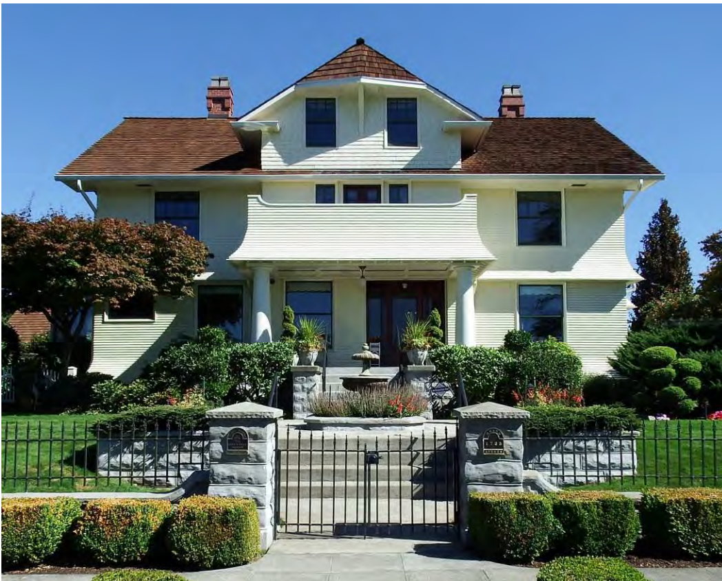
3 of 11. Main/West facade
