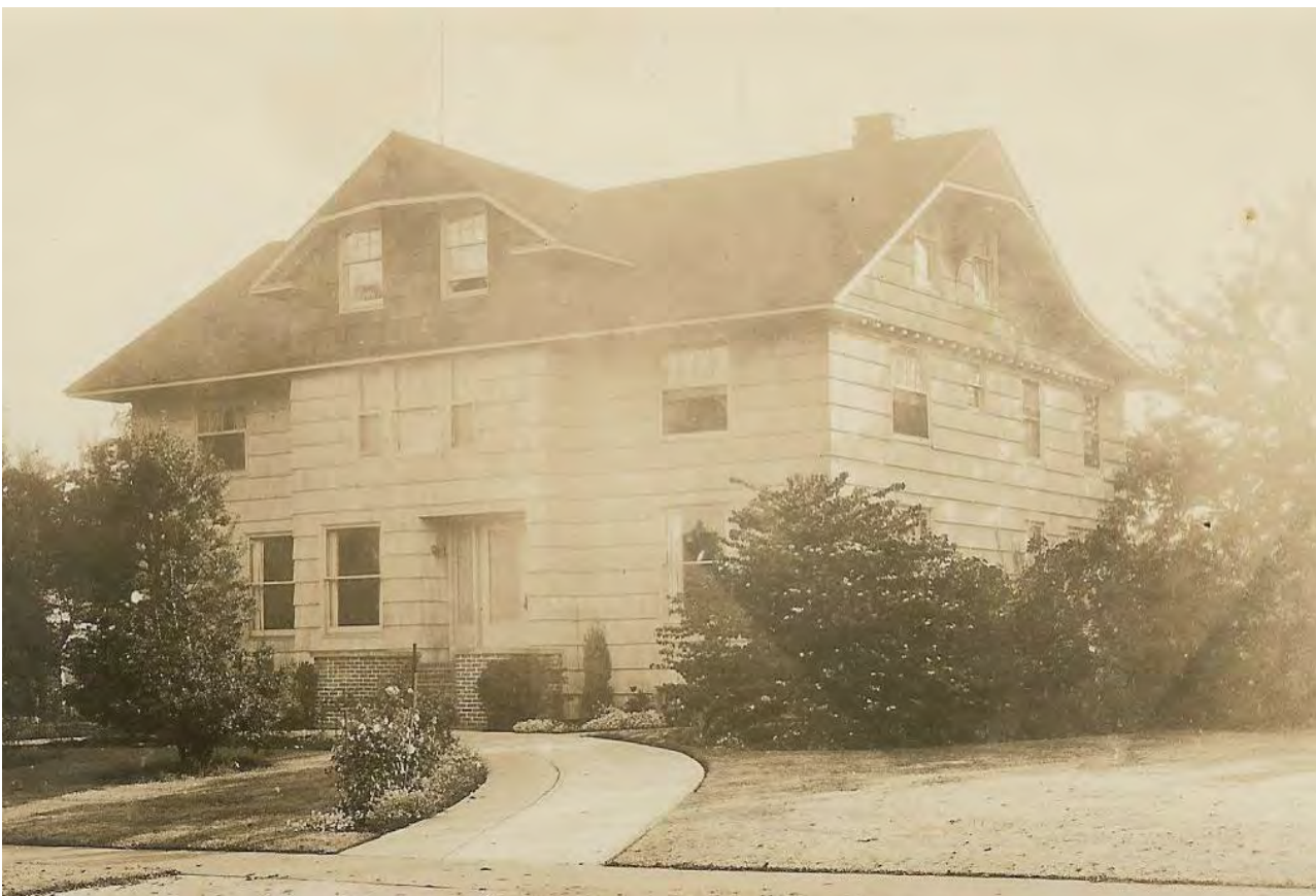
Result of remodeling by Knowles Family – c. 1932
