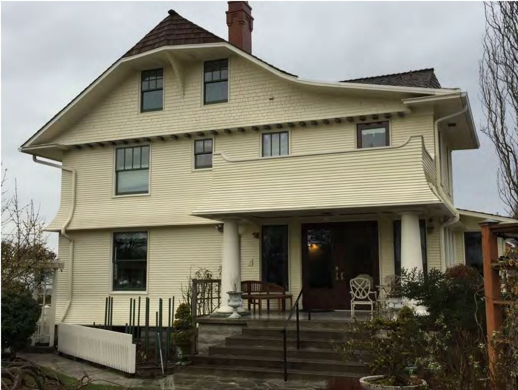
4 of 11. South facade
