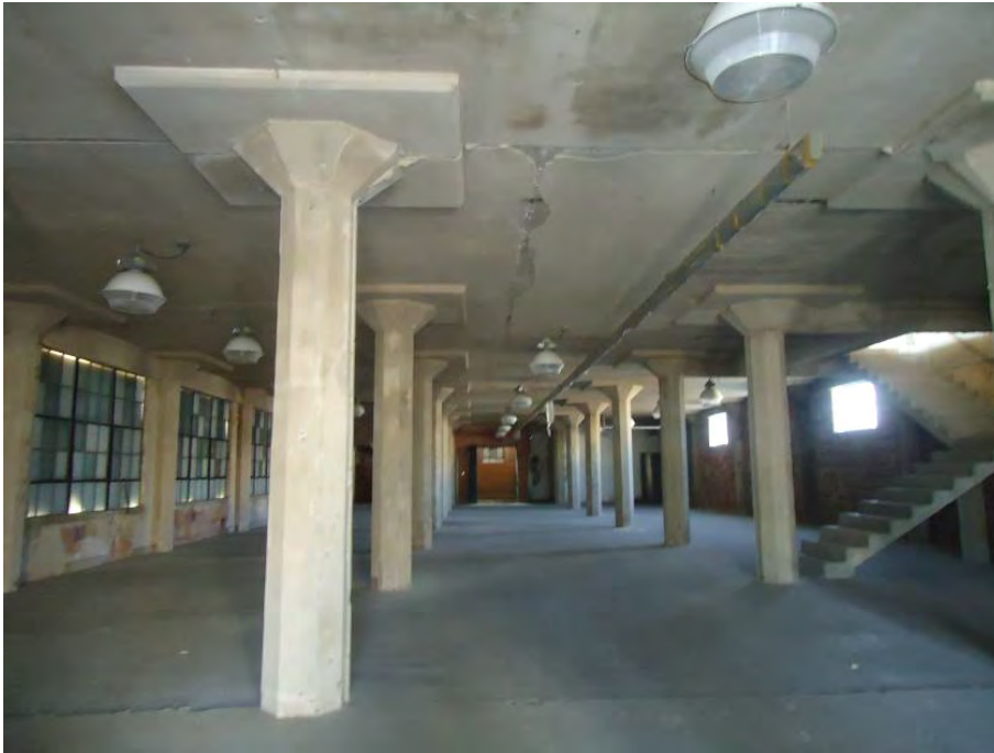
Interior, first floor, camera facing south
