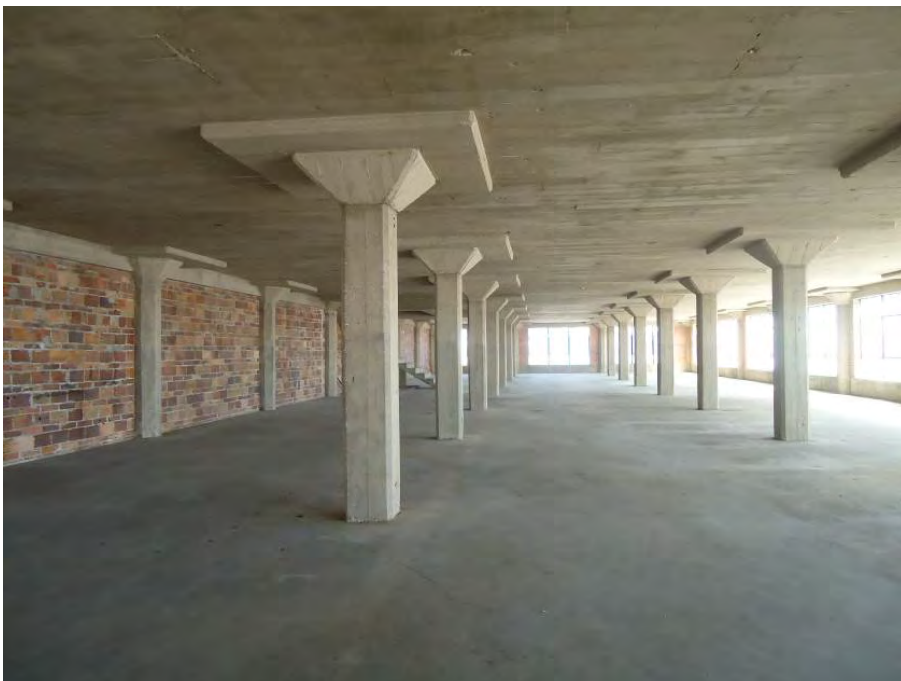
Interior, third floor, camera facing north
