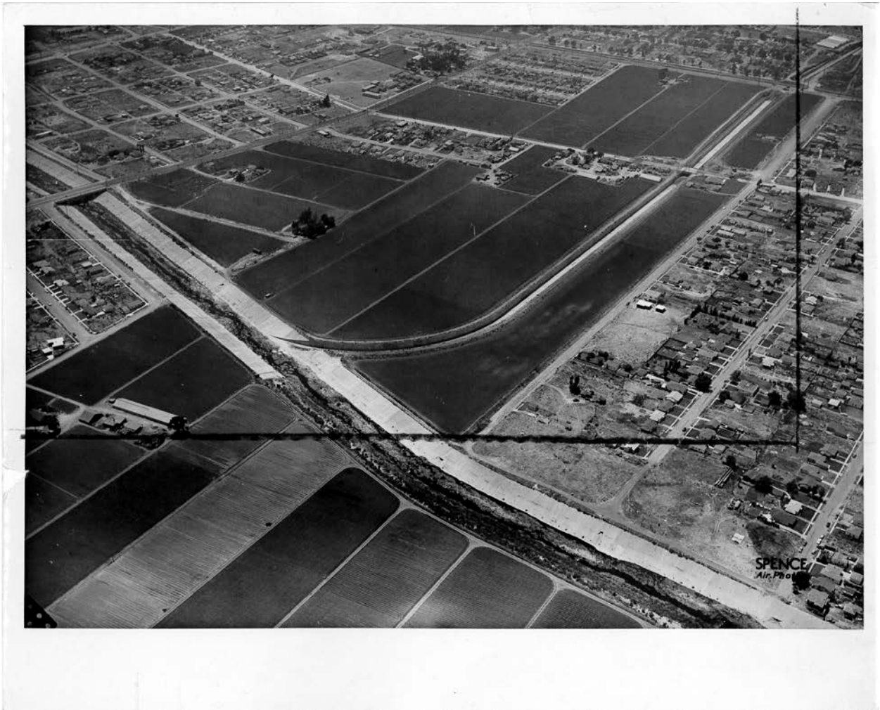
Figure 1: Aerial view of Mar Vista Gardens Site prior to construction. Undated. Courtesy of HACLA.
