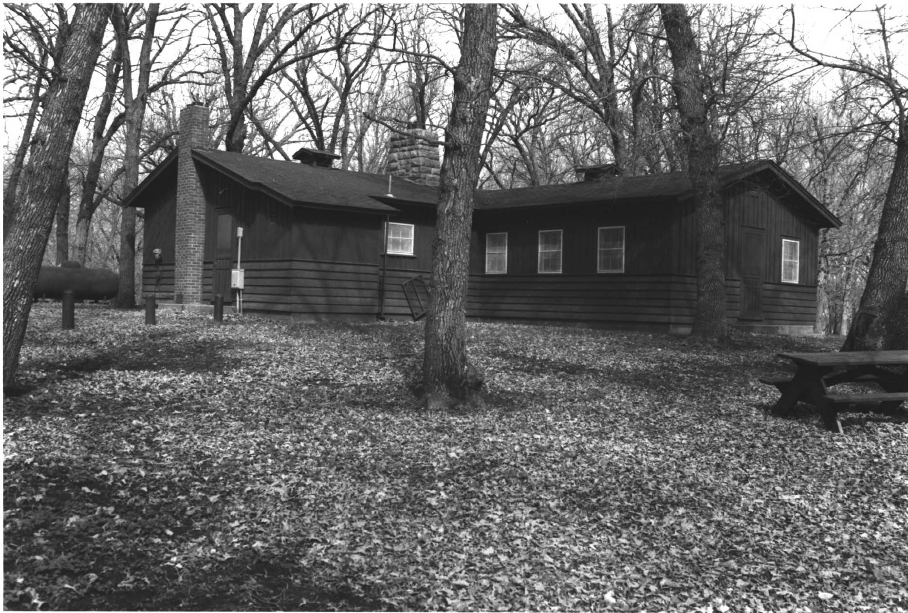
LAKE SHETEK STATE PARK WPA/RUSTIC STYLE GROUP CAMP MURRAY AND SHETEK TOWNSHIPS, MURRAY COUNTY, MINNESOTA #09721-12 BUILDING #1
