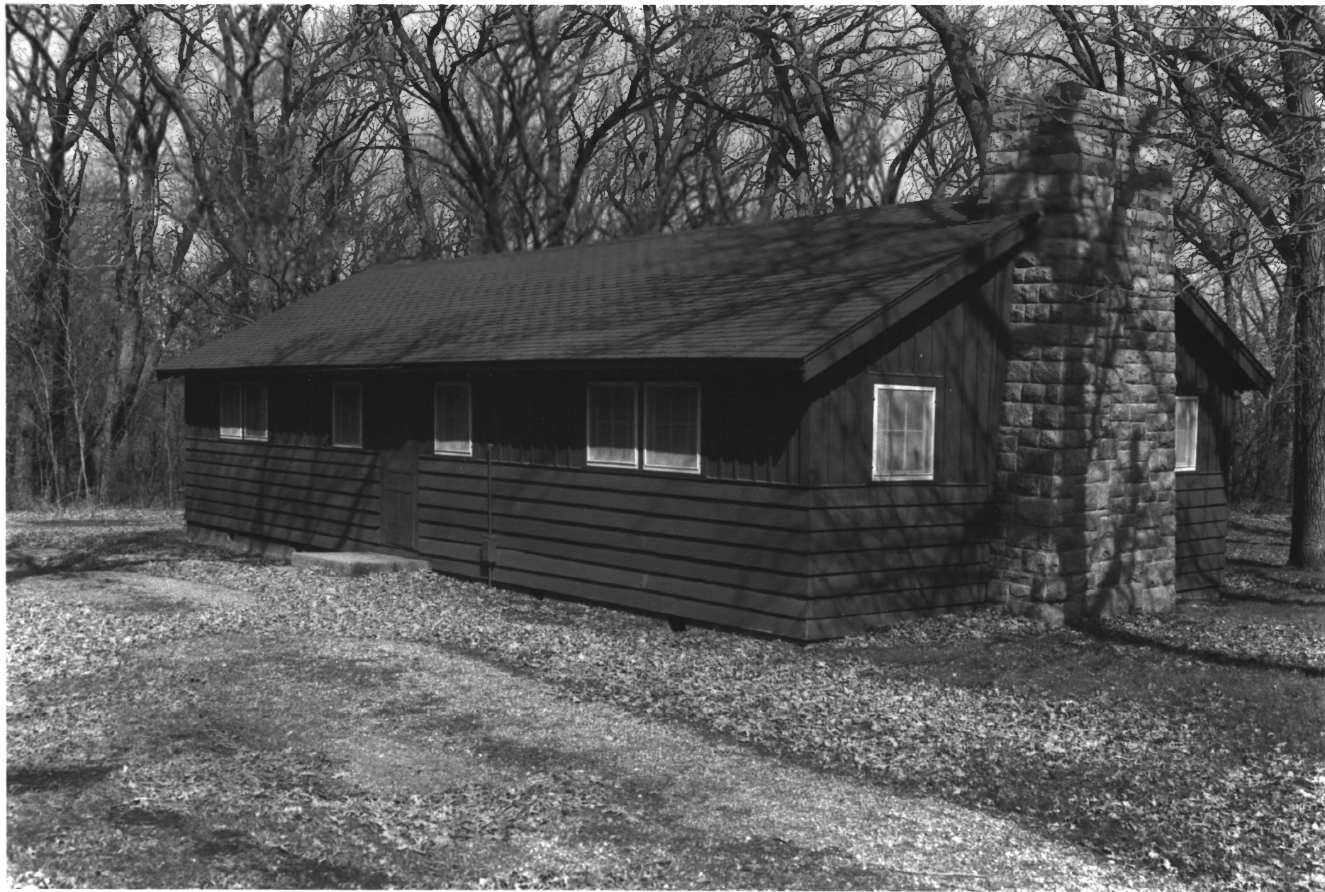
LAKE SHETEK STATE PARK WPA/RUSTIC STYLE GROUP CAMP MURRAY AND SHETEK TOWNSHIPS, MURRAY COUNTY, MINNESOTA #09721-9 BUILDING #2
