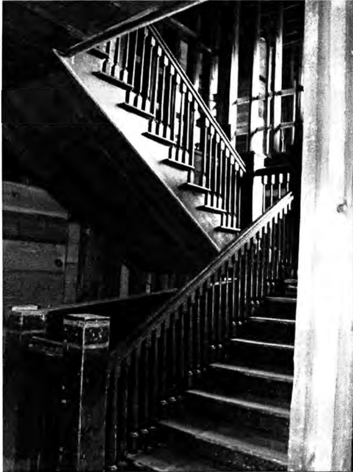
Grand staircase leading from 2 nd to the 3 rd floor of Coram Hotel (Hotel Libby). June 2011.
