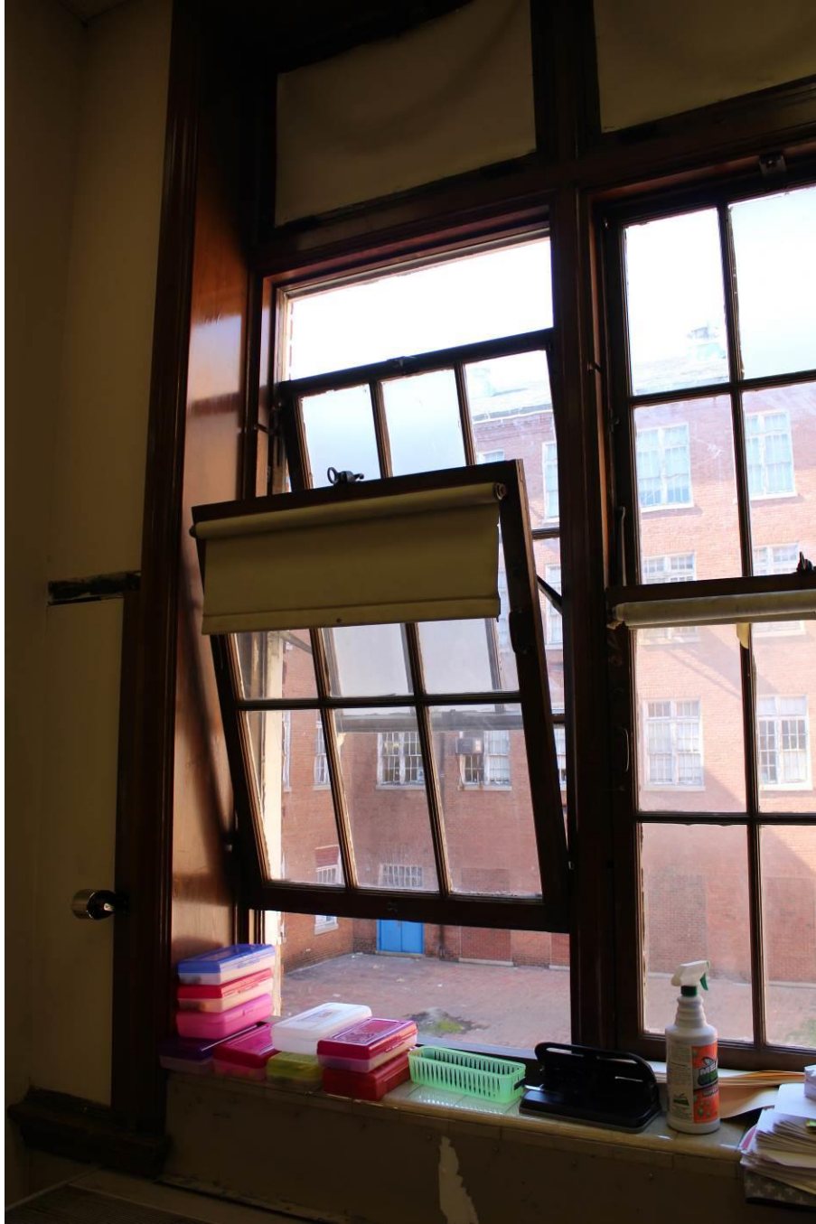
Photo 14: DC_Roosevelt Senior High School_0014.tif Austral-type Wood Windows
