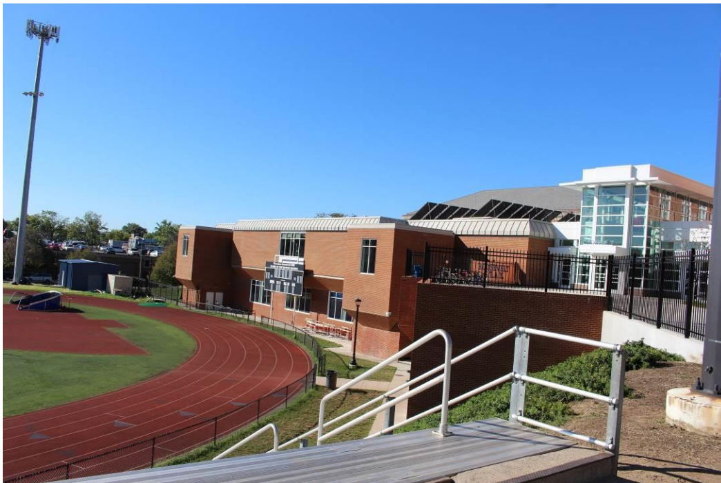
Photo 11: DC_Roosevelt Senior High School_0011.tif 1970 addition on Gymnasium Pavilion, Looking Southwest
