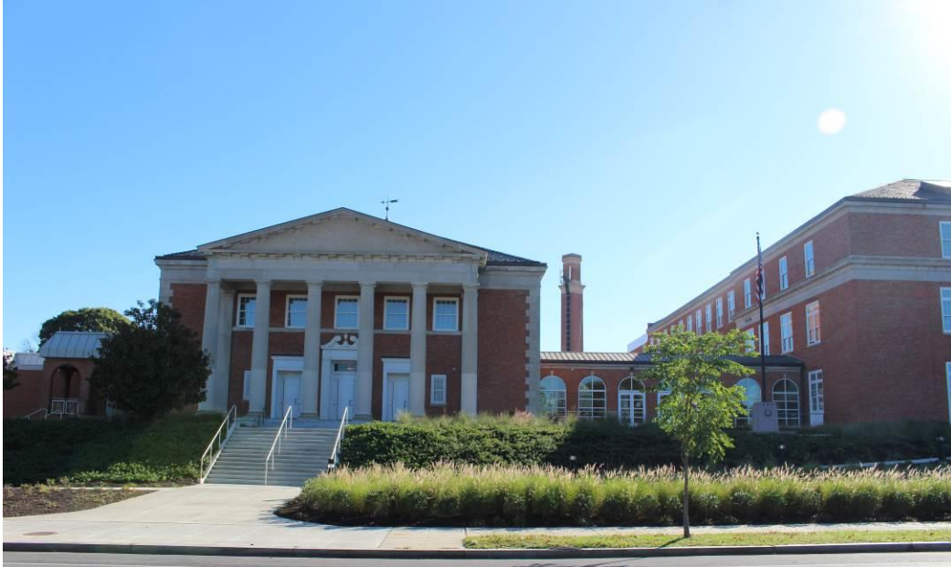
Photo 12: DC_Roosevelt Senior High School_0012.tif Auditorium Pavilion and Hyphen, West Elevation, Looking East
