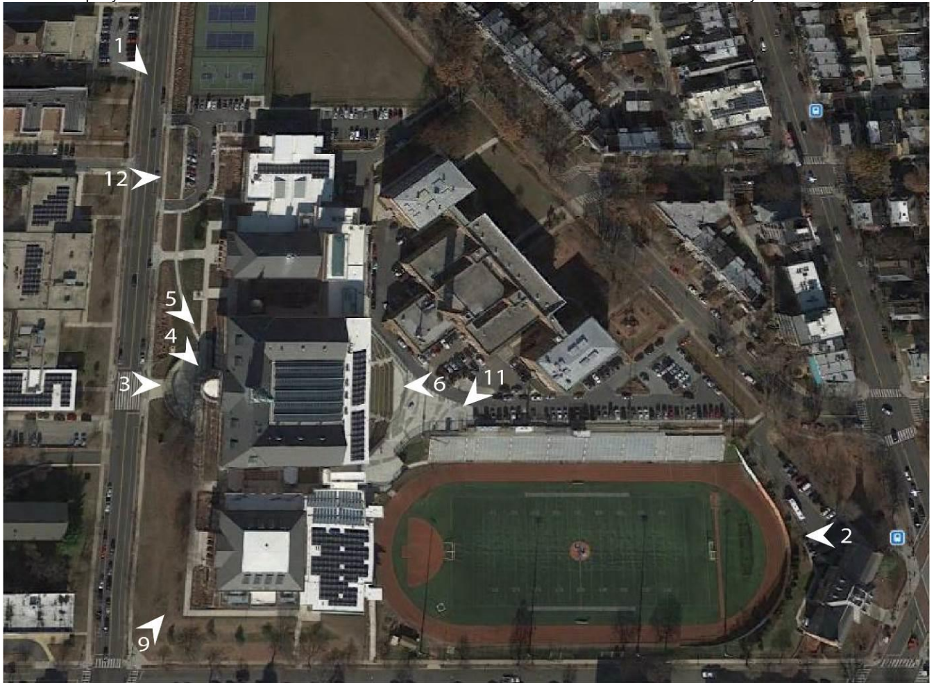
Aerial Illustrating Exterior Photo Locations
