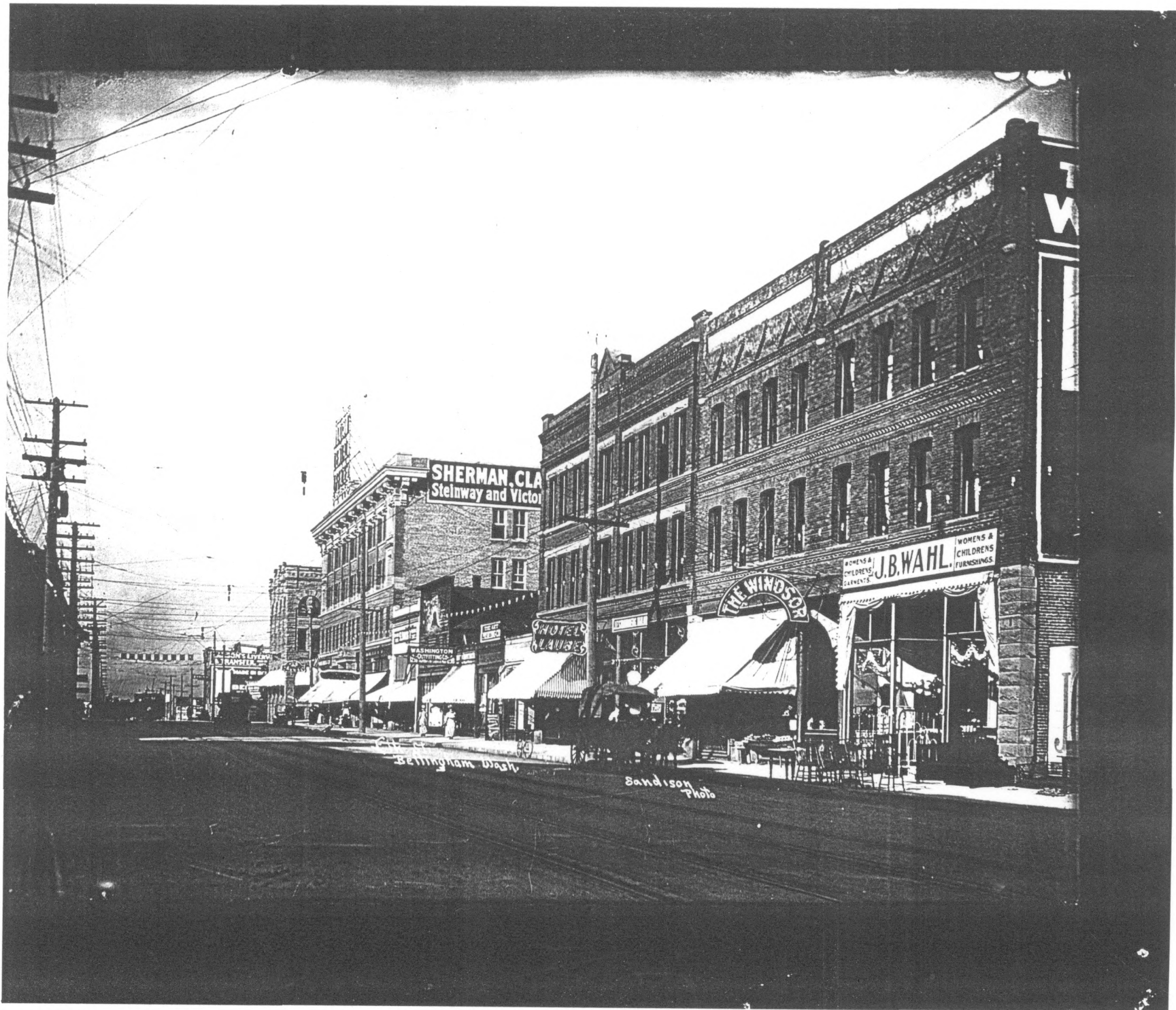
3. VIEW LOOKING N ON ELK STREET WITH HOTEL'S LAUREL; WINDSOR IN FOREGROUND, 1908.
