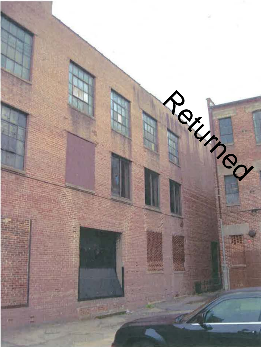
MD_BaltimoreCity_UnionBrosFurnitureCo_0003.tif Building Exterior – Clarkson St. (West) Elev. – Bldg. 1 3 of 27
