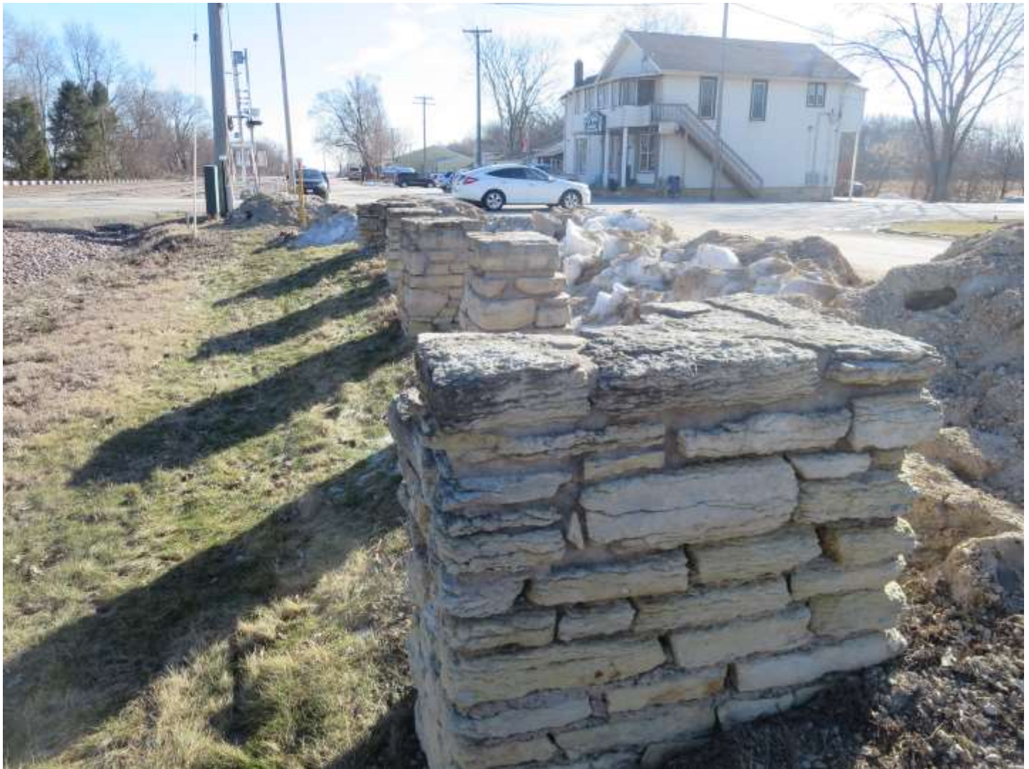
FIGURE 4: HISTORIC FOUNDATION PIERS AT THE ORIGINAL SITE.
