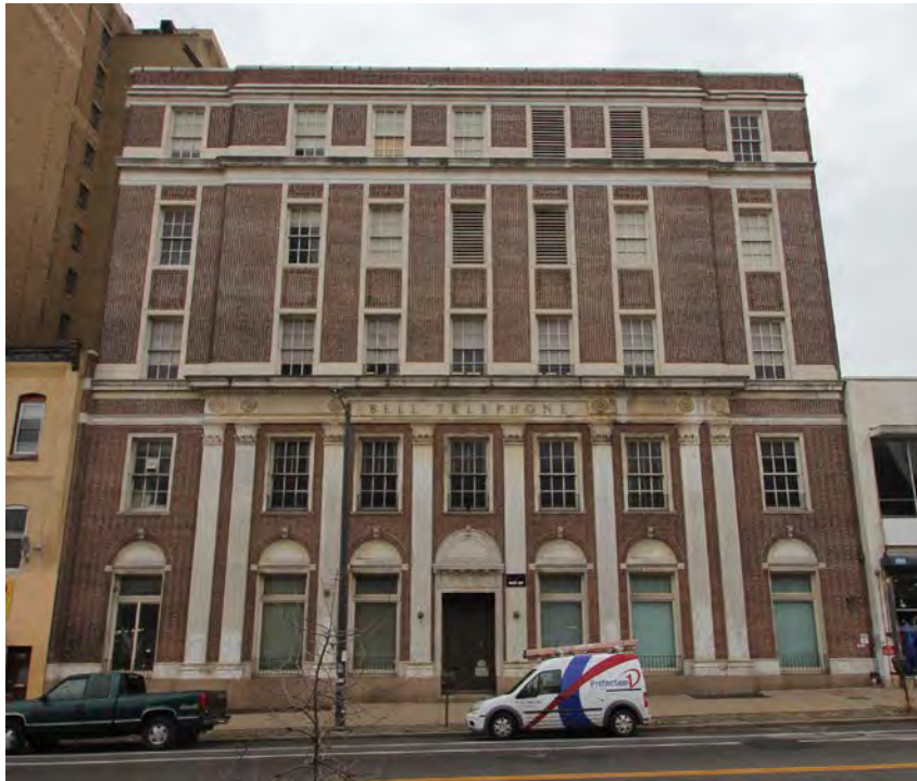
Figure 18 – Germantown Central Office, 2014.
