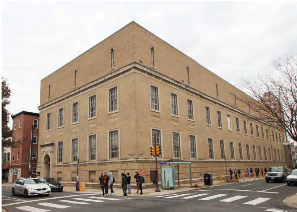
Figure 22 – Lombard Central Office, 2014.
