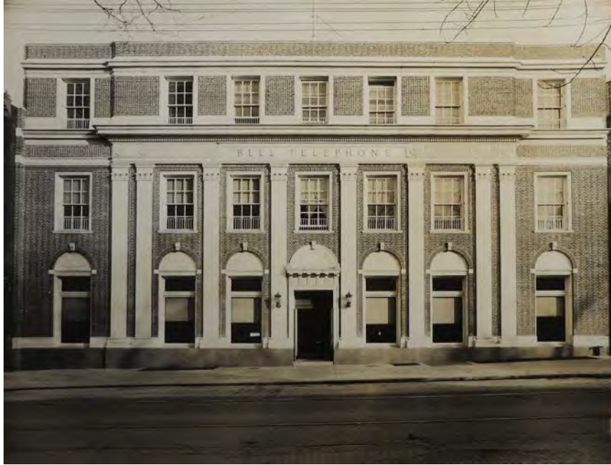
Figure 17 – Germantown Central Office, 26-34 W. Chelton Avenue, c. 1925. (Historical Society of Pennsylvania)
