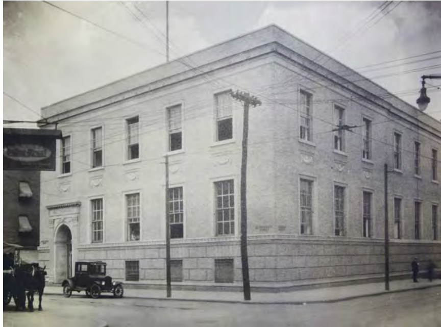
Figure 21 – Lombard Central Office, NE Corner of 17 th and Lombard Streets, c. 1925. (Historical Society of Pennsylvania)
