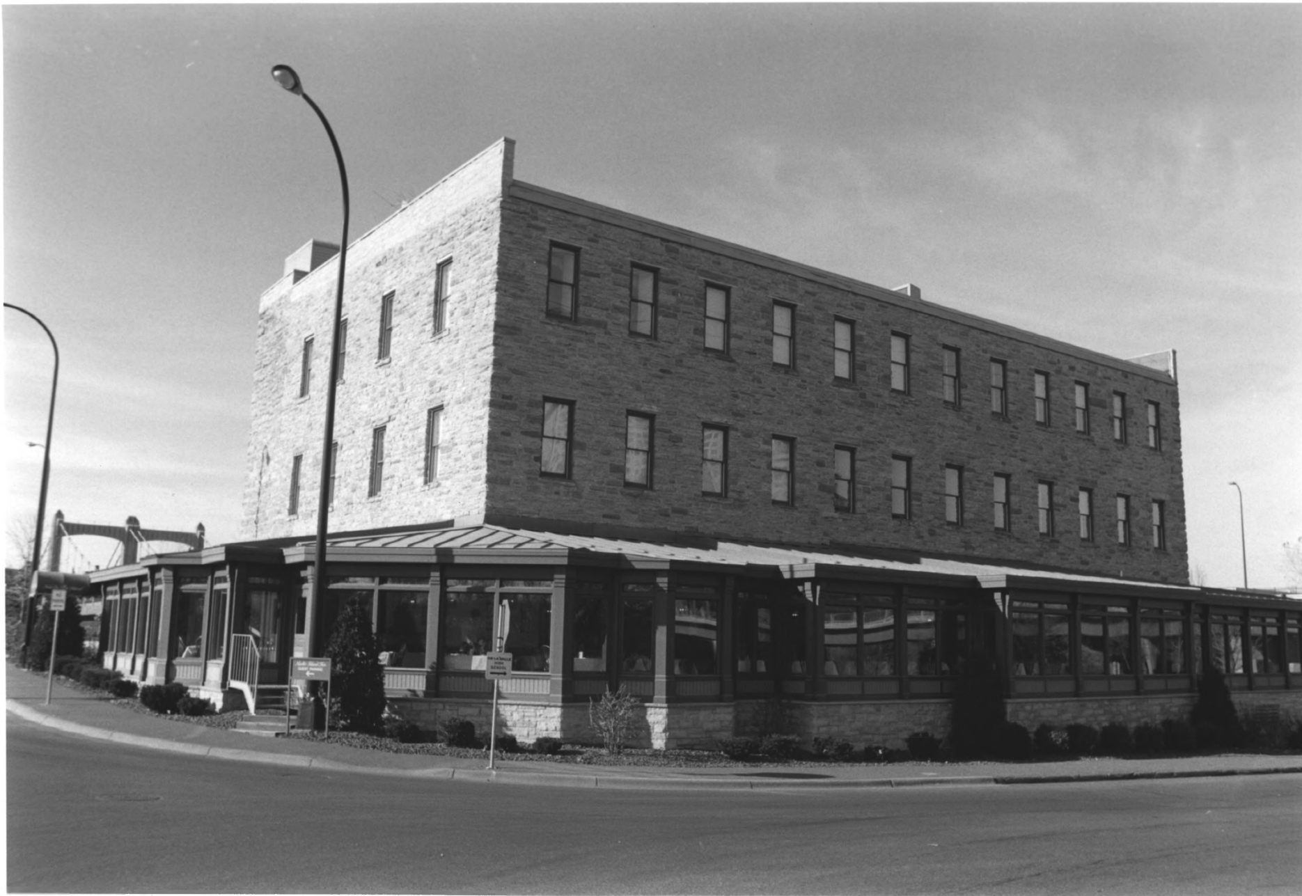
ISLAND SASH AND DOOR FACTORY ST ANTHONY FALLS HISTORIC DISTRICT MINNEAPOLIS, HENNEPIN CO., MN 010843 #4
