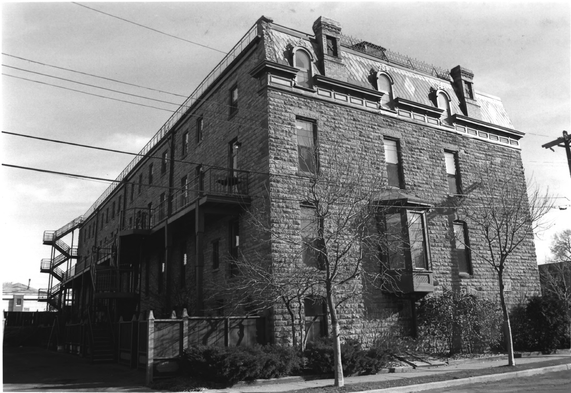
EASTMAN TOWN HOUSES ST. ANTHONY FALLS HISTORIC DISTRICT MINNEAPOLIS, HENNEPIN CO., MINNESOTA #010843-10
