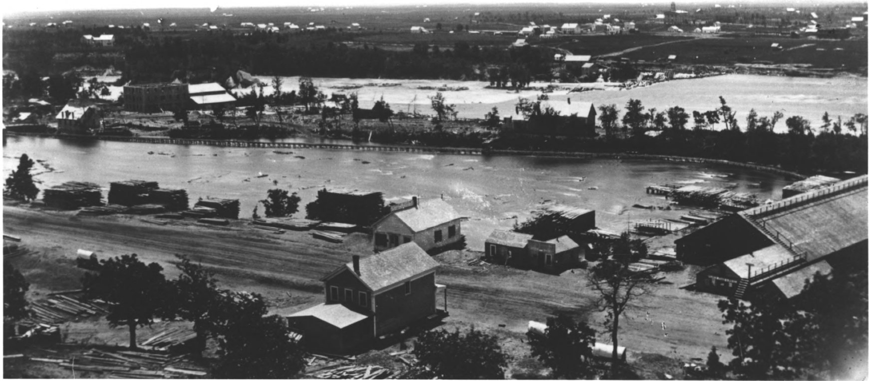
ST. ANTHONY FALLS WATERPOWER AREA ST. ANTHONY FALLS HISTORIC DISTRICT MINNEAPOLIS, HENNEPIN CO., MINNESOTA #4133
