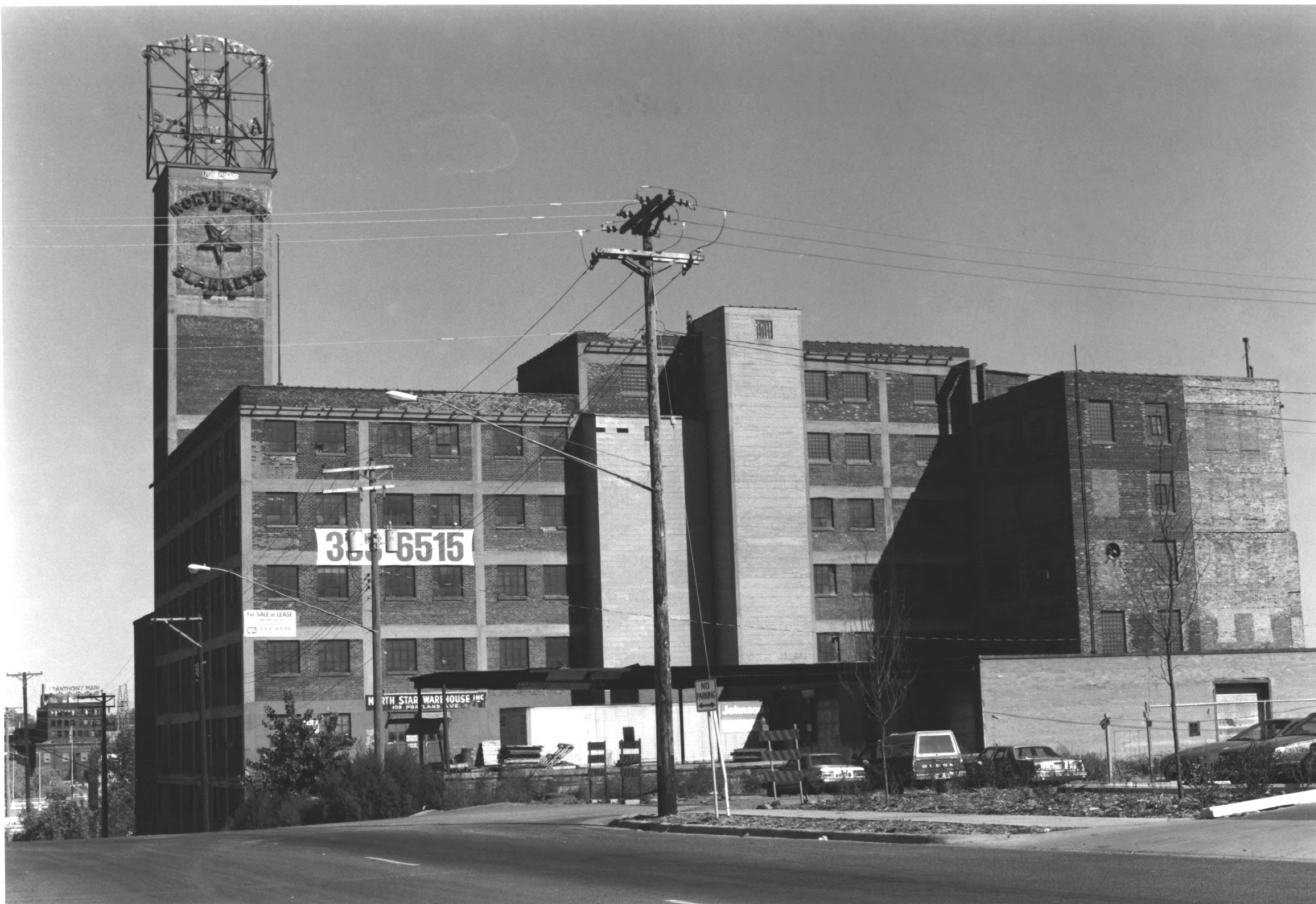
NORTH STAR WOOLEN MILL ST. ANTHONY FALLS HISTORIC DISTRICT MINNEAPOLIS, HENNEPIN CO., MN PHOTO: 010056-0A-1
