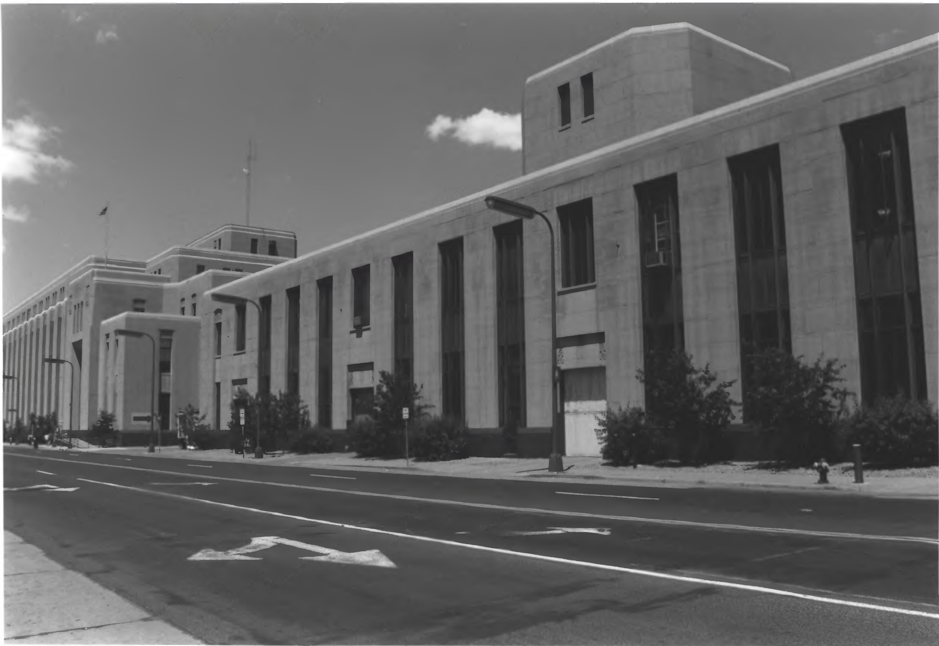
MINNEAPOLIS POST OFFICE, MAIN STATION ST. ANTHONY FALLS HISTORIC DISTRICT MINNEAPOLIS, HENNEPIN CO., MINNESOTA PHOTO: 010264-22
