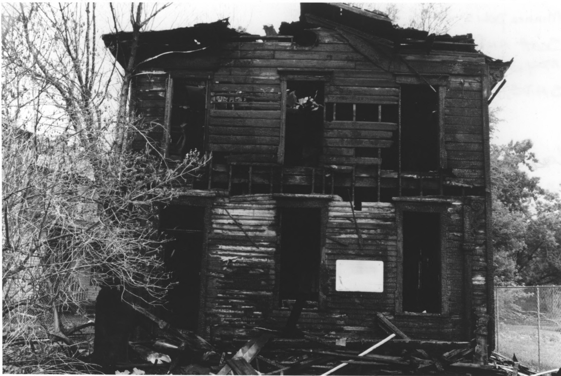
115 WEST ISLAND AVENUE NICOLLET ISLAND HISTORIC RESIDENTIAL AREA MINNEAPOLIS, HENNEPIN CO., MN NO PHOTO #
