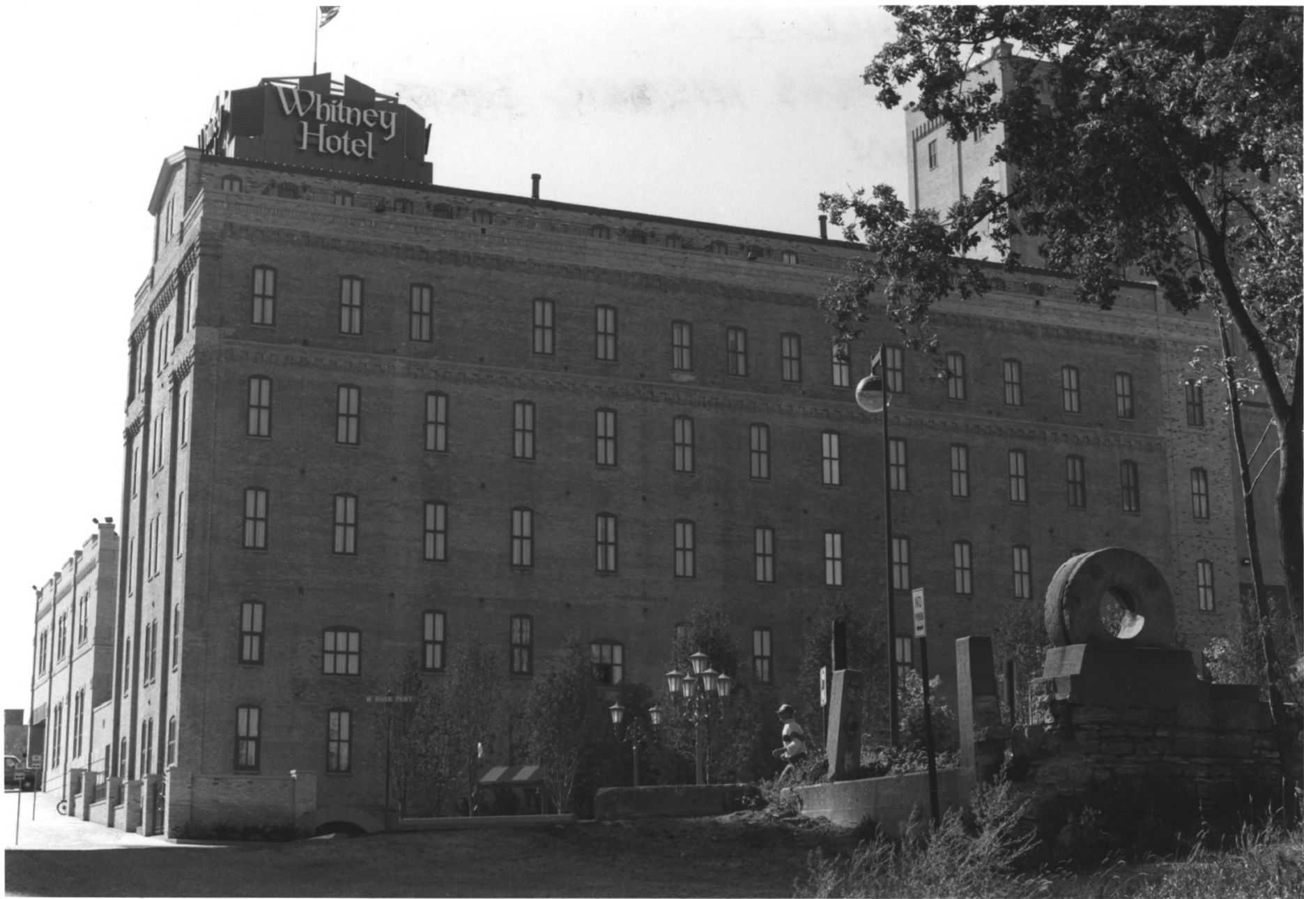
STANDARD MILL ST. ANTHONY FALLS HISTORIC DISTRICT MINNEAPOLIS, HENNEPIN CO., MN PHOTO: 010054-15A-16
