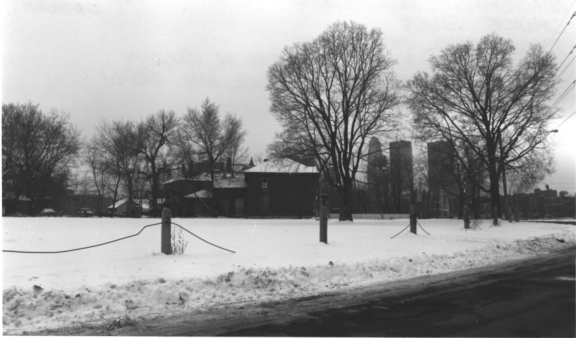
WEST ISLAND AVENUE - STREETSCAPE NICOLLET ISLAND HISTORIC RESIDENTIAL DISTRICT MINNEAPOLIS, HENNEPIN CO., MINNESOTA 010851 #17/17A
