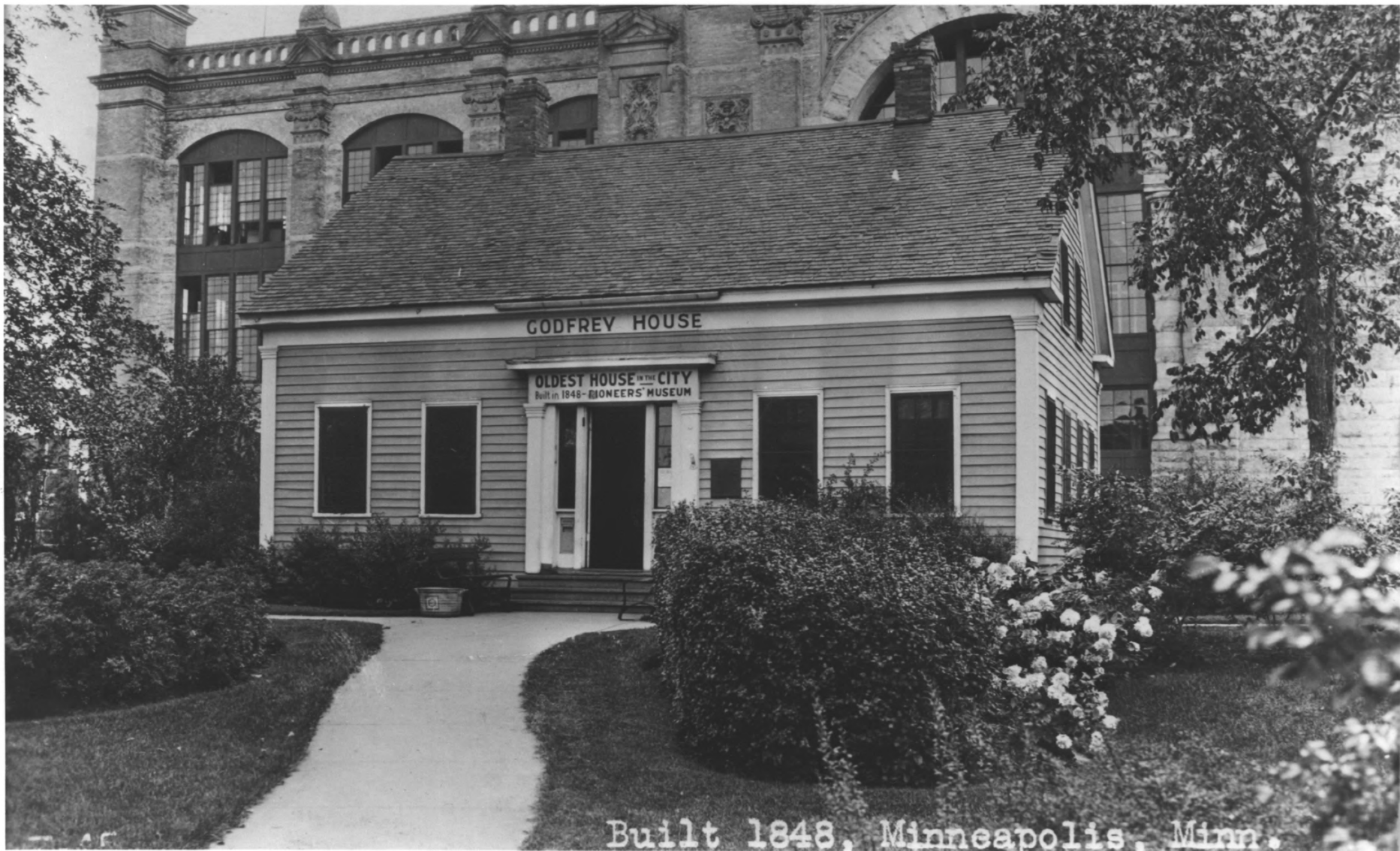
ARD GODFREY HOUSE ST. ANTHONY FALLS HISTORIC DISTRICT MINNEAPOLIS HENNEPIN CO., MINNESOTA # 7217
