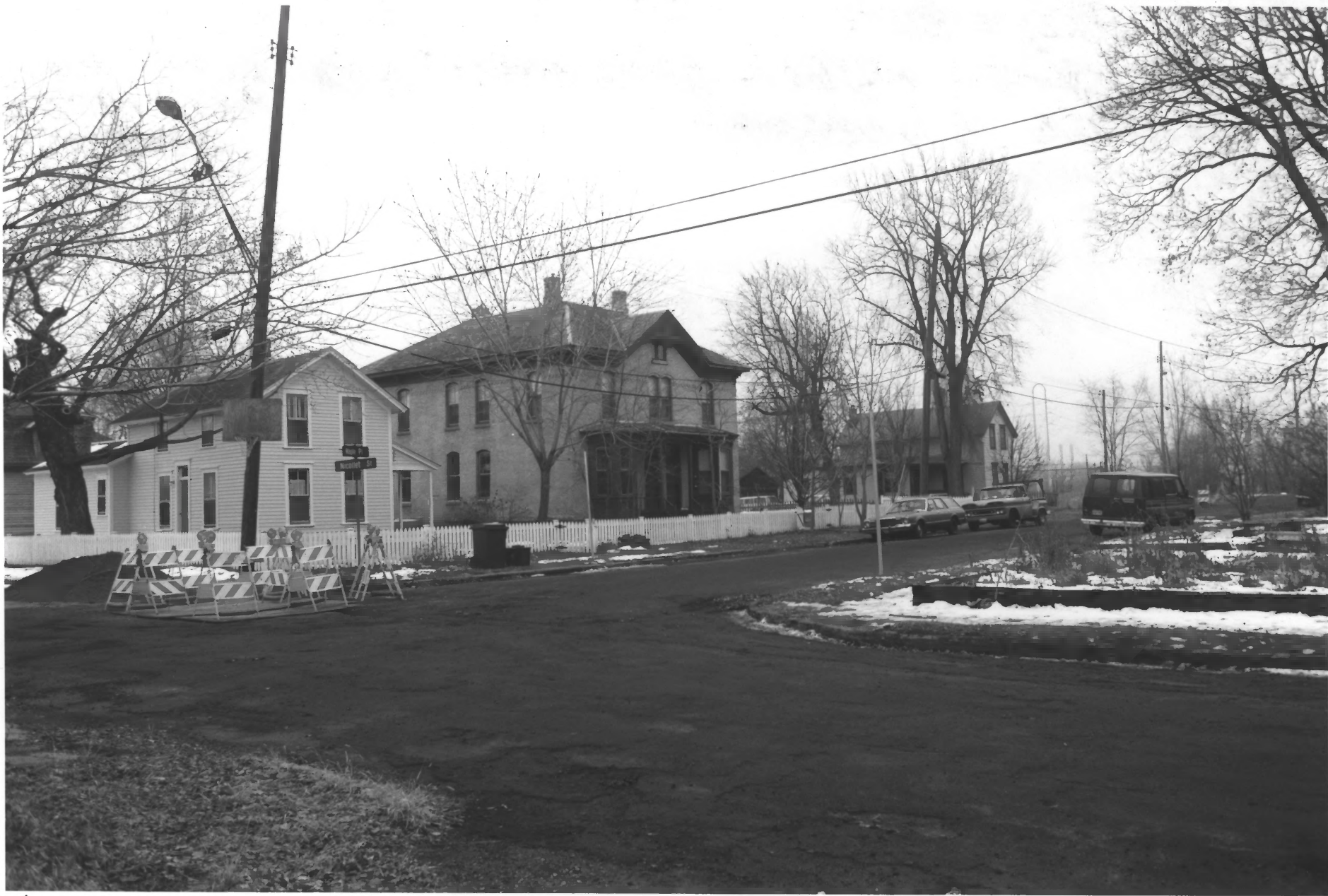
NICOLLET STREET- STREET SCAPE NICOLLET ISLAND HISTORIC RESIDENTIAL DISTRICT MINNEAPOLIS, HENNEPIN CO., MINNESOTA 010856 #23A
