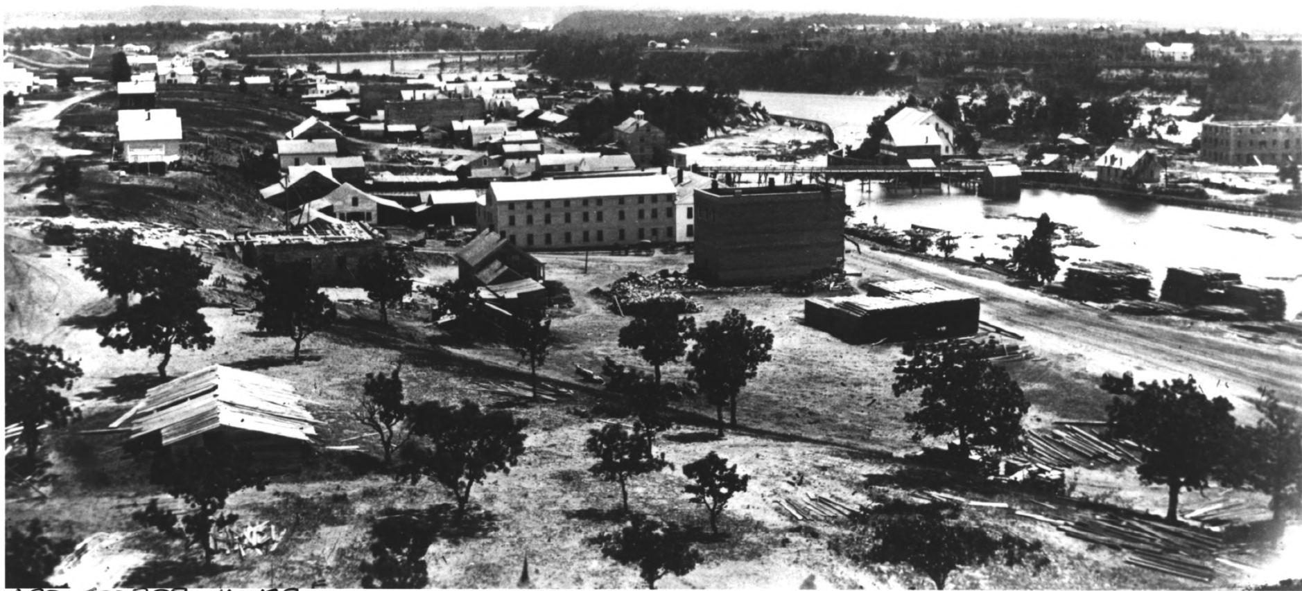
ARD GODFREY HOUSE ST. ANTHONY FALLS HISTORIC DISTRICT MINNEAPOLIS, HENNEPIN CO., MINNESOTA # 7422
