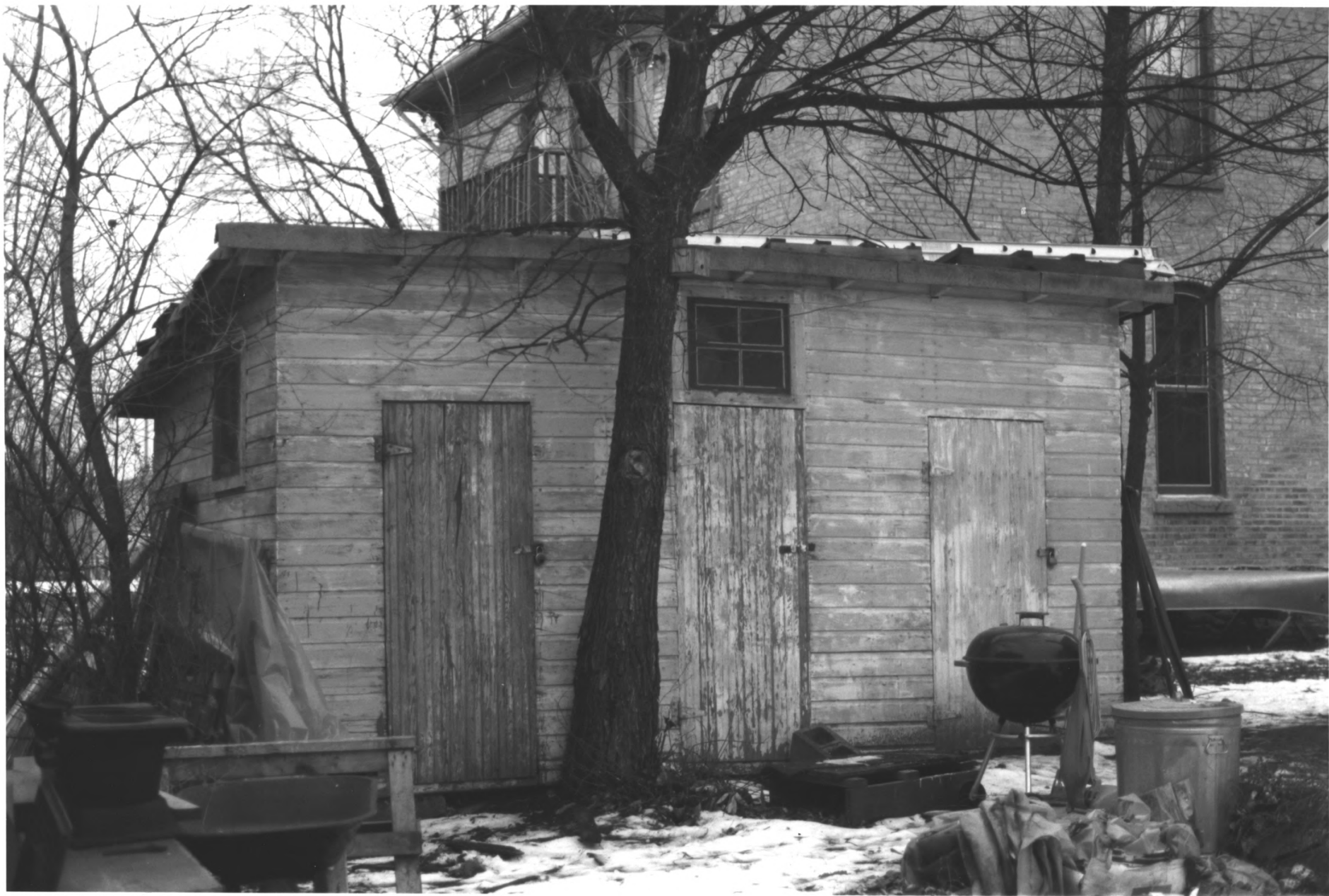
163 NICOLLET STREET- SHED NICOLLET ISLAND HISTORIC RESIDENTIAL DISTRICT MINNEAPOLIS, HENNEPIN CO, MINNESOTA 010 858 #6/6A NON-CONTRIBUTING
