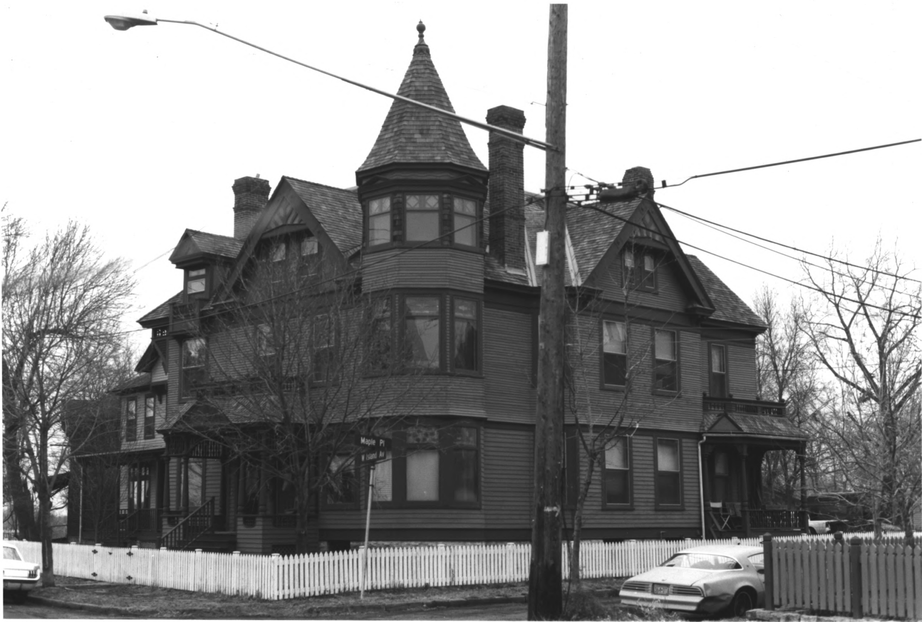
107-107 WEST ISLAND AVENUE NICOLLET ISLAND HISTORIC RESIDENTIAL DISTRICT MINNEAPOLIS, HENNEPIN CO.; MINNESOTA 010859 #18A/19
