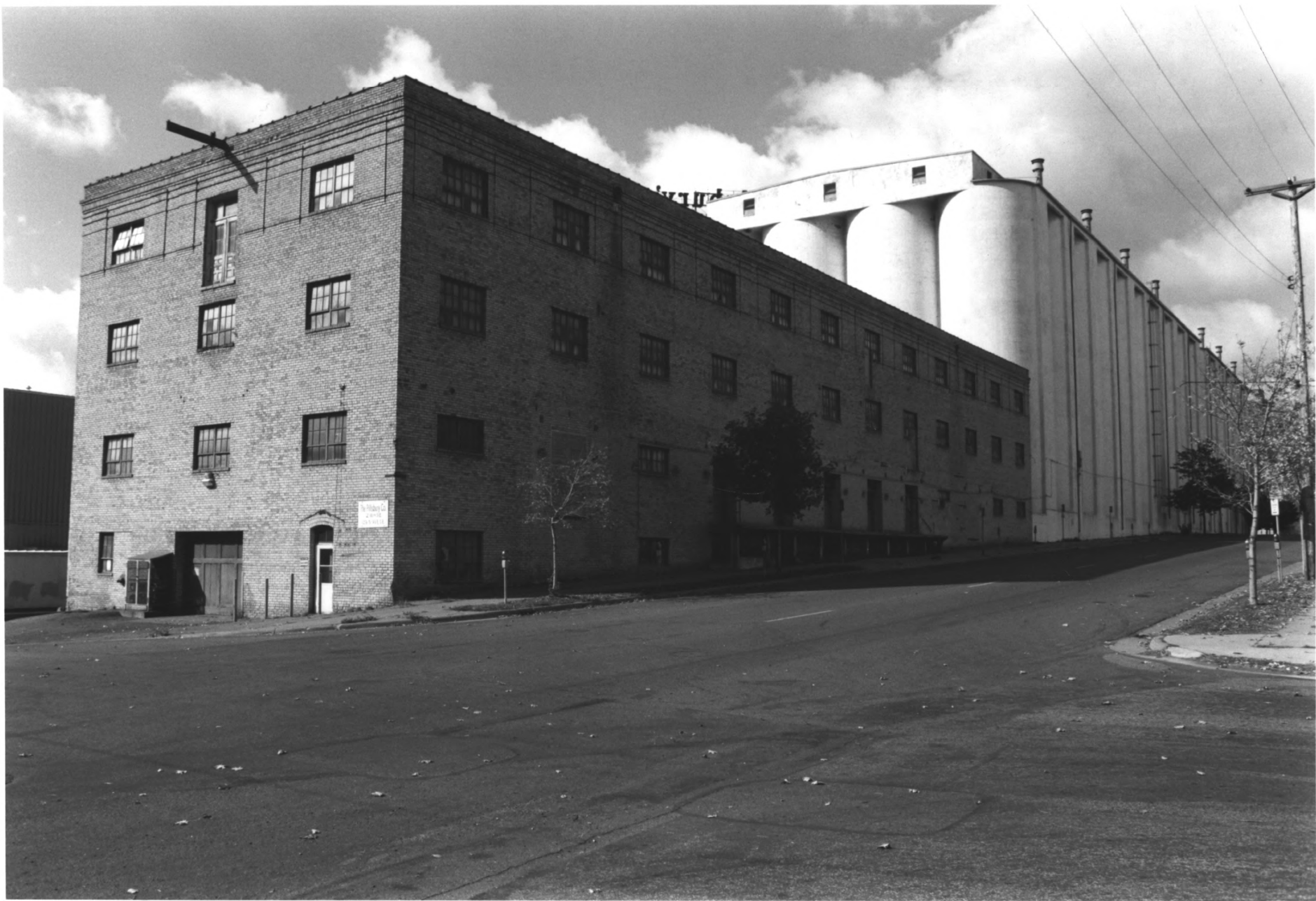
PILLSBURY WAREHOUSE #2 & CONCRETE ELEVATORS ST. ANTHONY FALLS HISTORIC DISTRICT MINNEAPOLIS, HENNEPIN CO., MN PHOTO: 010052 1A-2
