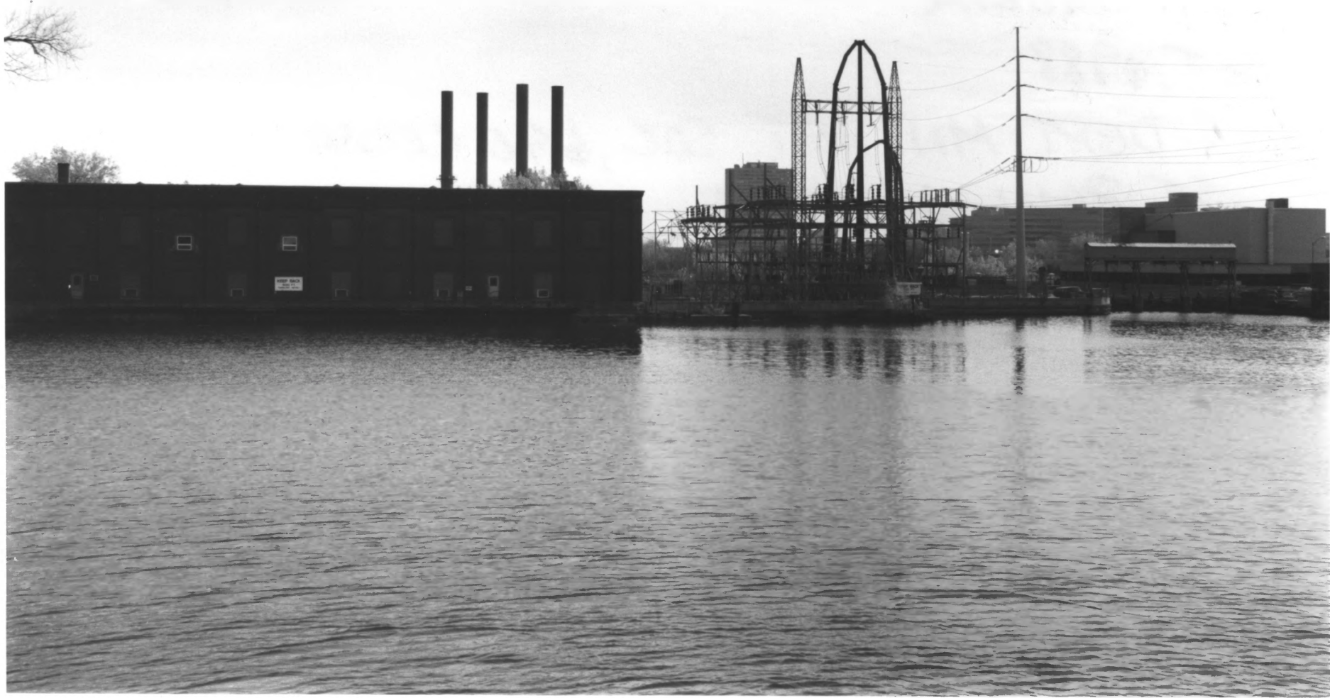
MAIN STREET HYDROELECTRIC STATION ST. ANTHONY FALLS HISTORIC DISTRICT MINNEAPOLIS, HENNEPIN CO., MN PHOTO: 010073 11-11A
