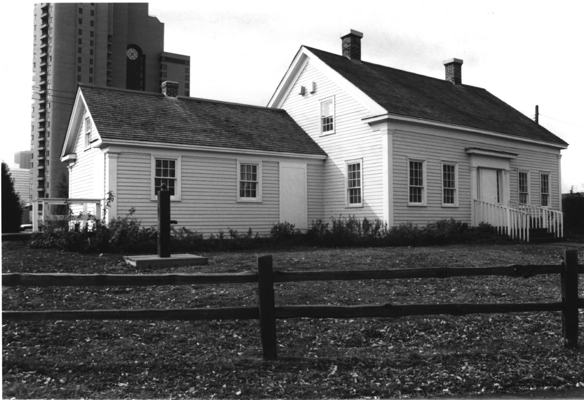
ARD GODFREY HOUSE ST. ANTHONY FALLS HISTORIC DISTRICT MINNEAPOLIS, HENNEPIN CO., MN PHOTO: 010073-20
