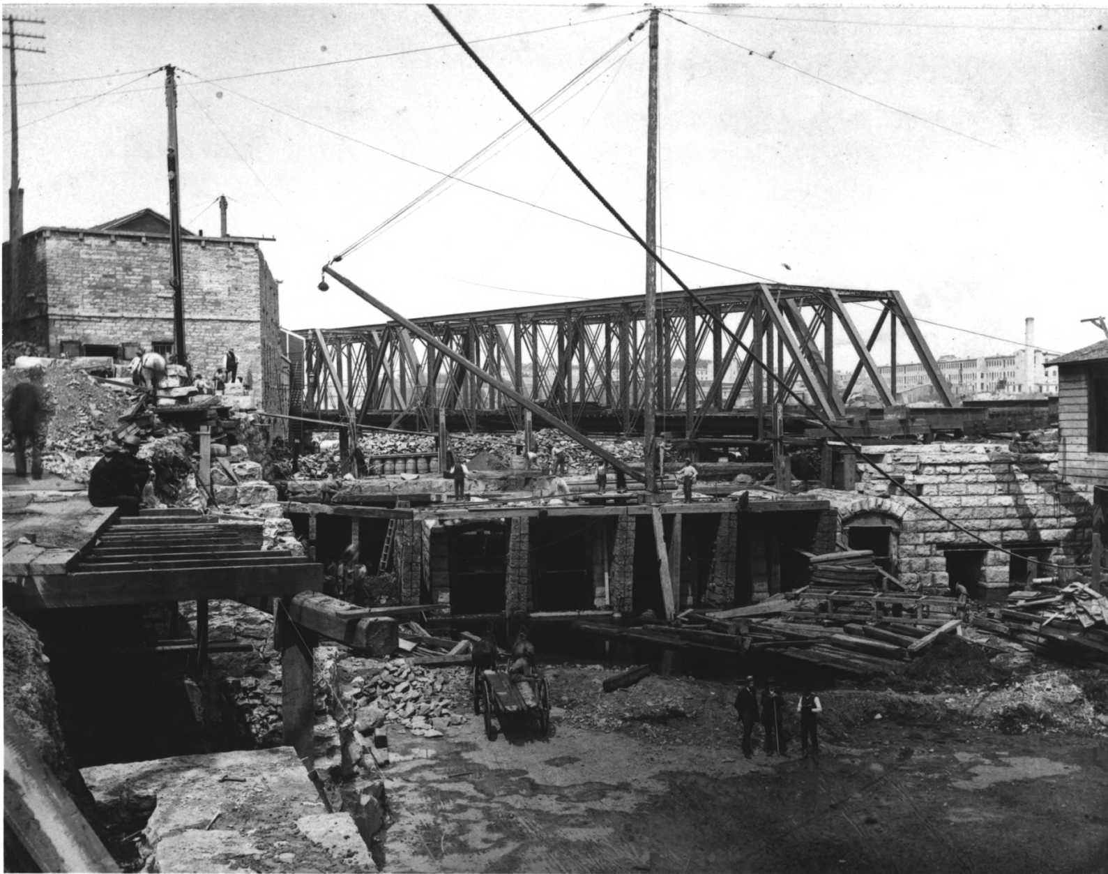
ST. ANTHONY FALLS WATERPOWER AREA ST. ANTHONY FALLS HISTORIC DISTRICT MINNEAPOLIS, HENNEPIN CO., MINNESOTA #34476
