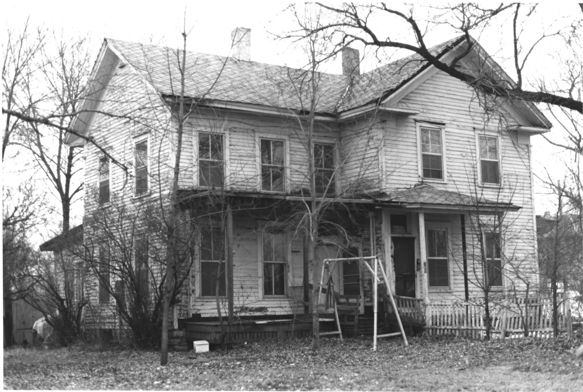
185-186 EAST ISLAND AVENUE NICOLLET ISLAND HISTORIC RESIDENTIAL DISTRICT MINNEAPOLIS, HENNEPIN CO., MINNESOTA 010860 #19A/20
